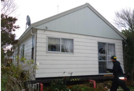
Figure 6: Wairoa St. House, base anchor beam visible
