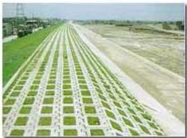
Figure 5. Dike construction employing ecology methods
