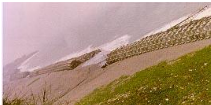
Figure 7. Coastal protection along Ginshan beach in Taipei County
