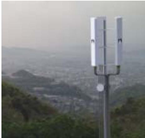
Fig 1-30 A cluster of 120° panel array antennas
