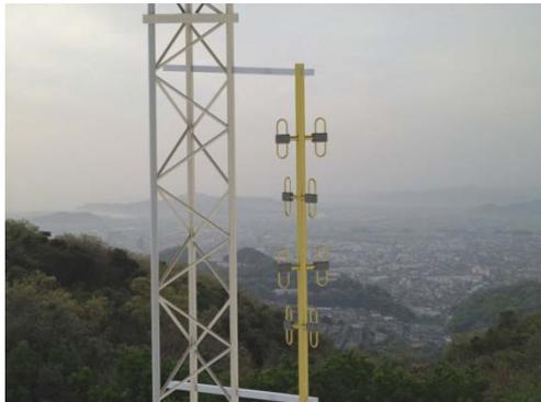
Fig 1-32 Corporate fed folded dipole array (RFI BA80-67) [2]
