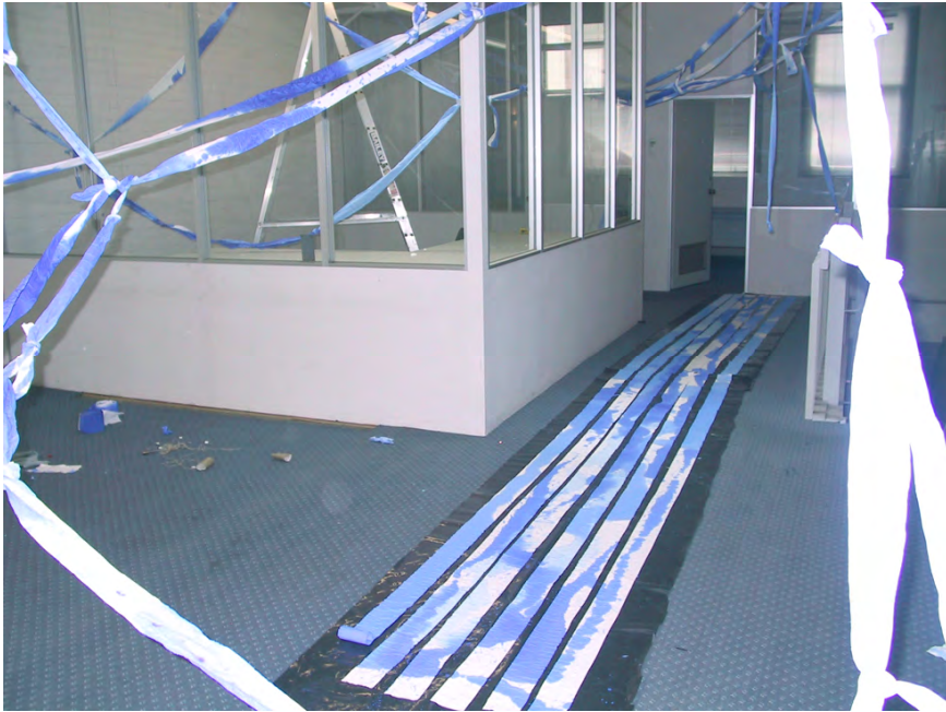
Figure 2.13. Greg Creek, installation structures (studiowork detail)
