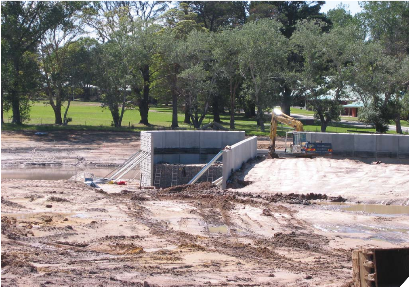
Construction photo. Breaking the dominance of the Plateau with the fissures
