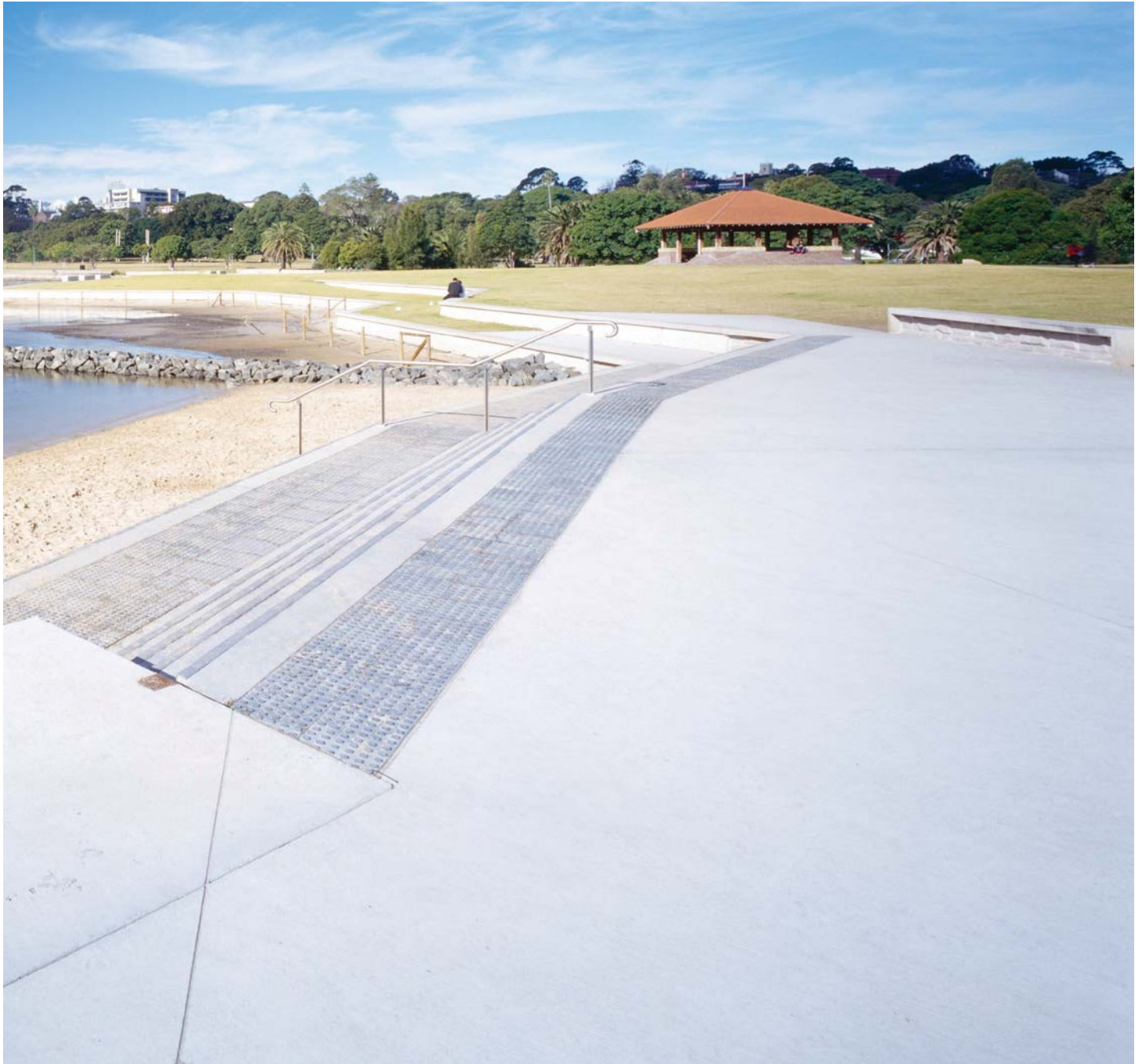
Looking east. The rock embankment in the middle ground becomes an island at high tide and separates the new beach from the new mangrove and salt marsh. This section of the project dramatically increases marine habitat and provides a safe resting place for birds at high tide.
