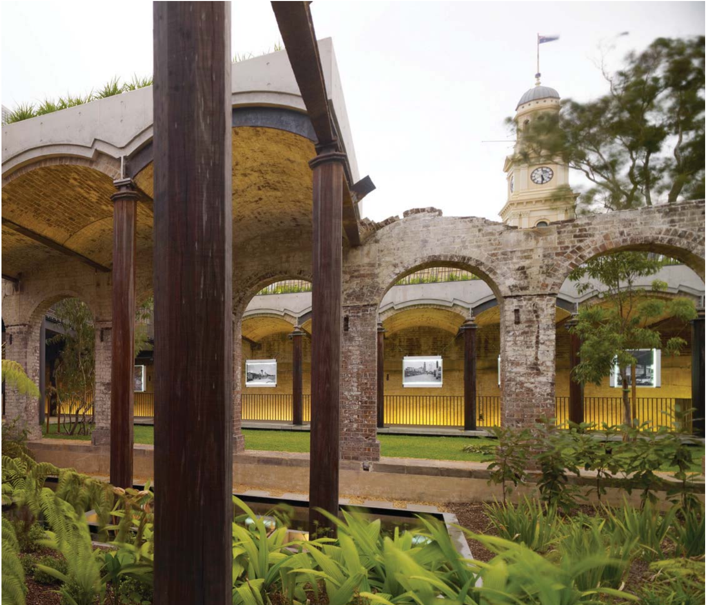
A view from within the western chamber showing the garden plantings and retained roof fragment
