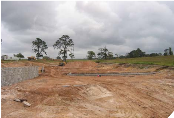
Construction photos of Water Gardens.
