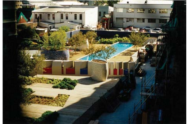
Construction site view from the south towards the pool. 1999
