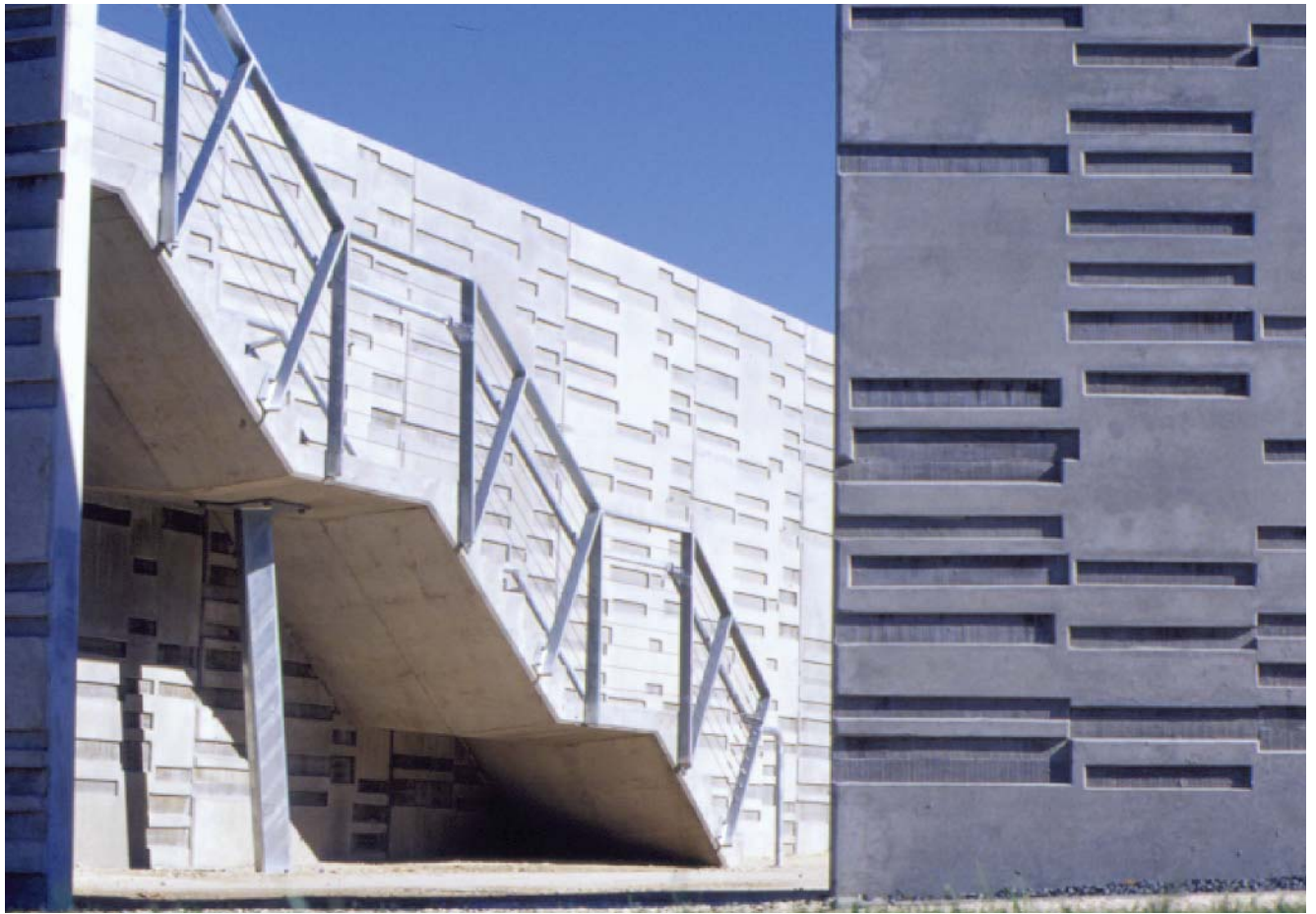
Stair against the concrete Plateau wall and a grounded stair leading to the Bottle Tree Garden (bottom right)
