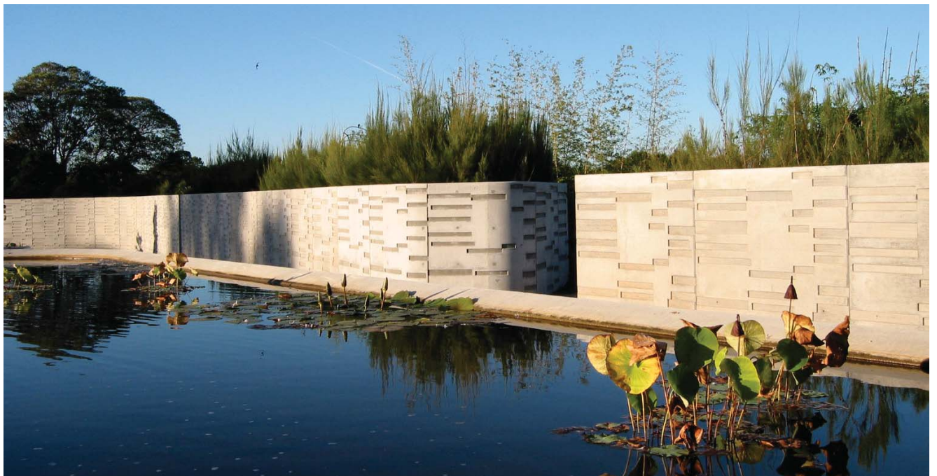
Concrete wall along the Water Gardens between the existing dam and the Plateau.
