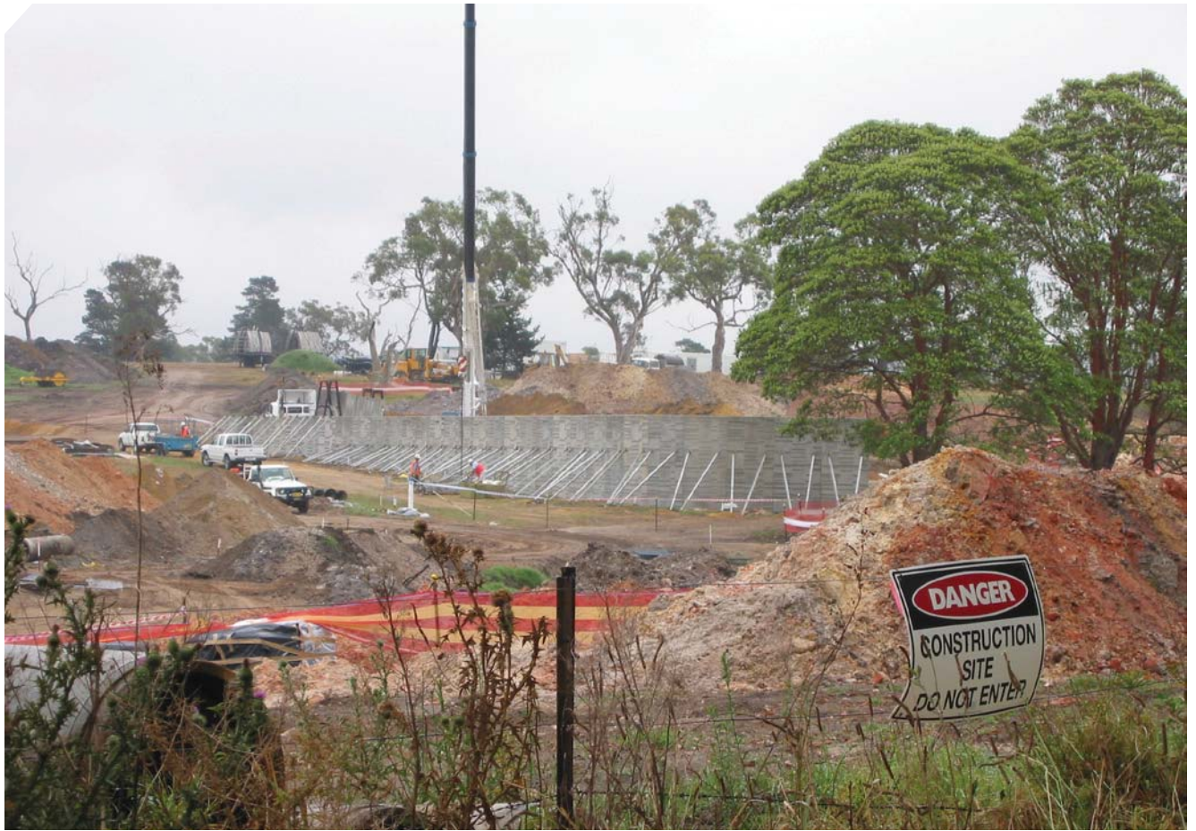
Construction photo. Built diversion around the easement
