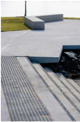
Views of the platforms, stairs and reconfigured basalt used to scale the beach and new mangrove
