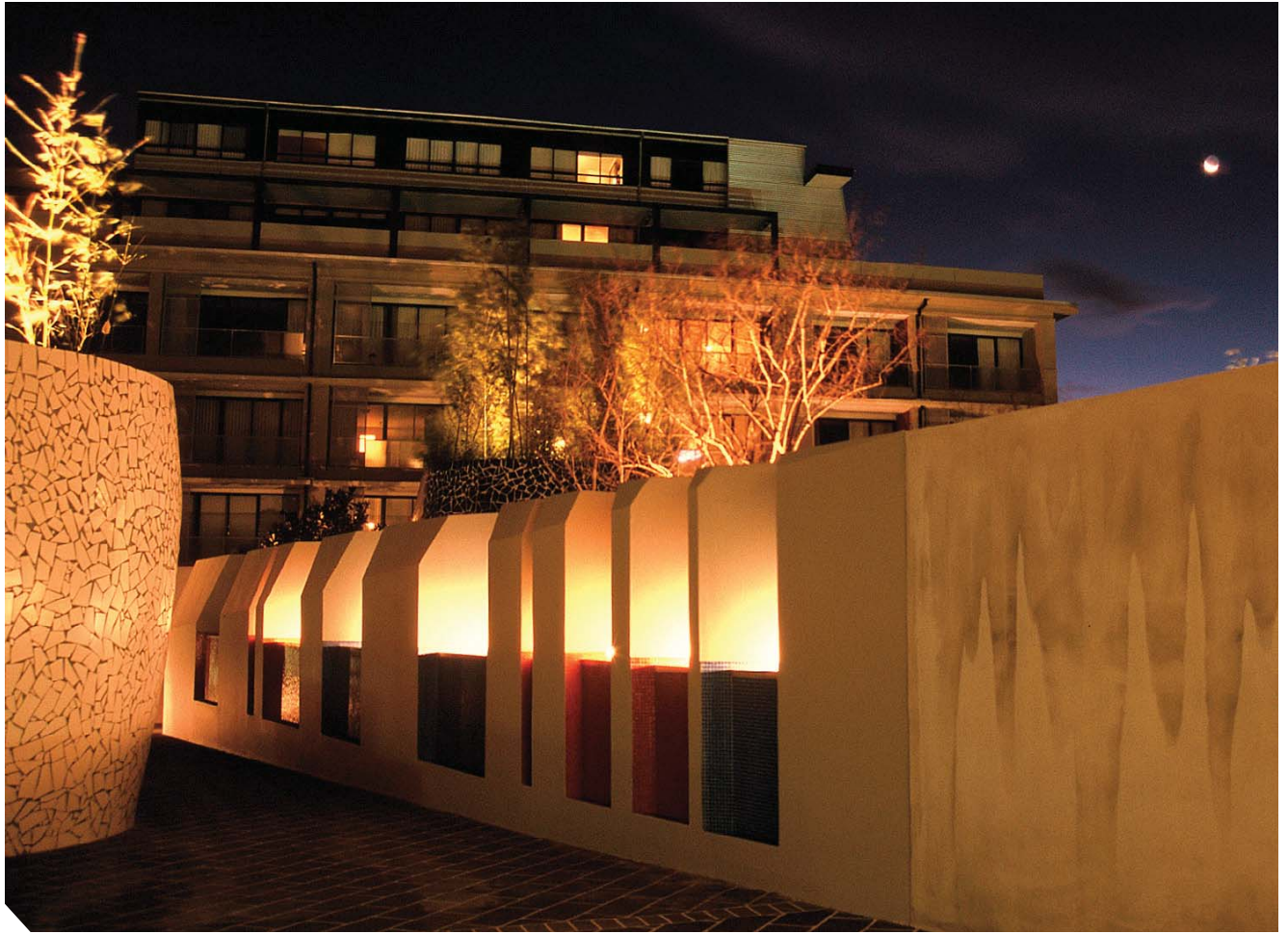
Night time view of the Wedge Wall Photo Allen Jack and Cottier
