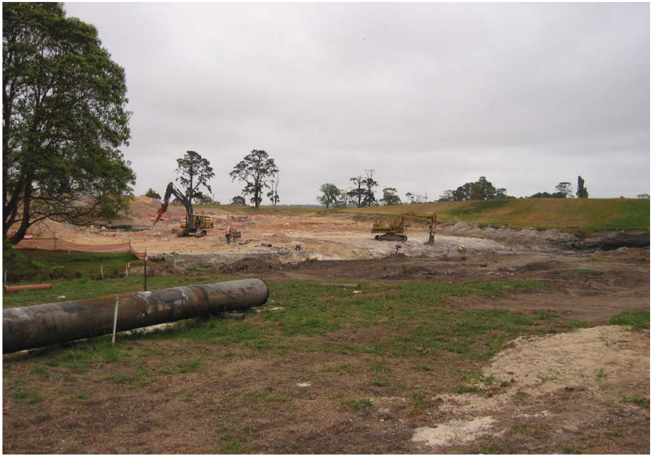
Construction photos. Earthworks against existing dam wall. Establishing scale
