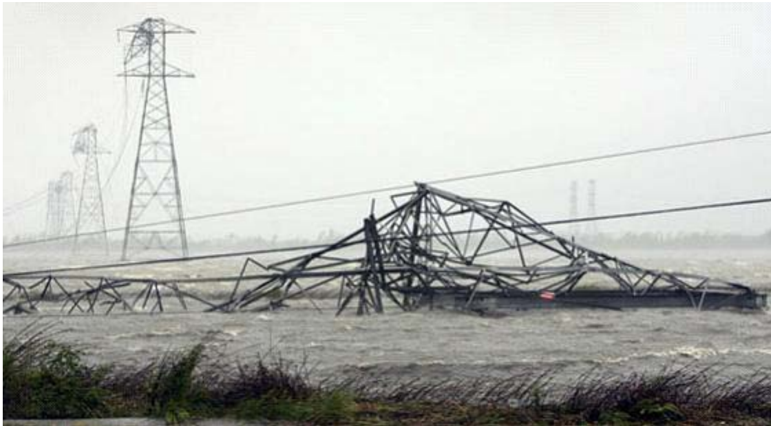
Figure 1.2 A Collapsed Power Pylon due to 1998 Storm
