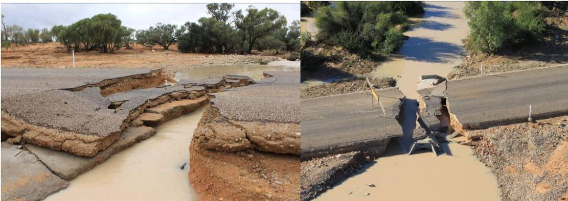
**Figure 2.** Flood damaged roads in Central West Region, Queensland, Australia in early 2011 (DTMR, 2011)
