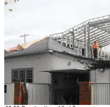
02.33 Construction of first floor
