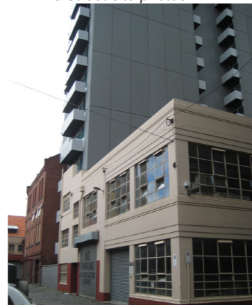
01.43 17 Wills Street site photos
