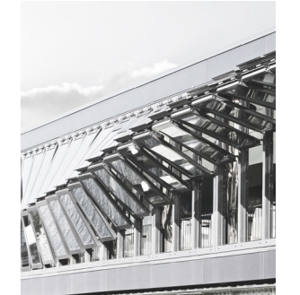
02.15 Image by Rob Hoekstra railway bridge on the Westerdokseiland in Amsterdam by de Architekten Cie.
