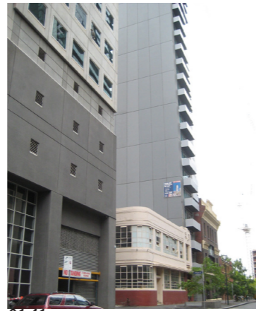
01.41 17 Wills Street site photos
