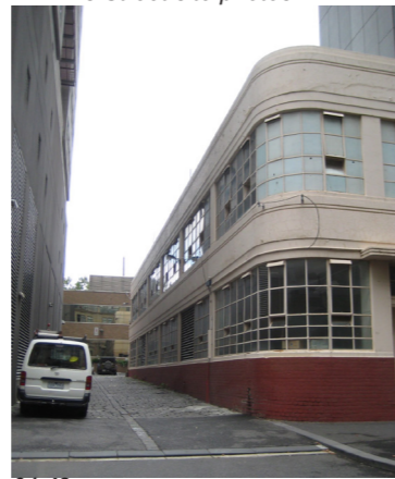
01.42 17 Wills Street site photos
