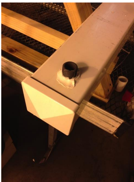
FIGURE 20: LEAK FIXED WITH SILICONE
