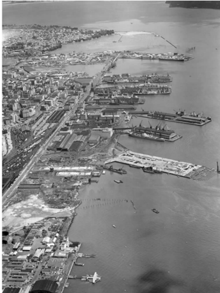
Right: circa 1900 showing Auckland's waterfront aligned along Quay Street comprising a series of landfill and finger wharfs. The project site is in the top right hand corner of the photograph.
