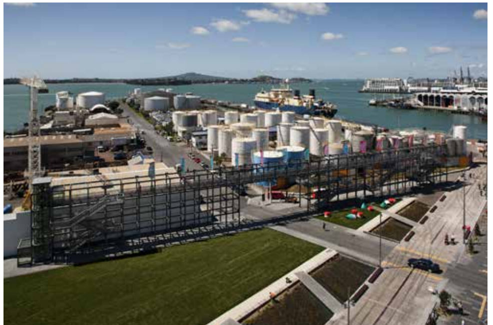
Right: Silo Park comprising the central lawn, Silos, Wetlands, Gantry's and promenade. The park is now a popular concert and film venue.
