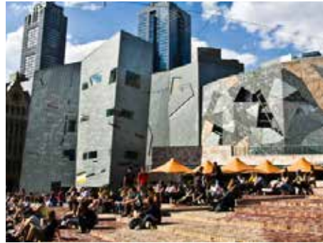
Left: Occupying the terraces at Federation Square. Opposite Right: The Plaza, Federation Square.
