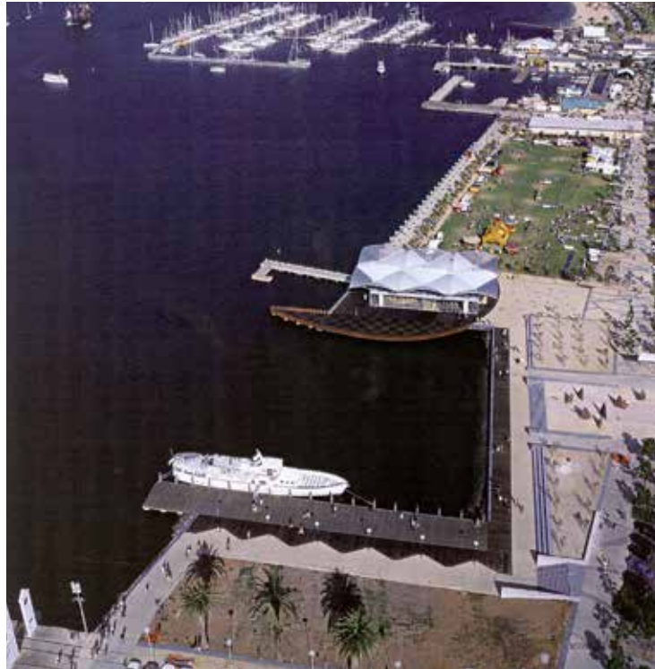
Right: Completed Geelong Waterfront redevelopment comprising a linear promenade, event spaces and nodal points, such as small harbours, that were located of the intersection extension of Hoddles grid.
