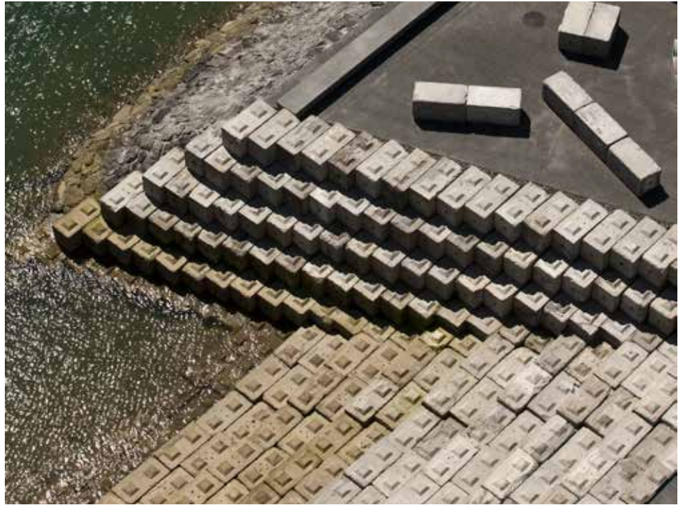
Right: Material Presence in Auckland is captured via the use of precast concrete blocks that were on the site, as a new water stair to the harbour.
