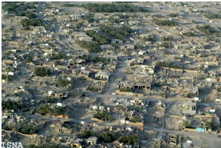
Figure 1.2: The catastrophic Bam earthquake (Source: Iran Students News Agency, (2003))
