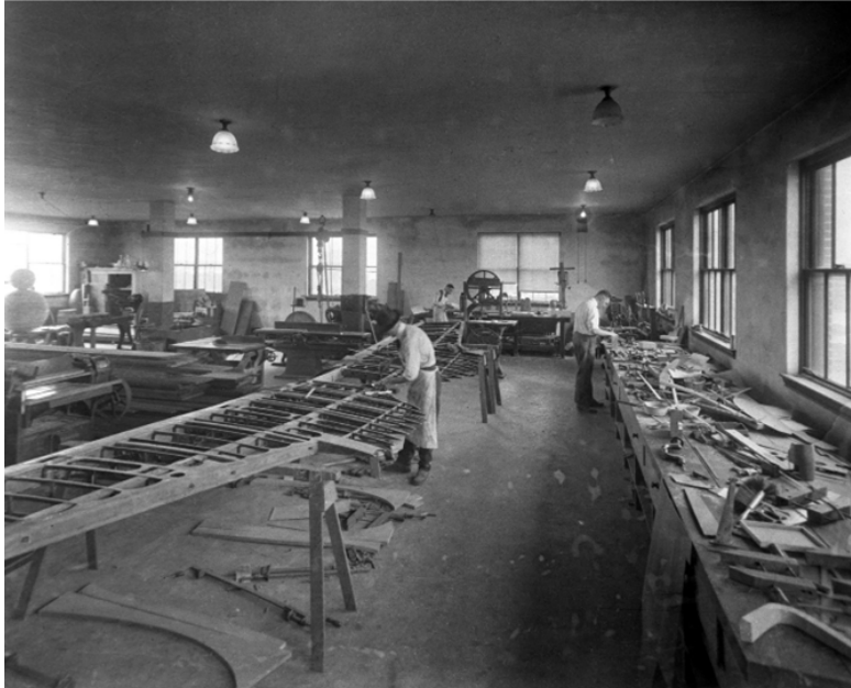
Figure 3.5-1: Workmen in the Patternmakers' Shop manufacture a wing skeleton for a Thomas-Morse MB-3 Airplane for pressure distribution studies in flight, June 1922. 5
