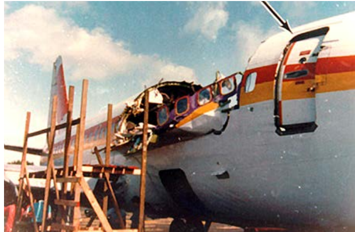
Figure 13.3-1: The photograph from the NTSB Report (NTSB number: AAR-89-03) shows the explosive decompression of the fuselage.
