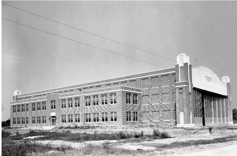
Figure 3.5-3: Completed Structures and Materials Research Facility Building 1148; 1940.
