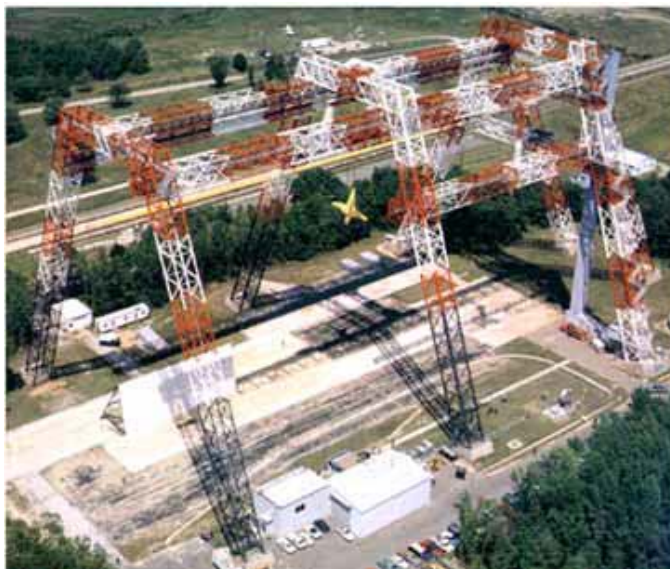
Figure 2.2-2: Photograph of the IDRF Located at NASA Langley Research Center.
