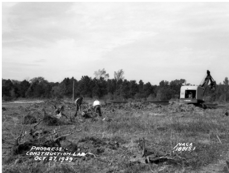
Figure 3.5-2: Clearing for Structures and Materials Research Facility Building 1148; October 27, 1939.
