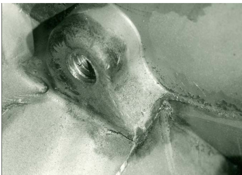
Figure 2.10-6: Region of a Fastener Boss Exhibiting Cracking.
