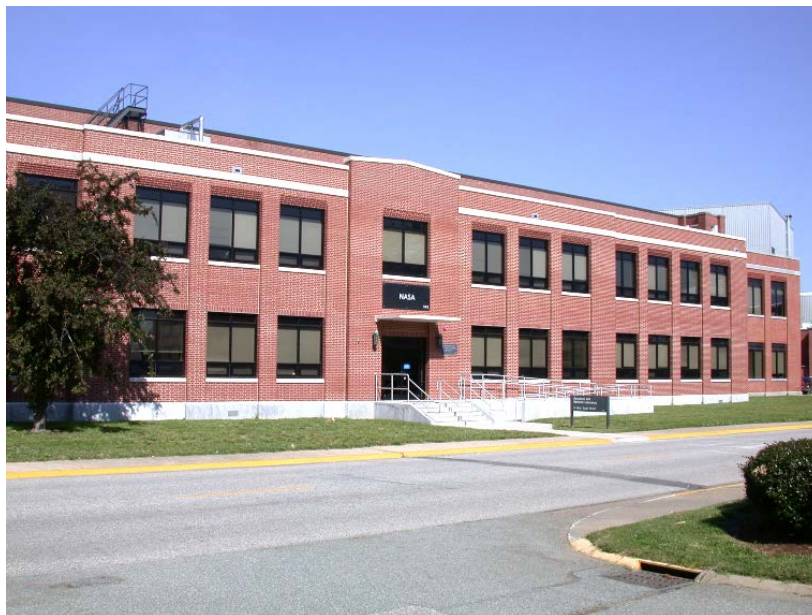
Figure 3.5-5: Exterior View of the Structures and Materials Research Facility Building 1148; 2007.
