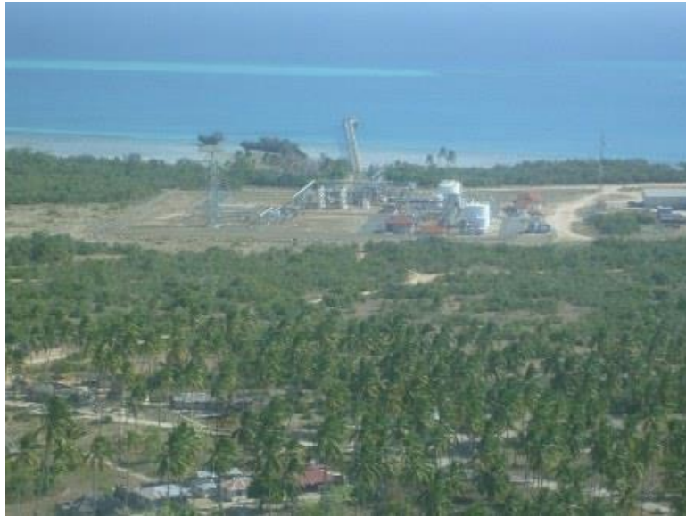
Figure 5.10: Aerial view of gas plant showing part of the island zoned off
