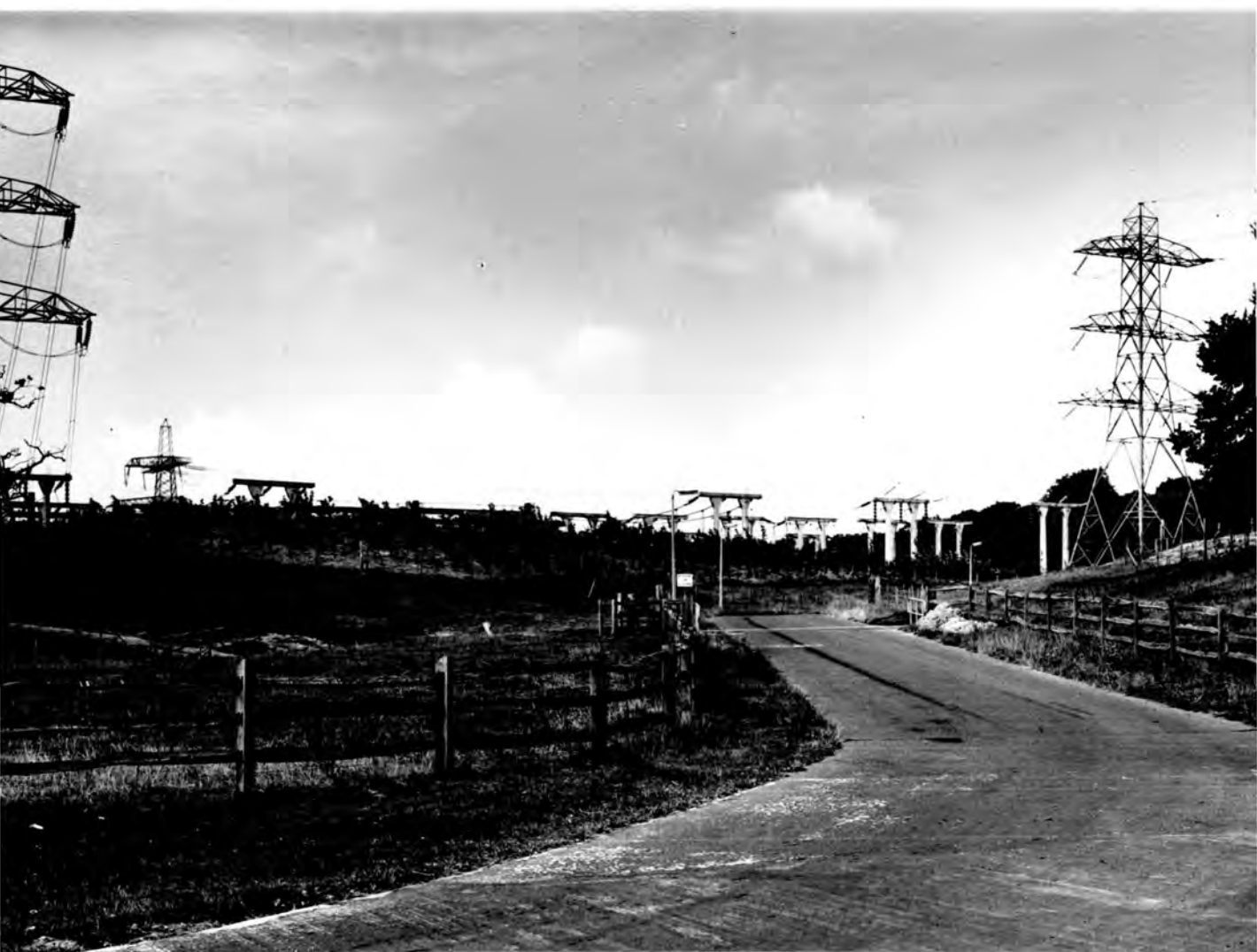
Photograph 80. View of Ninfield substation in East Sussex from the access road. See also Maps 36 and 37 and Photograph 40. The photograph illustrates that ground modelling on a considerable scale has been carried out in order to make the substation 'fit into' the existing land form and to screen it from the adjoining highway. The ground modelling and tree planting is said to be 0.35% of the total contract cost. A considerable amount of earth moving was necessary to form a level for the substation, the surplus material being used for the ground modelling. The landscaping in this case represents a financial saving to the Board by using to advantage the surplus material rather than having it carted away.
