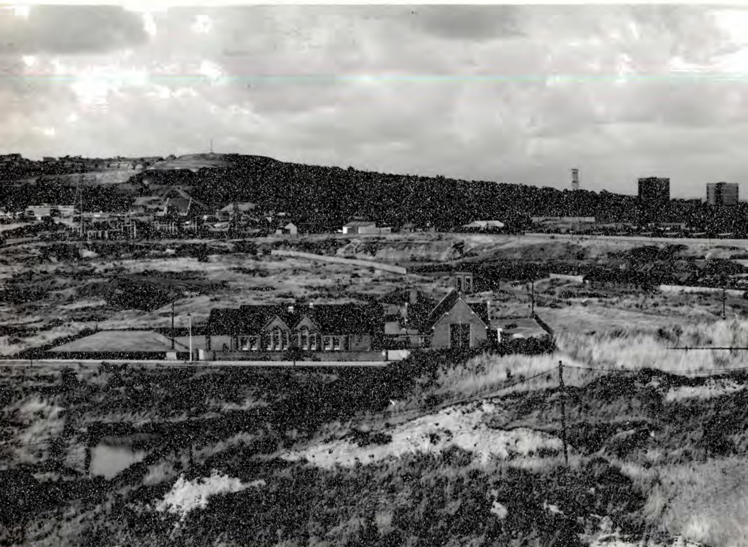
Photograph 44. View from 'Blue Billy' westwards across the proposed Oldbury substation site, showing general character of the area of industrial dereliction.
