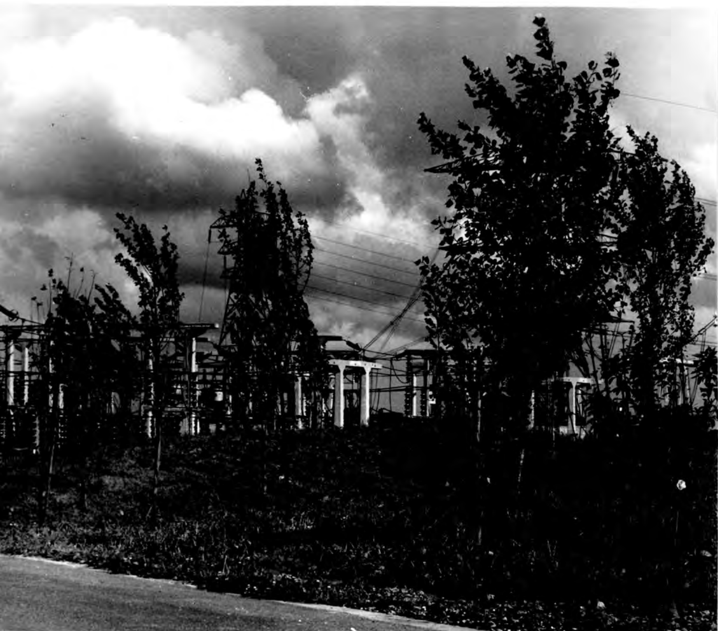
Photograph 75. View of Coventry substation from the access road. Modest ground shaping and a few recently planted trees have the effect of focusing attention to the foreground and 'smudging out' the substation behind.
