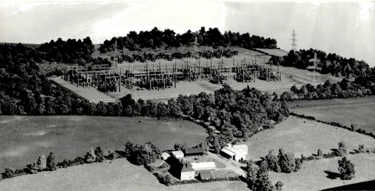
Photograph 70 S.W. view of model of proposed substation at Botany Bay. A combination of careful siting retaining the existing woodlands, with new planting would provide effective screening for this site.
