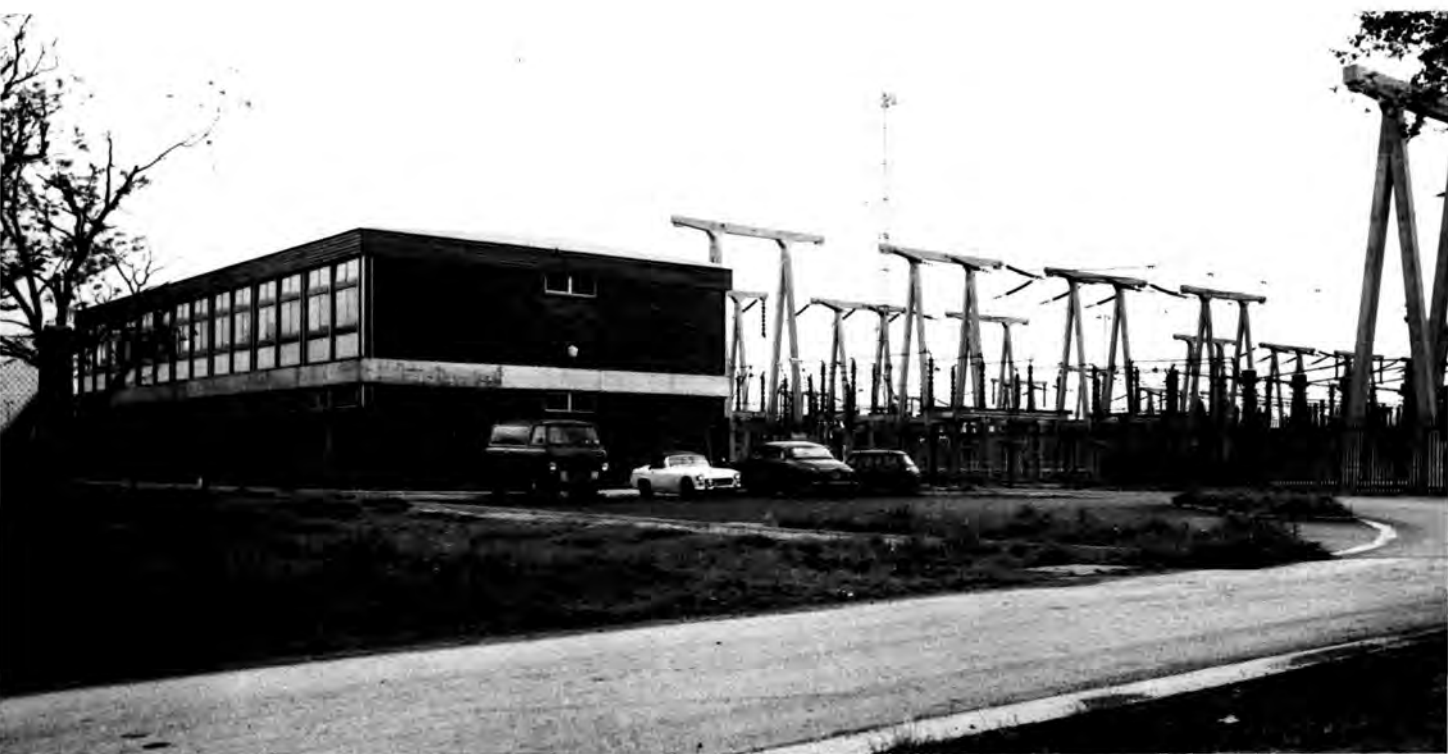
Photograph 51. Control building at South Manchester substation. Nearly every primary grid substation has a control building similar to the one shown in this photograph, usually two storey, but occasionally single storey. It is manned continuously for the operation of the transformer and switches, as well as providing for the security and supervision of the substation. The main room is the control room which occupies most of the first floor. The ground floor provides accommodation for banks of relay panels, and the electronic apparatus required for telecommunication with national control in London, and a local area control in Manchester.
