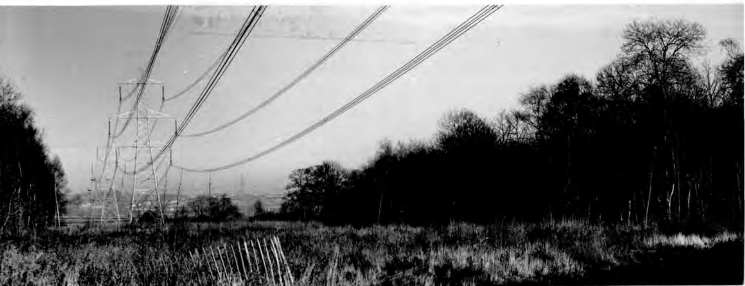
Photograph 20. The last span of a 400 kV line into Cowley substation near Oxford. This clear felling has opened up a view into the substation, behind the photographer, from a road in the middle distance. This could possibly have been avoided if a few trees had been retained near the tower. The trees at the edge of the swathe, being formerly in the heart of the wood, and thus tall and slender, are very liable to be blown over in a high wind. See next photograph for view in opposite direction.
