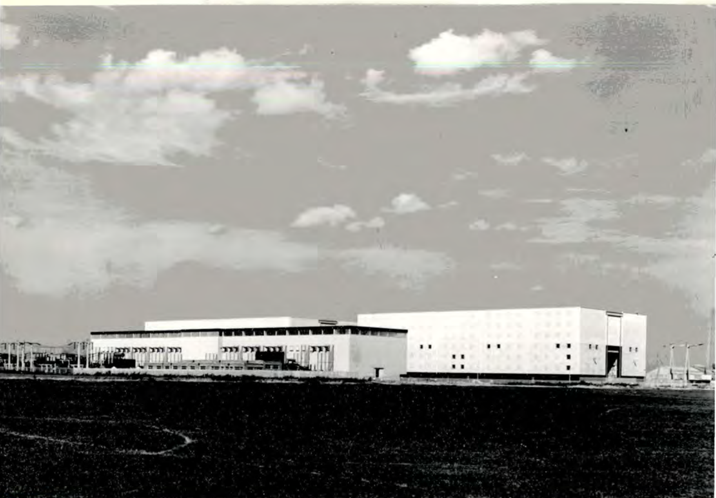
Photograph 47 showing 132 kV switchhouse in foreground and a 275 kV switchhouse behind at Willesden. The Board justifies the cost of these buildings on the ground that this was the only way to get all the electrical equipment required on to this restricted site.
