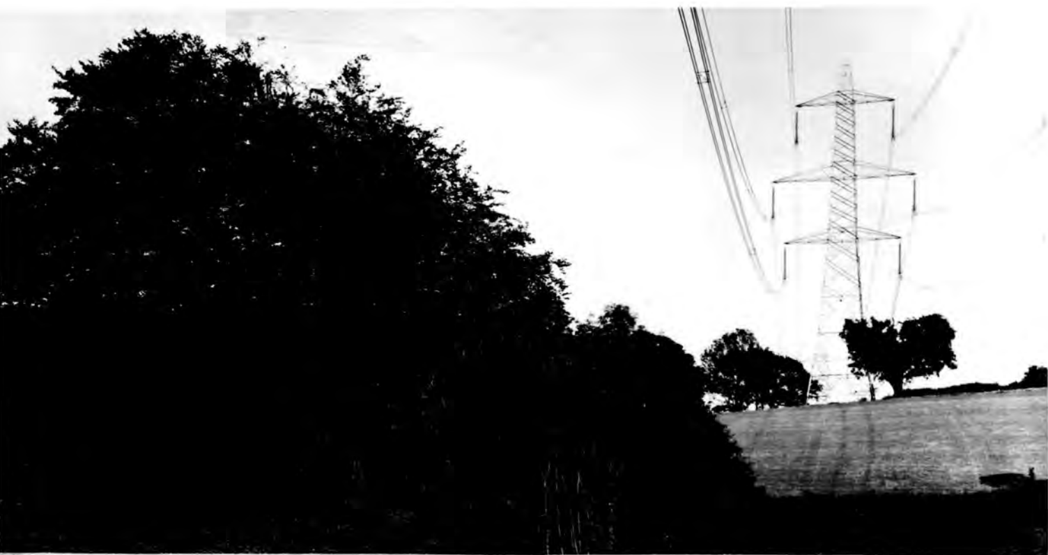
Photograph 15. A section of the Lydd-Bolney 400 kV line near Hurstmonceaux, Sussex. The two trees under the line were cut at the owners insistence to the minimum required to meet the electrical clearance regulations, and no reshaping of these trees was done. The tree in the foreground is a large Copper Beech, and this was lopped and side pruned by about 20 ft., and reshaped to conform to the natural shape of the tree.
