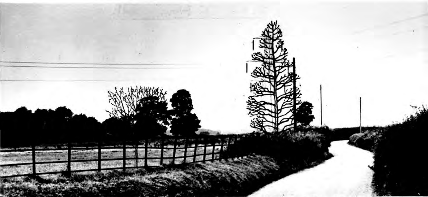
Photograph 68. Same view as above but illustrating effect of careful tree planting to focus attention away from tower.
