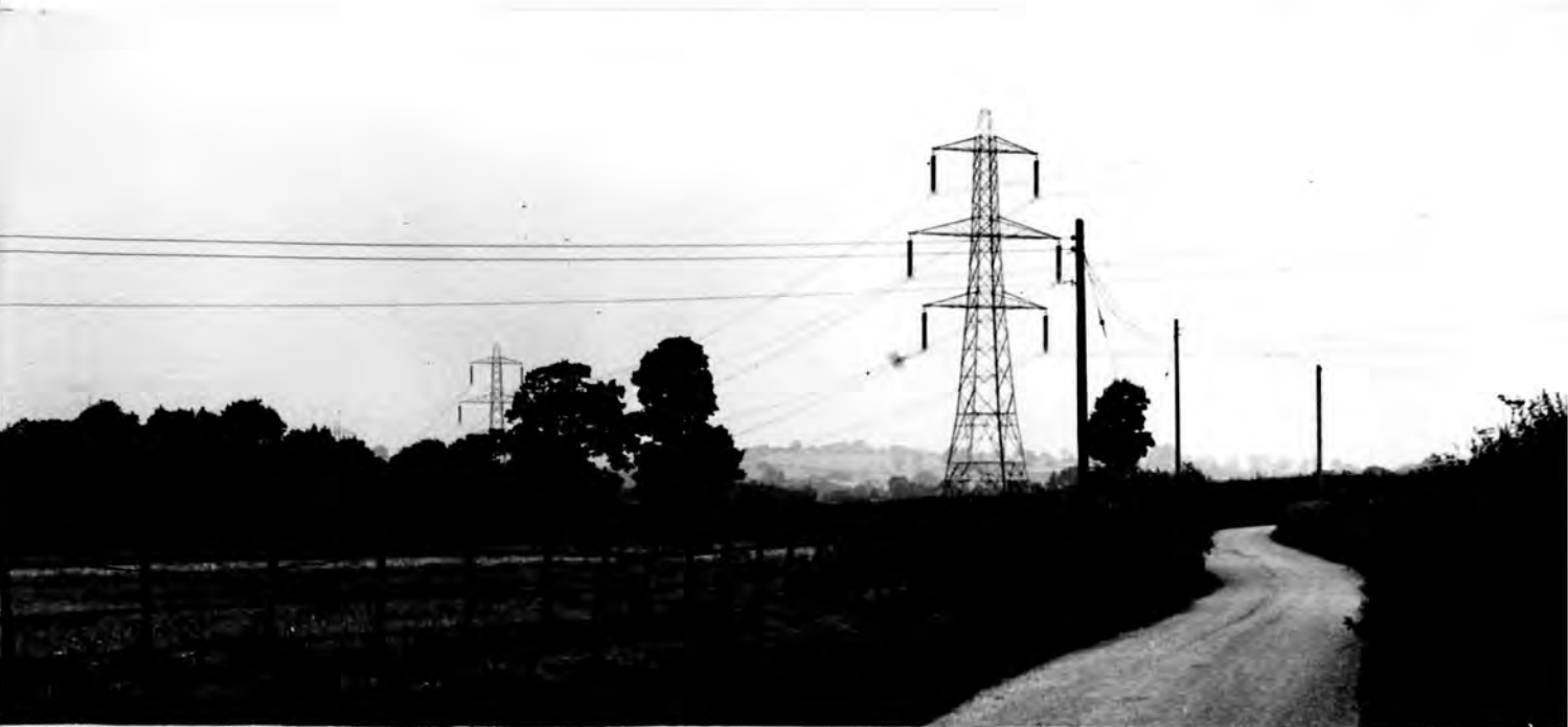
Photograph 67. 275 kV straight line tower conspicuously sited alongside highway.
