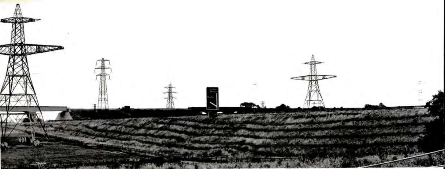
Photograph 7. Reduced height towers on Iron Acton-Locklease 400 kV line crossing M.4 motorway at Hambrook to provide safety clearance for aircraft using Filton airfield.
