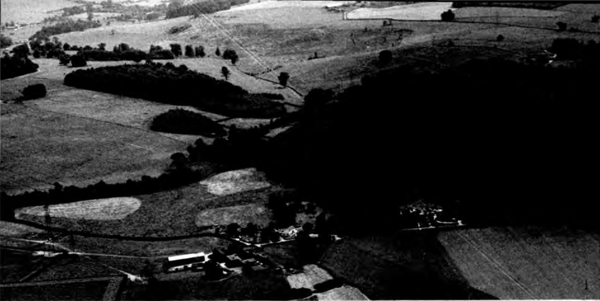
Photograph 52. Air oblique view eastwards of proposed South Buc substation with extent of electrical compounds outlined.
