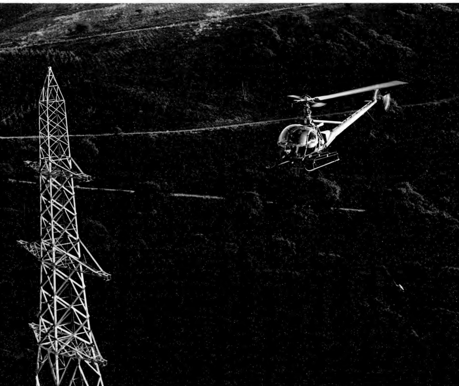
Photograph 24. Use of helicopter to carry a pilot line to link three towers on the Connah's Quay-Pentir line where they spanned the Aber Gorge in North Wales in order to prevent tree felling.
