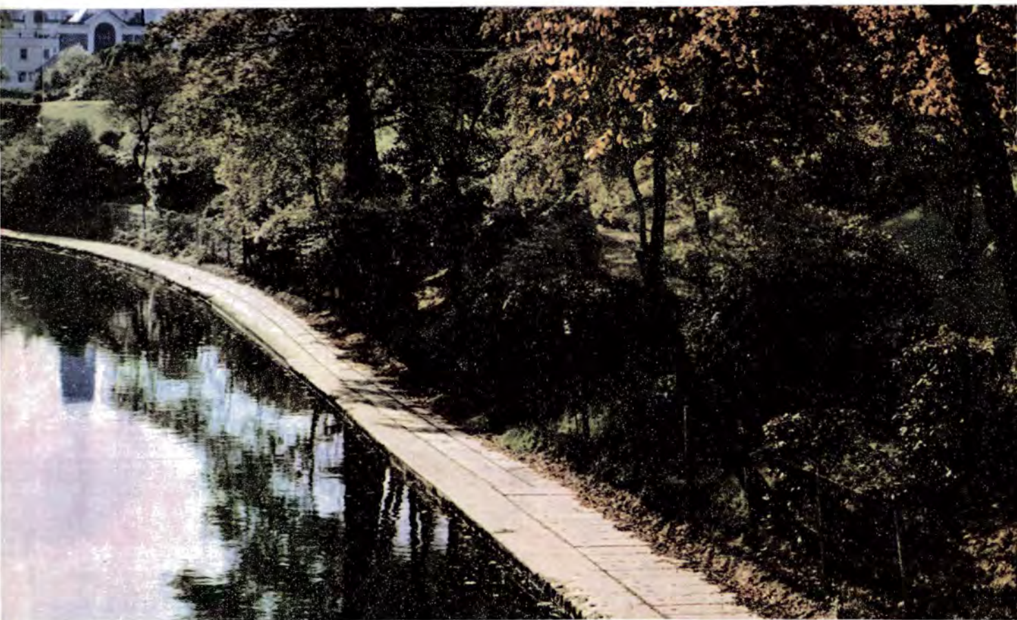
Photograph 27. Towpath of the Grand Union Canal through Regents Park, London, showing concrete covers to the 275 kV cable troughs.
