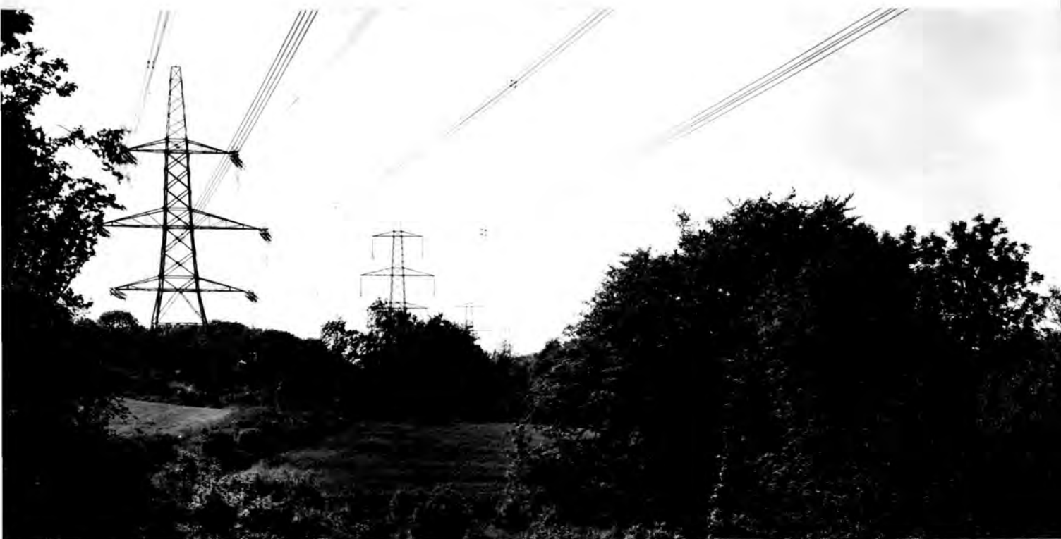
Photograph 16. A section of the Lydd-Bolney 400 kV line near Hurstmonceaux, Sussex which illustrates minimum tree cutting.
