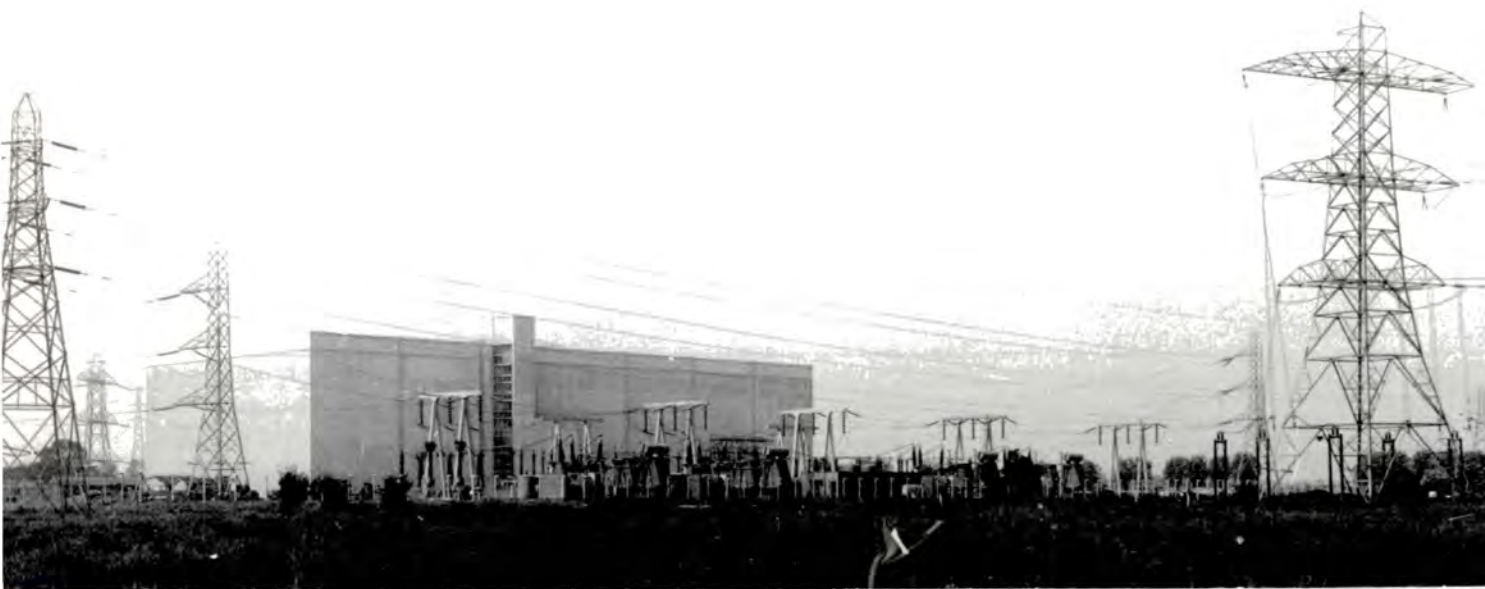
Photograph 39. Whitson 275 kV switchhouse was the first switchhouse of this size, and is typical in size and appearance to many others built in exposed situations or on restricted sites.
