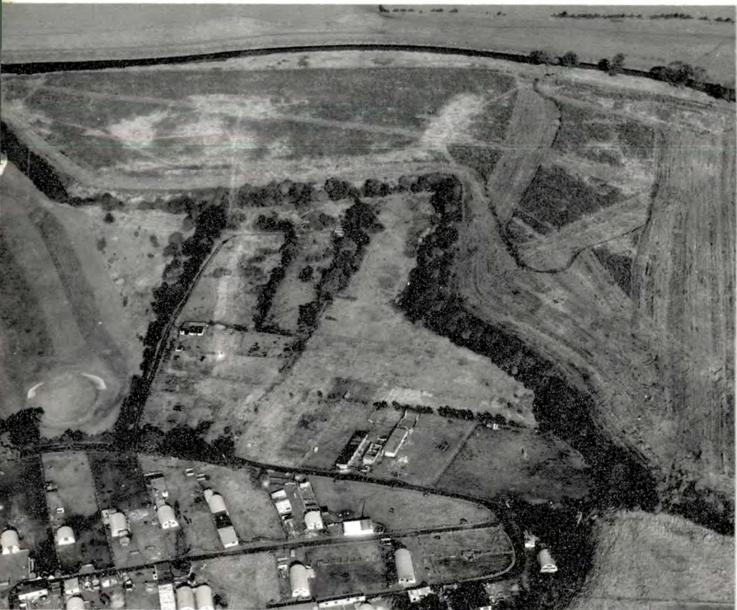
Photograph 50 showing site of South Manchester substation before construction, and the piggyery smallholdings the retention of which required an expensive modification to the substation layout.
