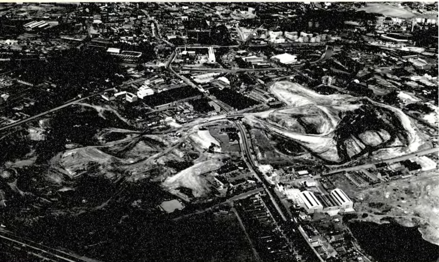
Photograph 45. Air view showing the removal of 'Blue Billy' on the right of the photograph to fill the marl pits to the left of the photograph, to form Oldbury substation site.
