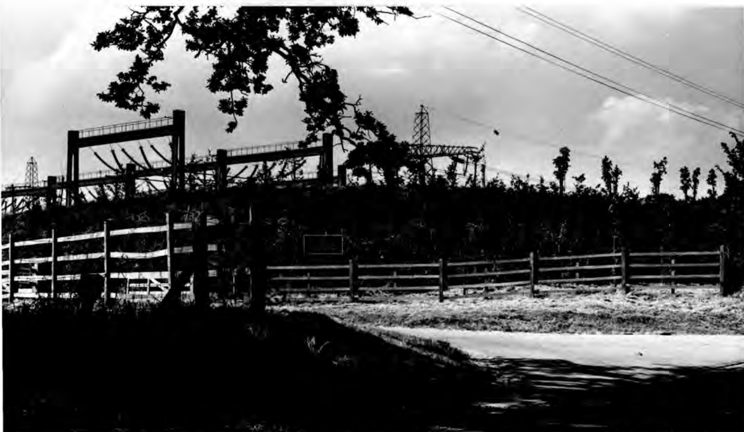
Photograph 77. The entrance to Lovedeane substation showing how the ground modelling and new tree and shrub planting provides screening for most of the substation. In a few years time one would expect the tree screen to hide the substation entirely from this view.
