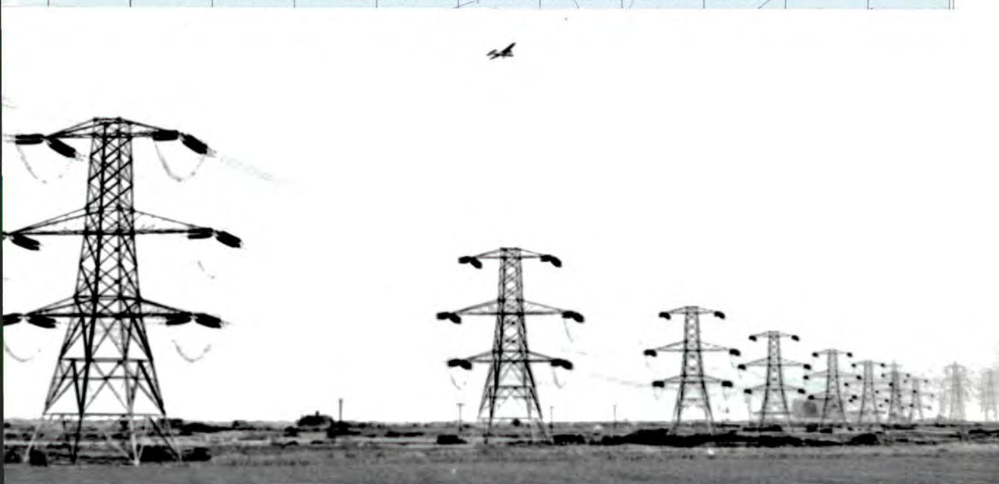
PHOTOGRAPH 8 REDUCED HEIGHT TOWERS CLOSE TOGETHER WITH TENSION INSULATORS. NOTE STANDARD HEIGHT TOWERS TO RIGHT OF PHOTOGRAPH.
