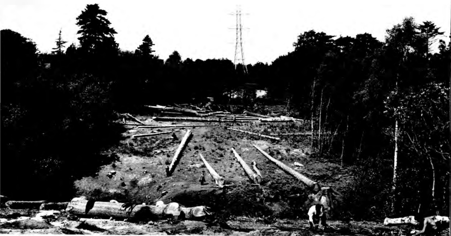
Photograph 17. A section of the Ninfield-Hastings 275 kV line under construction adjoining Claremont School near Hastings, showing deliberate uneven felling along the sides of the swathe to give a more natural effect. The scaffolding near the tower is to carry the conductors during erection to avoid damaging or felling the trees near the base of the tower.
