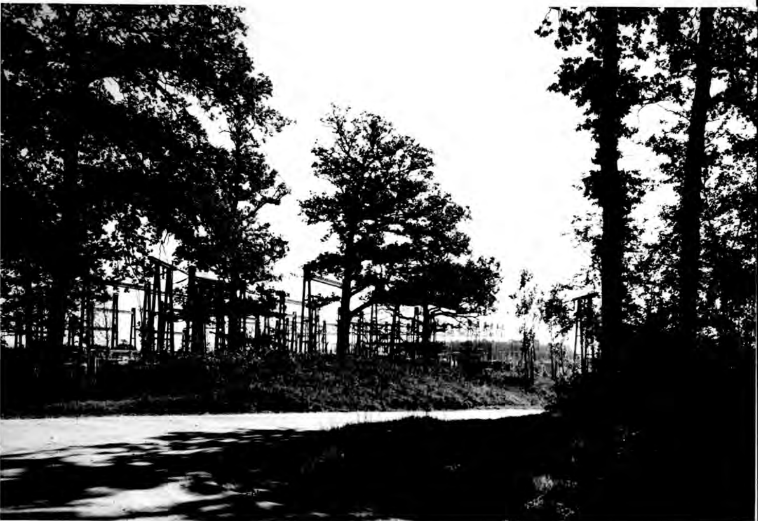
Photograph 74. Illustrating how the retention of mature trees at the entrance to Bolney Substation with the new tree planting and modest ground modelling has helped to screen and diffuse the 70' high steel supporting structures. Bolney substation is situated between Bolney and Cowfold in south-east Sussex. The site was already reasonably well screened on the south and west boundaries which have been augmented by further tree planting of indigenous species. The surplus material from the site levelling was used for ground modelling chiefly on the northern boundary of the substation and to a lesser degree on the western side of the access road. An existing dew pond was enlarged, planted with aquatic flora, and restocked with fish for the benefit of the local angling society who formerly fished there. In addition to the standard size trees, some semi-mature trees were also planted, to close particularly vulnerable viewpoints. The total cost of tree planting and ground modelling was in the order of 2½% of the total cost of the substation.
