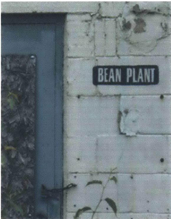
Abandoned vegetable processing buildings in cannery complex
