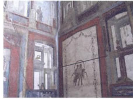
Figure 1.79 The lintels and jambs in the representation of the windows on the south and east walls do not, from this angle, connect seamlessly.
