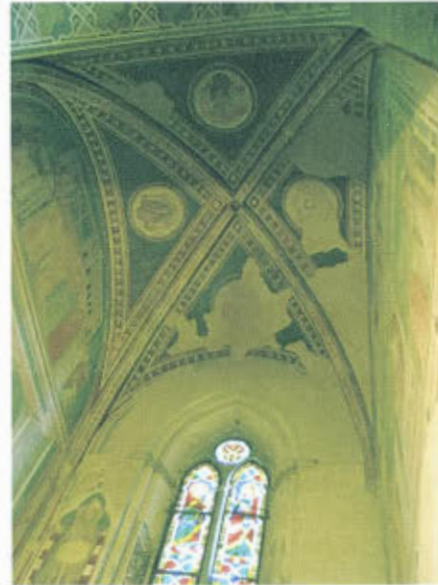
Figure 2.10 Looking up at the quadripartite vault at the ceiling of the Bardi Chapel—with four medallions representing the Franciscan virtues.
