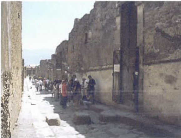
Figure 1.3 In Pompeii all the houses have adjoining walls. This is a view looking along the Via Dei Vettii with the entrance visible on the right to the House of the Vettii, 79 A.C.E.
