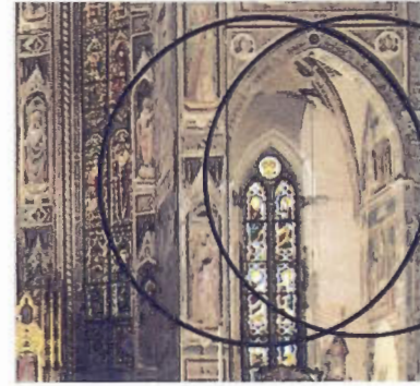
Figure 2.6 The arch that defines the Bardi Chapel at its apex is an example of squaring the circle and is typical of a Gothic arch.
