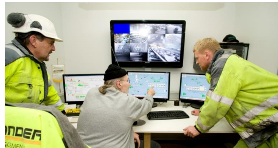
Figure 1. Operators interacting with the process via HMI/SCADA.
