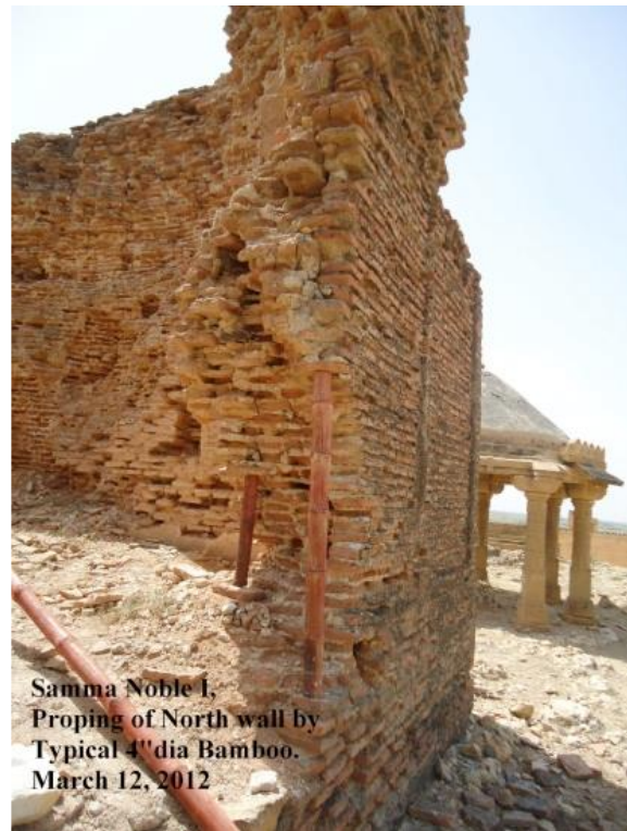
Figure 9-12: The side views of underpinning activity
