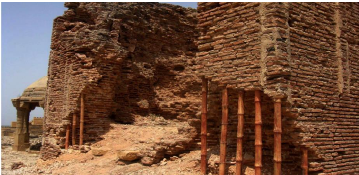
Figure 9-11: The underpinning activity executed on site
