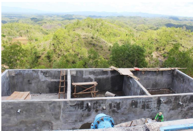
Figure 66. Construction works in Kaligoro (Fuchs et al. , 2015)
