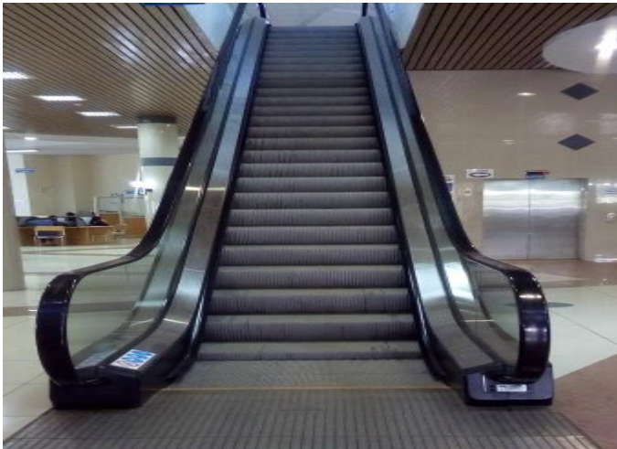
Figure 27: An elevator in one of the libraries (Source: Field data, 2017)
