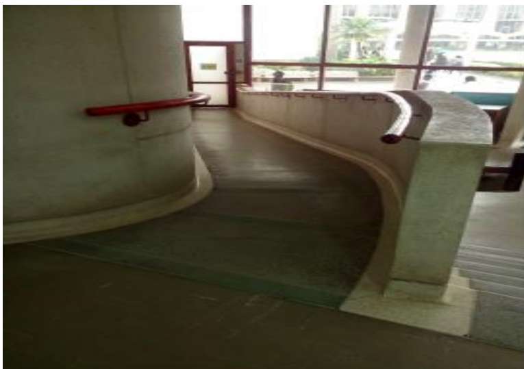
Figure 21: A ramp with hand rails on both sides (Source: Field data, 2017)
