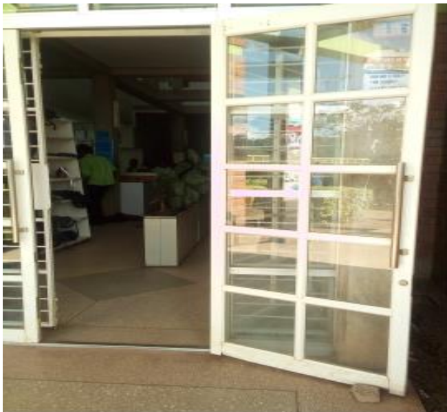
Figure 25: A double door closed on one side at one of the libraries rendering it narrow (Source: Field data, 2017)
