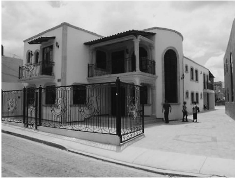
Figure 2. Partial Rustico-type residence.
