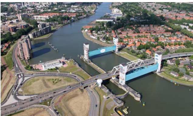
Figure 1: The Algera Complex [beeldbank.rws.nl].
