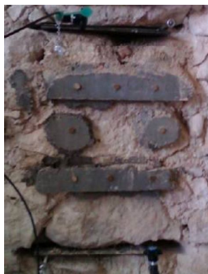
Figure 20 Flat jack test on masonry: test set-up (see online version for colours)
