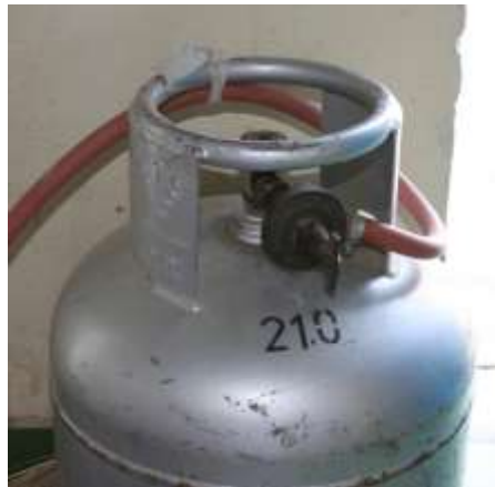
Figure 409 A gas cylinder with on/off valve, pressure reducing valve and hose © Khalid Al Busaidi
