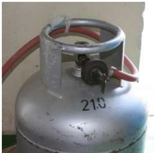
Figure 384 Gas cylinder, hose and pressure reducing valve © Khalid Al Busaidi
