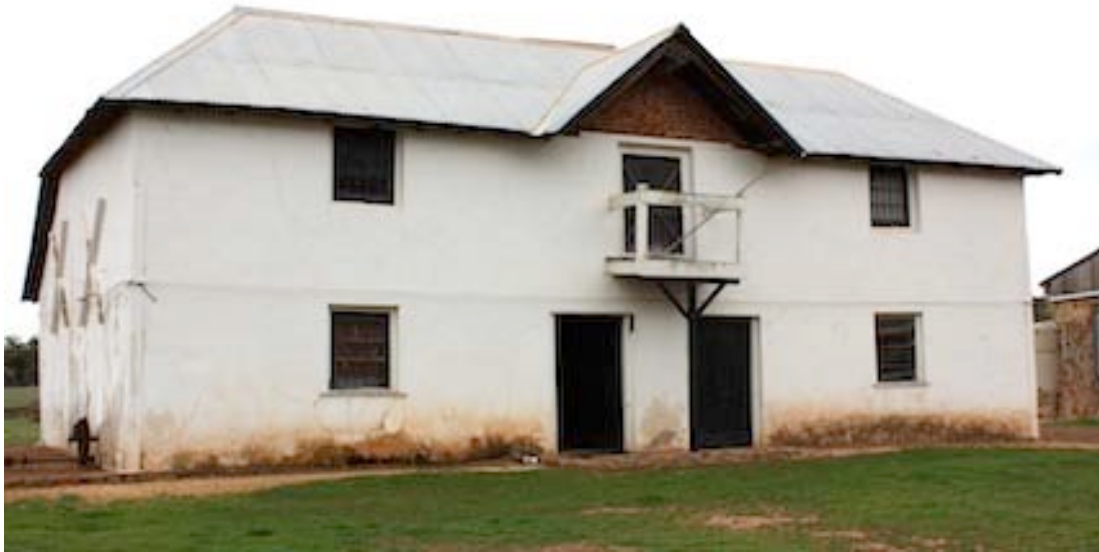
Figure 5 Front view of Mill Building
