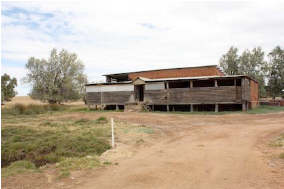
Figure 11 View of northern side of Shearing Shed
