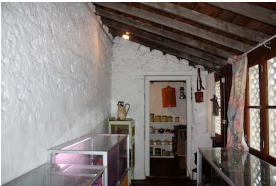
Figure 9 Rear verandah area looking east towards Room 5
