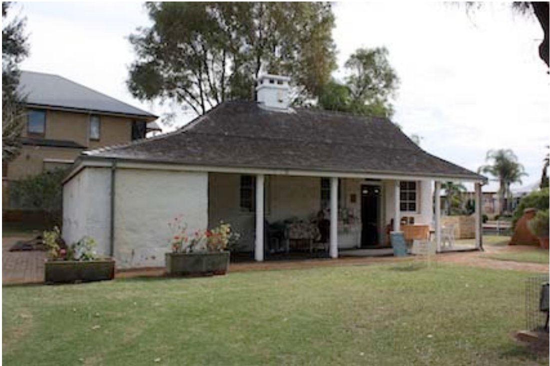
Figure 2 Front view of Hall's Cottage with slightly later addition on left side
