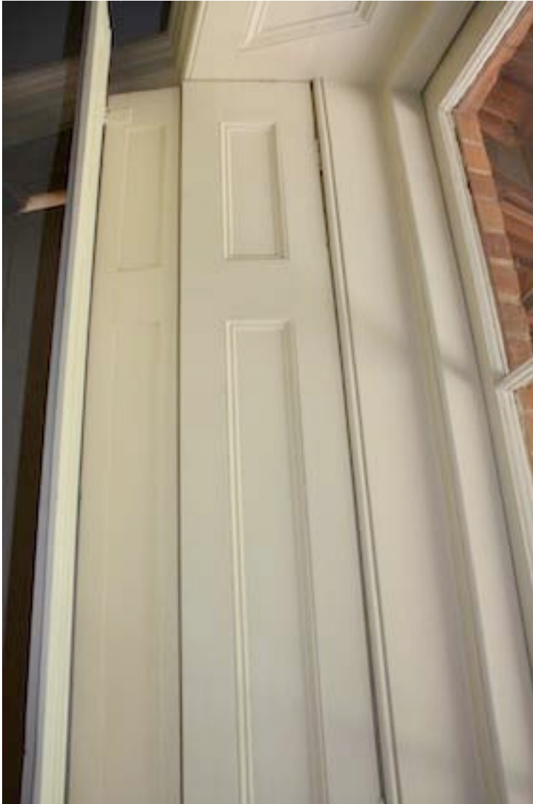
Figure 10 Detail of shutter housing in French doors in bay window.
