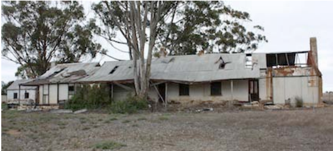
Figure 2 Eastern (front) side of Homestead with originally detached kitchen on left and later addition to right
