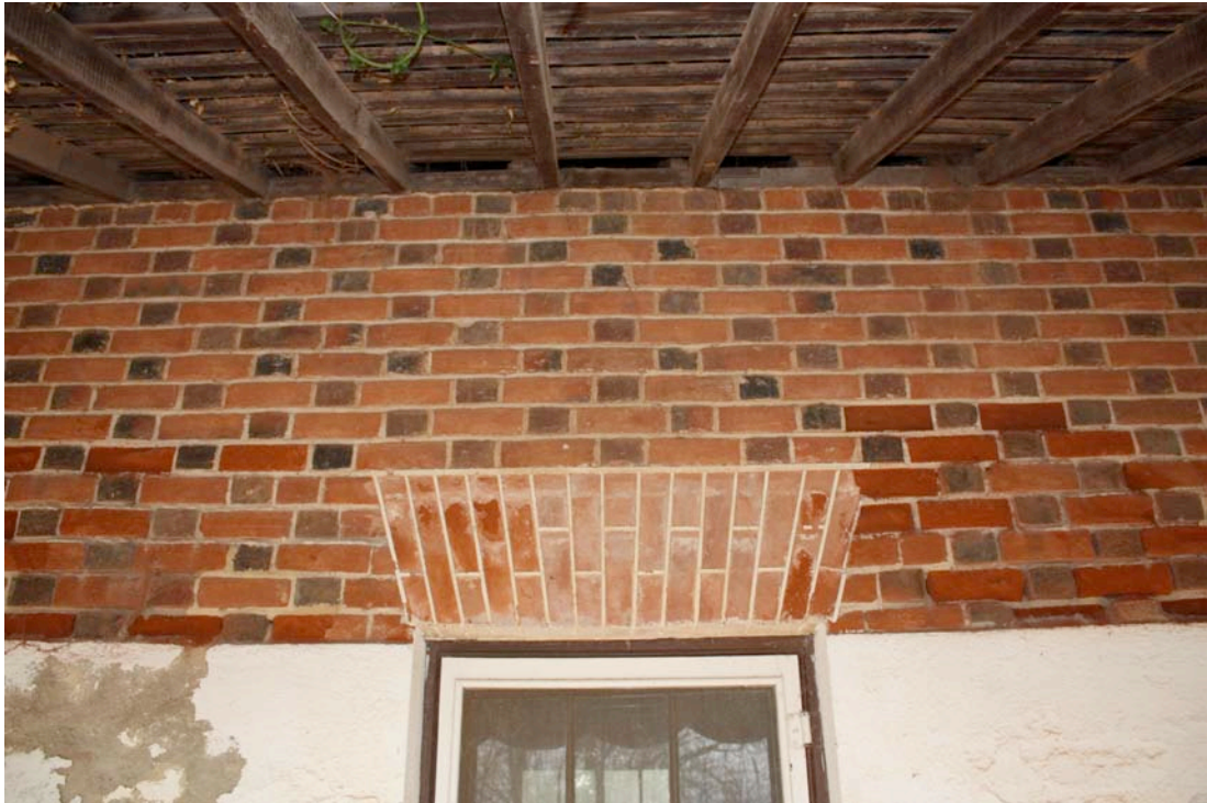
Figure 28 Detail of brick arch above one of the doorways to the guest rooms. Note Flemish bond brickwork.
