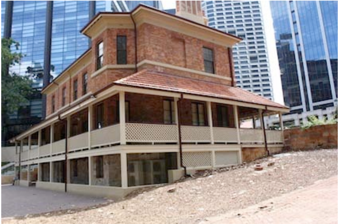
Figure 4 South-east corner of building showing basement level.
