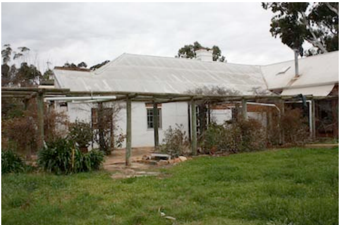
Figure 14 Southern side of Manager's House with new addition on right
