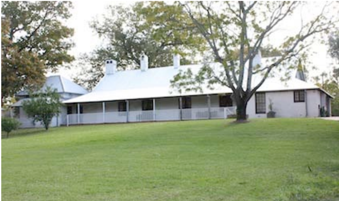
Figure 2 South side of Tranby. The detached store room is on the left and on the right are the extensions built in 1920s
