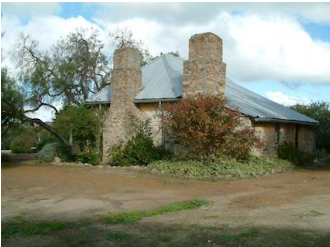
Figure 5 Northern side of building. Note differences between the two chimneys.
