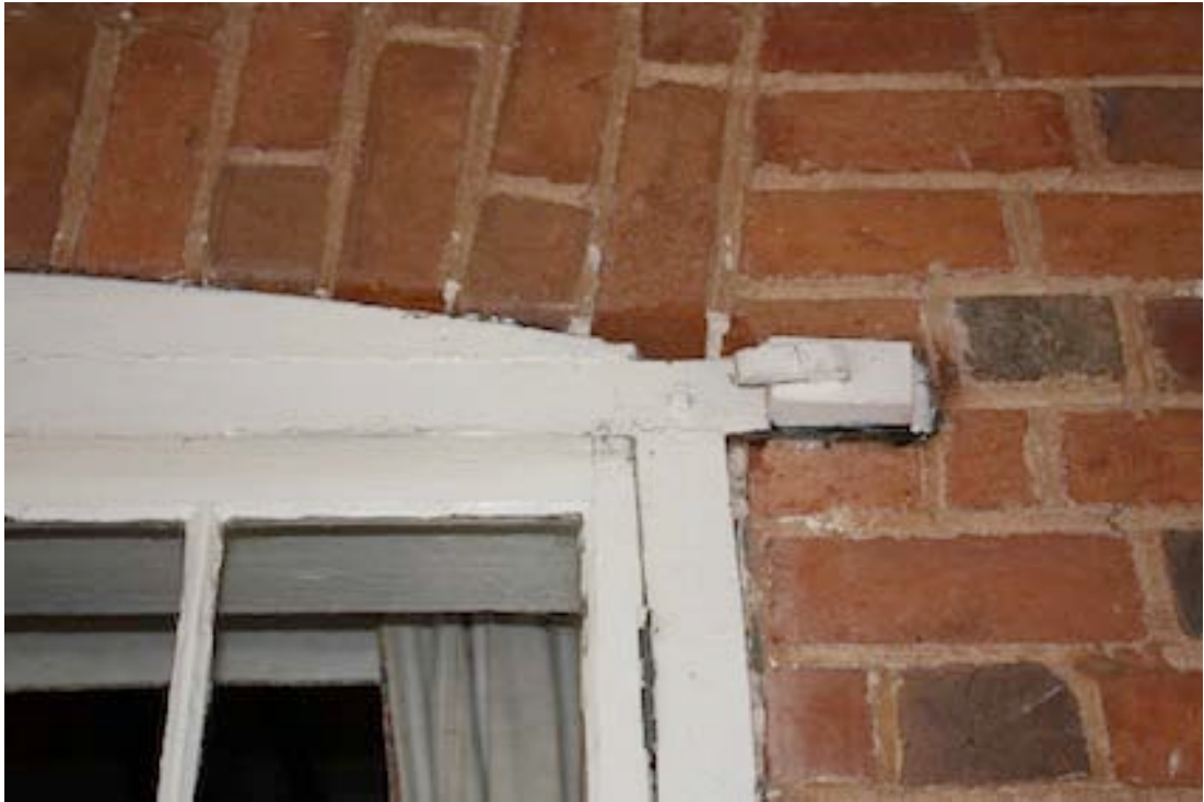
Figure 17 Detail of window frame and brickwork
