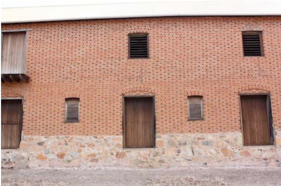
Figure 13 Detail of eastern side showing brick arches above door and window openings.
