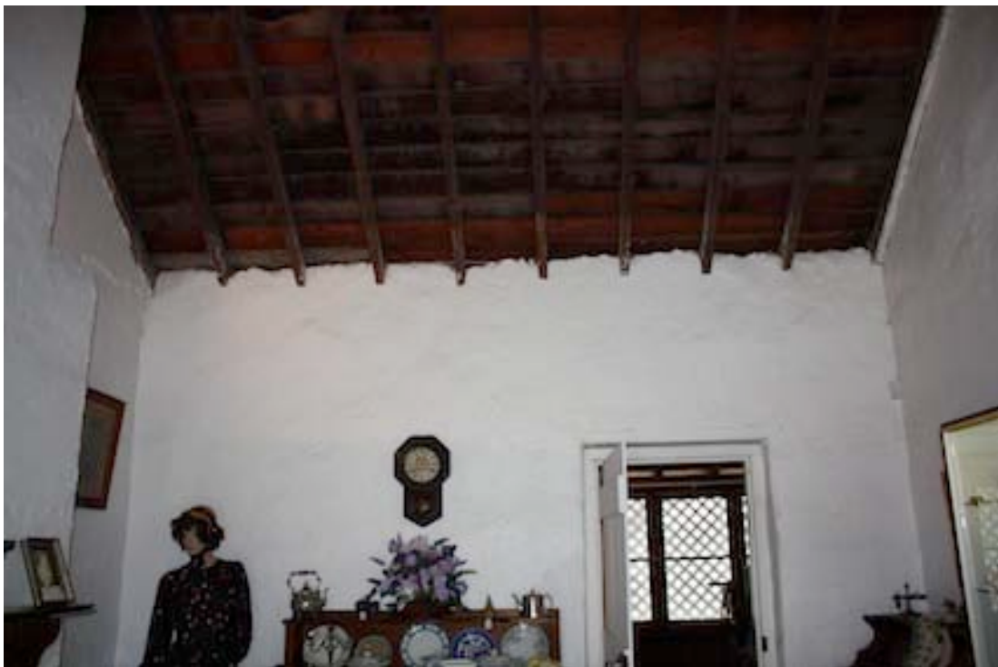
Figure 7 Interior view of Room 1 looking towards back verandah area.
