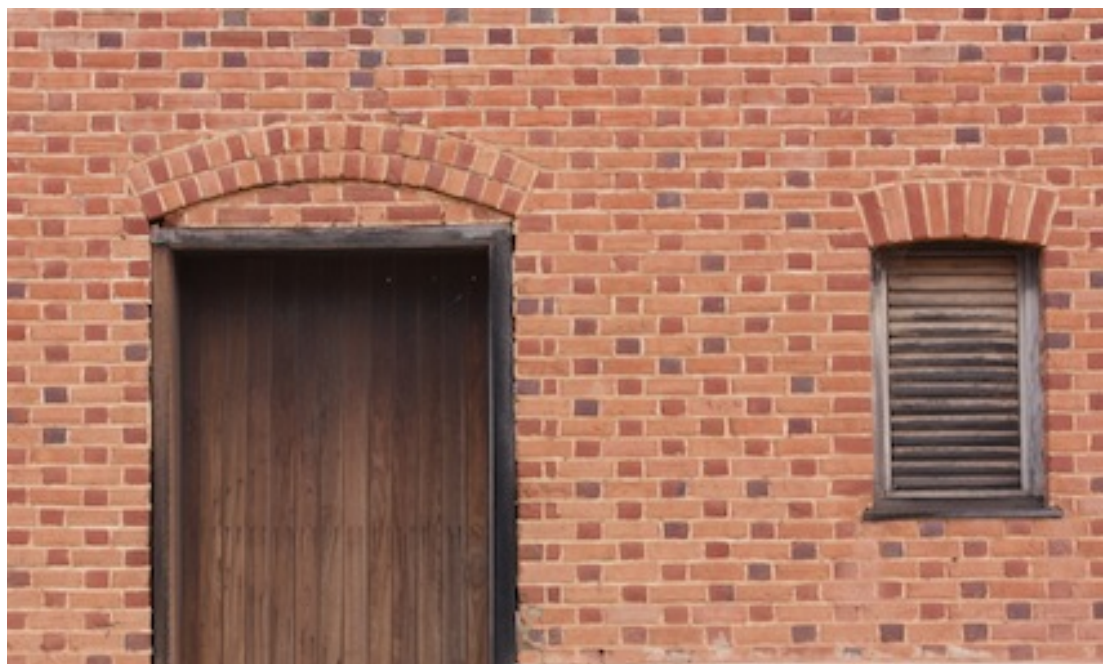
Figure 8.10 Brick relieving arches on the Stables at 'Glentromie' (F. Bush 16 March 2010)
