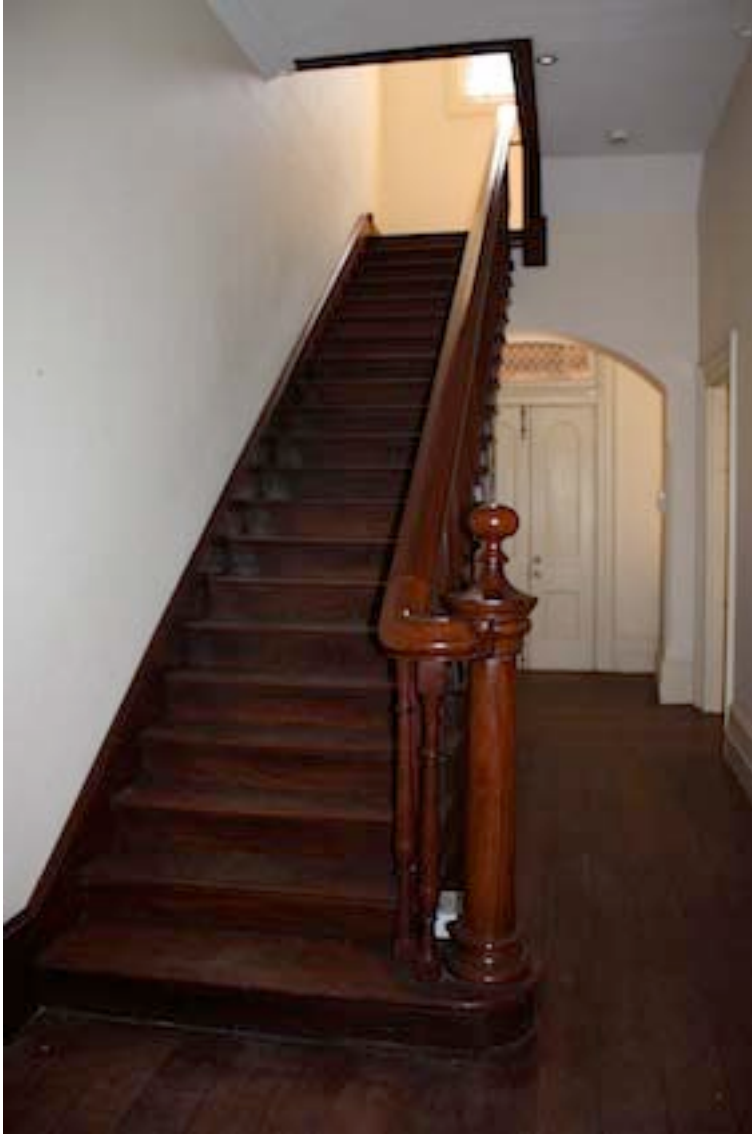
Figure 11 Detail of staircase in main entry hall, looking north.
