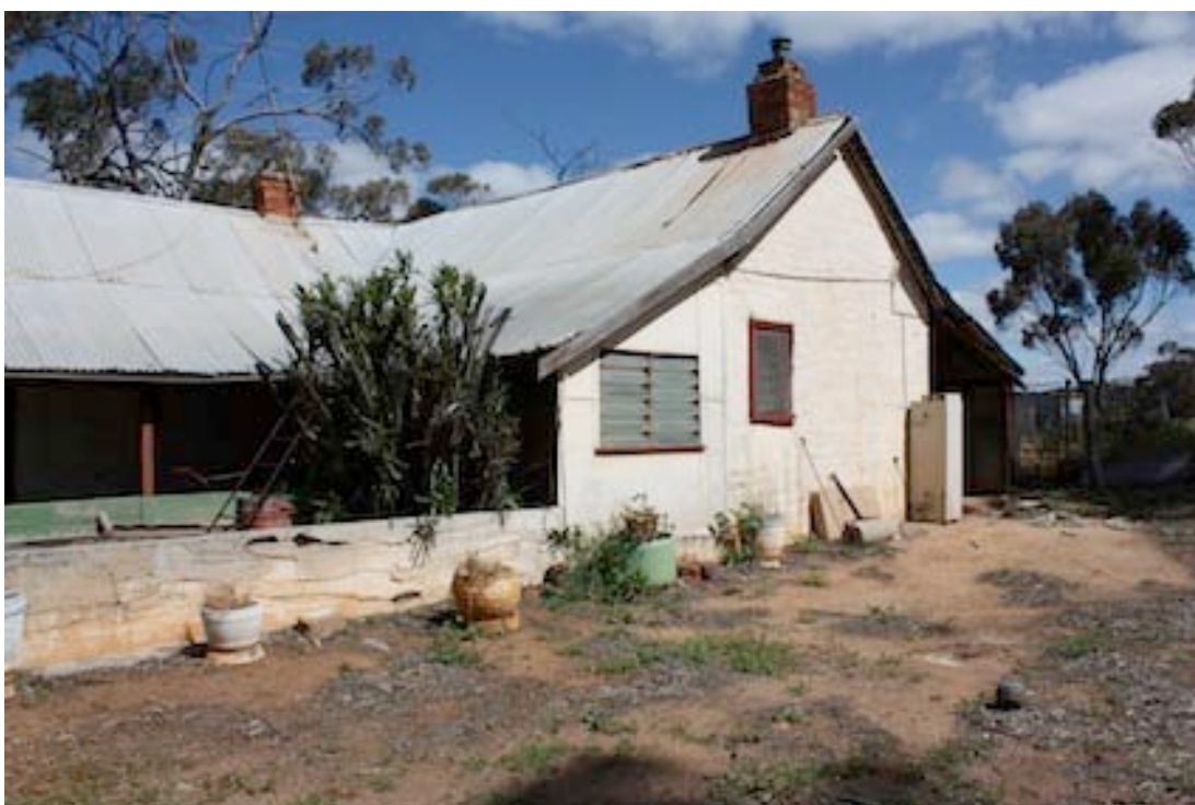
Figure 3 South eastern end of the building showing the kitchen wing
