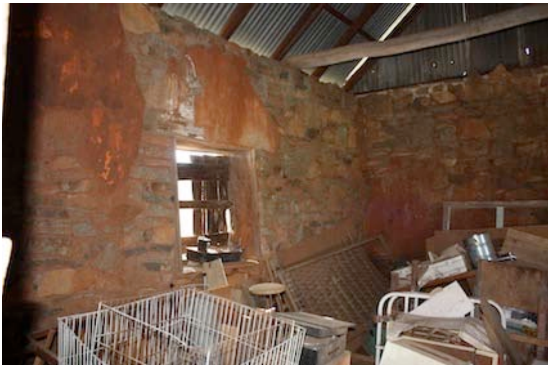
Figure 13 Interior view of building looking towards the north-east corner. Note the remains of the mud render above the window
