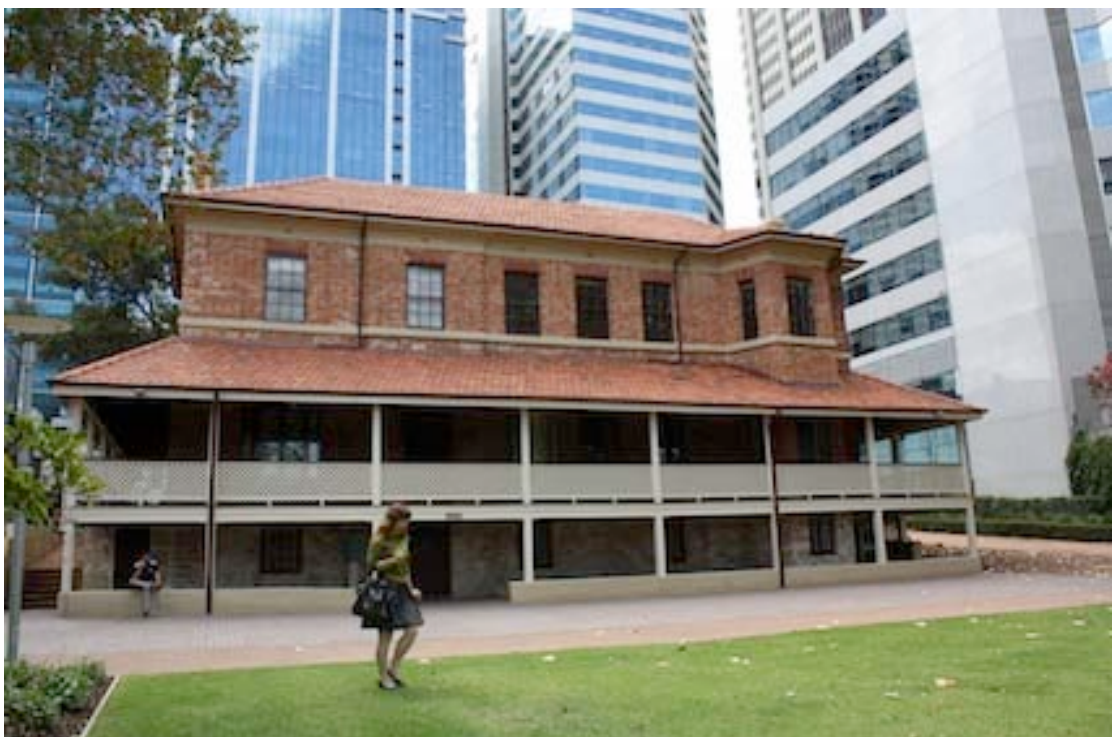
Figure 3 Southern side of building.
