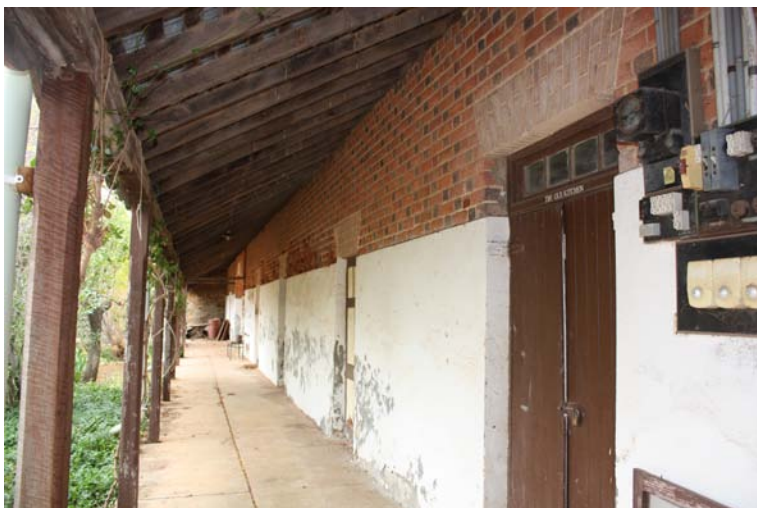
Figure 8.16 Southern side of Gate House (F. Bush 11 August 2010)
