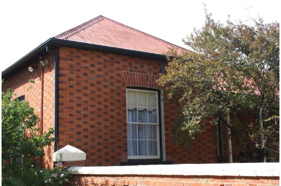
Figure 7.12 Detail of brickwork on Wansborough House (F. Bush 20 April 2011)
