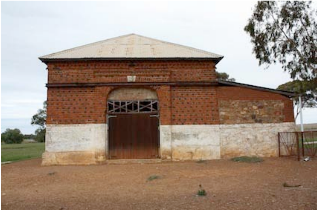
Figure 40 Northern side of building which displays high attention to detail in the laying of the bricks in Flemish bond and also the detailing of the doorway arch.
