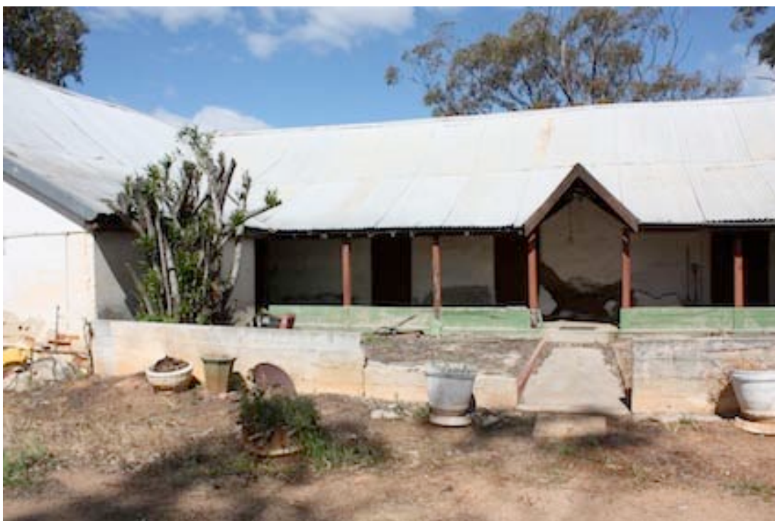
Figure 2 Eastern side (front) looking towards the northern end
