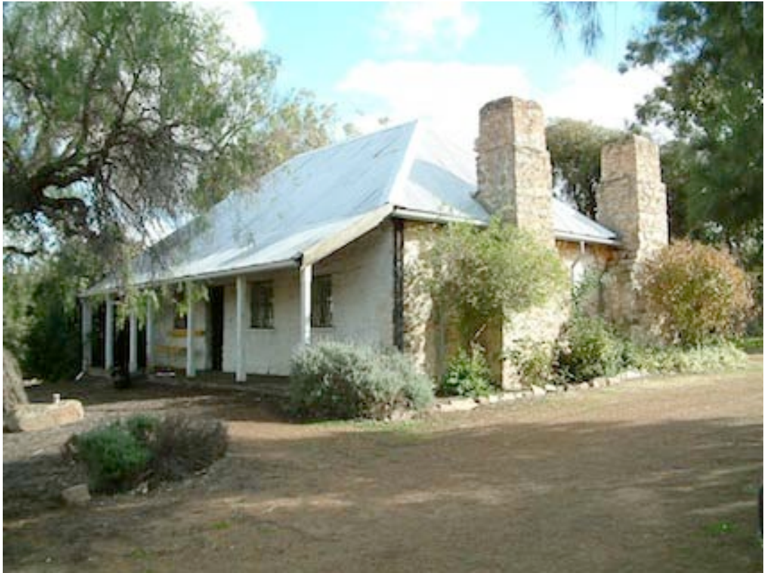
Figure 2 View of south-east corner showing first section and later skillion addition at rear
