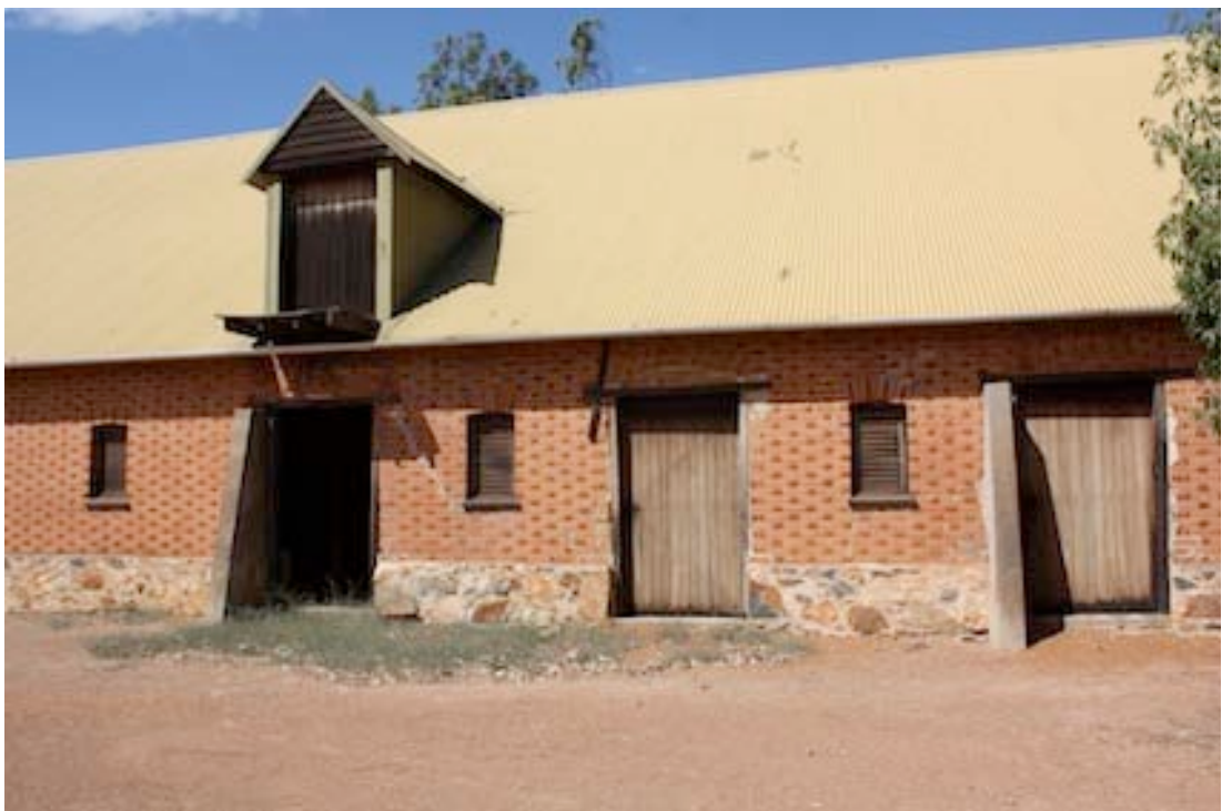
Figure 12 Western side of stables, southern end.
