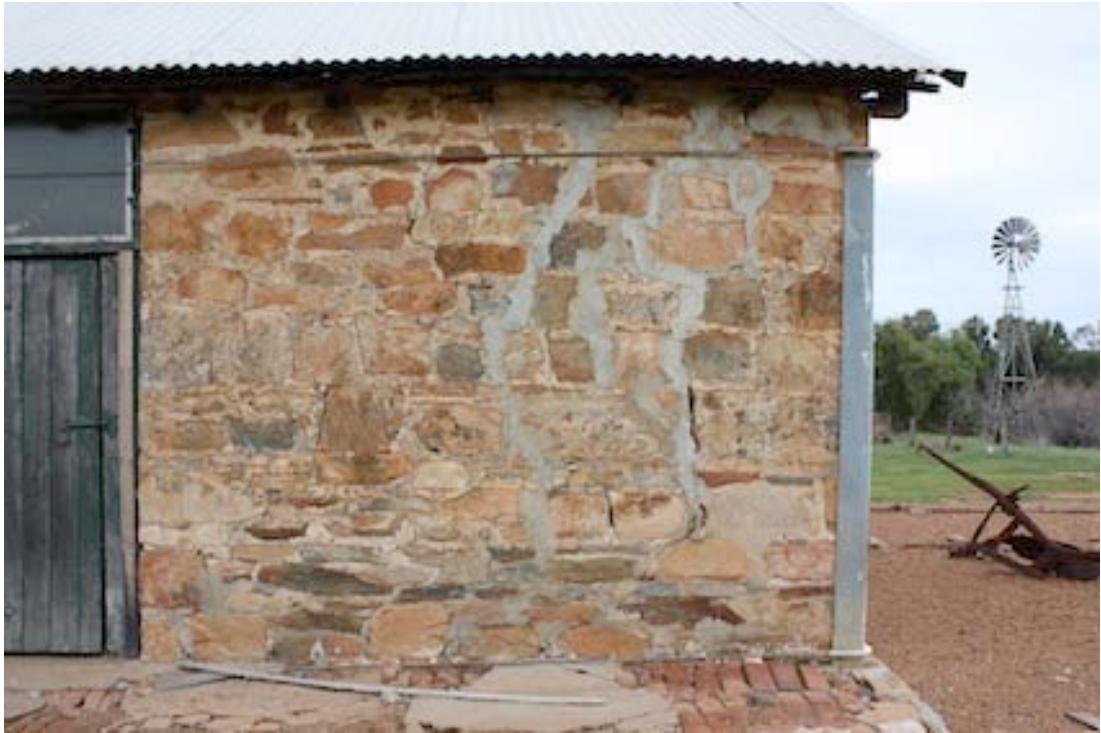
Figure 7 Detail of rear (north) wall showing stonework.
