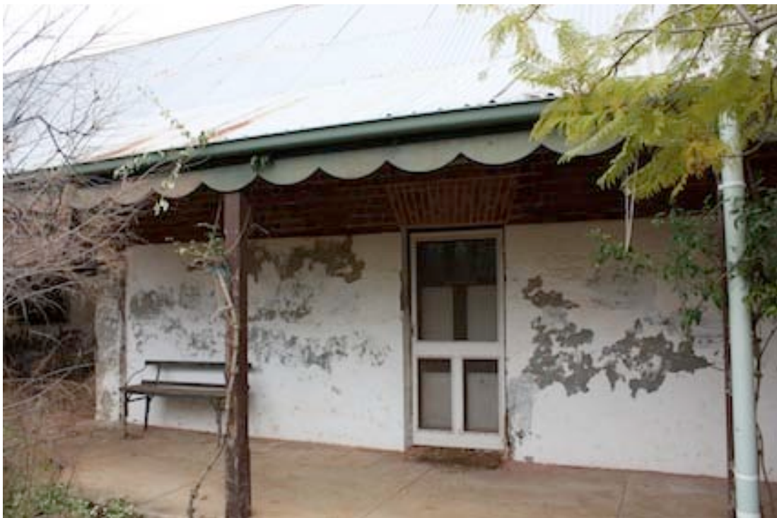
Figure 25 Detail of valance on the verandah.
