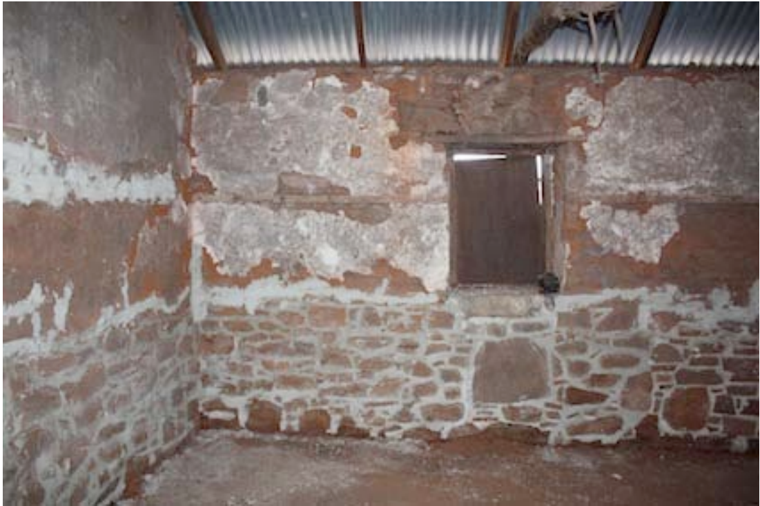
Figure 26 Interior of southern section.
