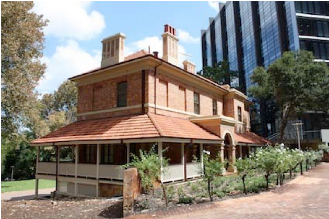
Figure 2 North-east corner of the building showing front portico where the main front door is located. Note the two infilled brick windows on the north side and the single window on the east side.
