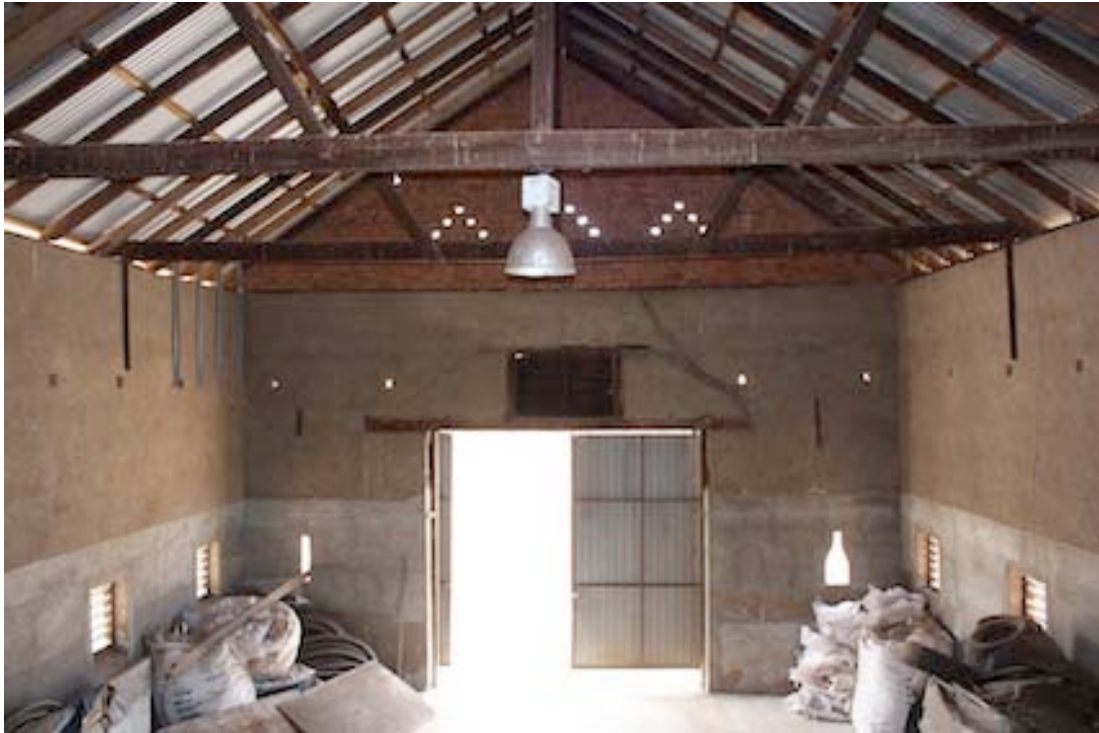
Figure 31 Interior view of Stables looking east.
