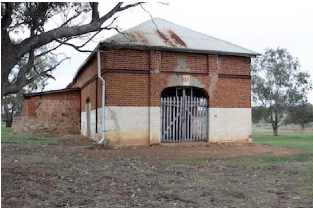
Figure 41 Southern side of building.
