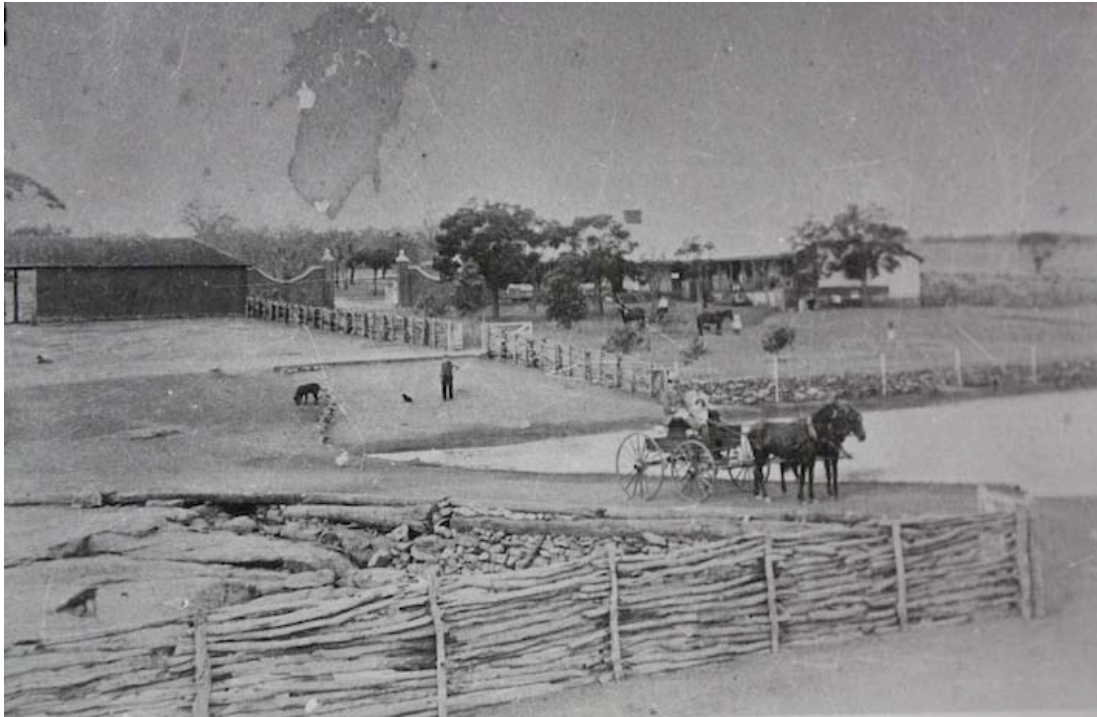
Figure 1 View of property looking towards the Homestead and the former arched gateway. The building to the left of the gateway may be the carriage house, now referred to as the Blacksmith's Building (reproduced with permission of Duncan Young)
