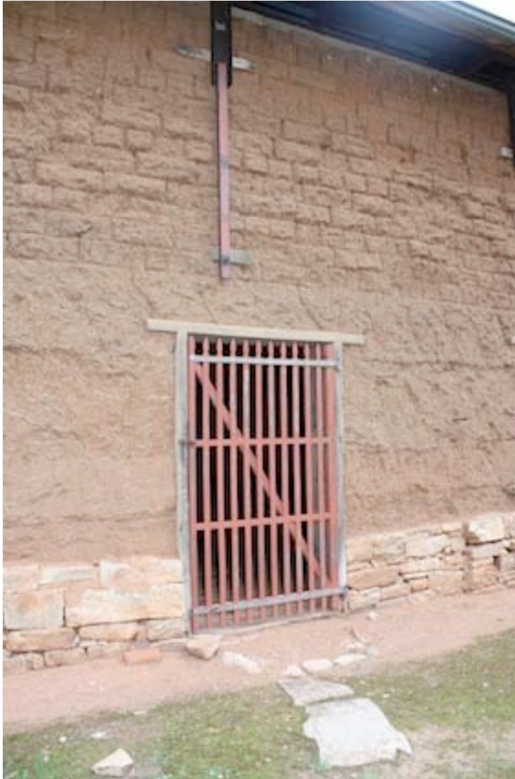
Figure 32 South side (front) of Stables. Note cob walling to the ground floor and then the unfired bricks above.
