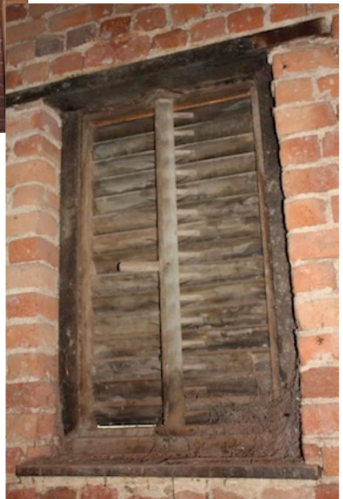
Figure 20 Louvered window: the shaft fits into metal bearings at the top and bottom of the window and when rotated open or close the louvers .
