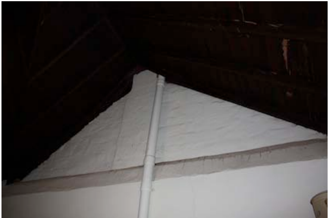
Figure 17 Detail of western wall of Room 4 showing extension to this wall
