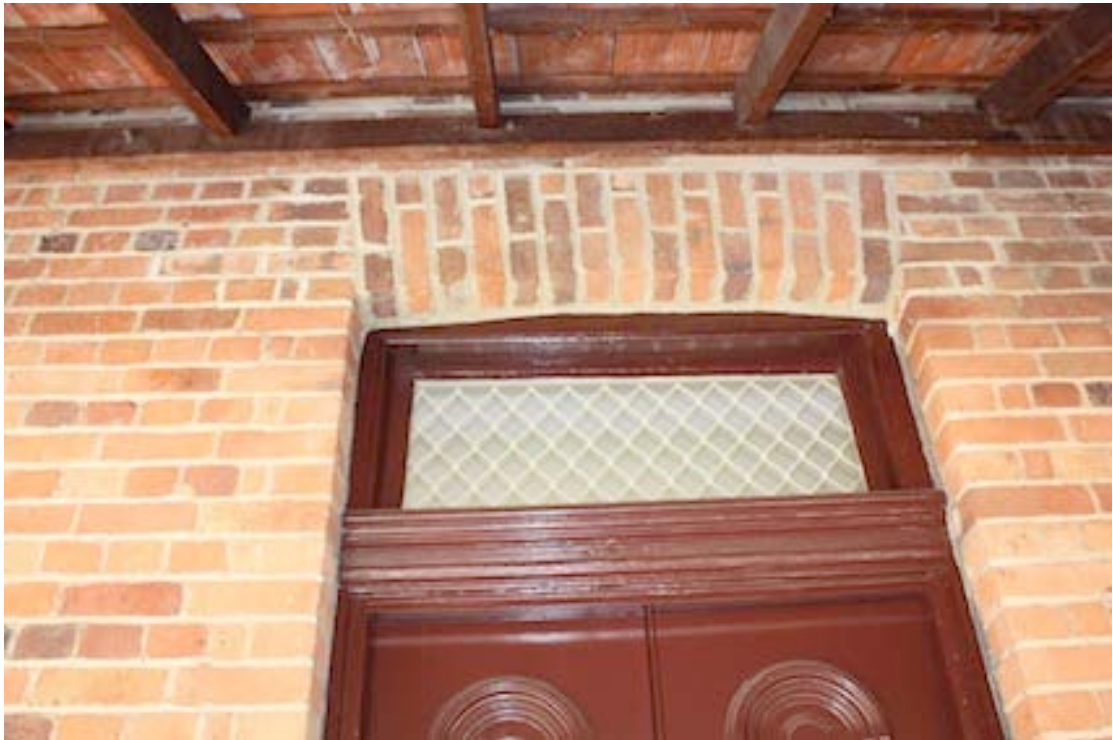
Figure 8 Detail of secondary door on the northern side.
