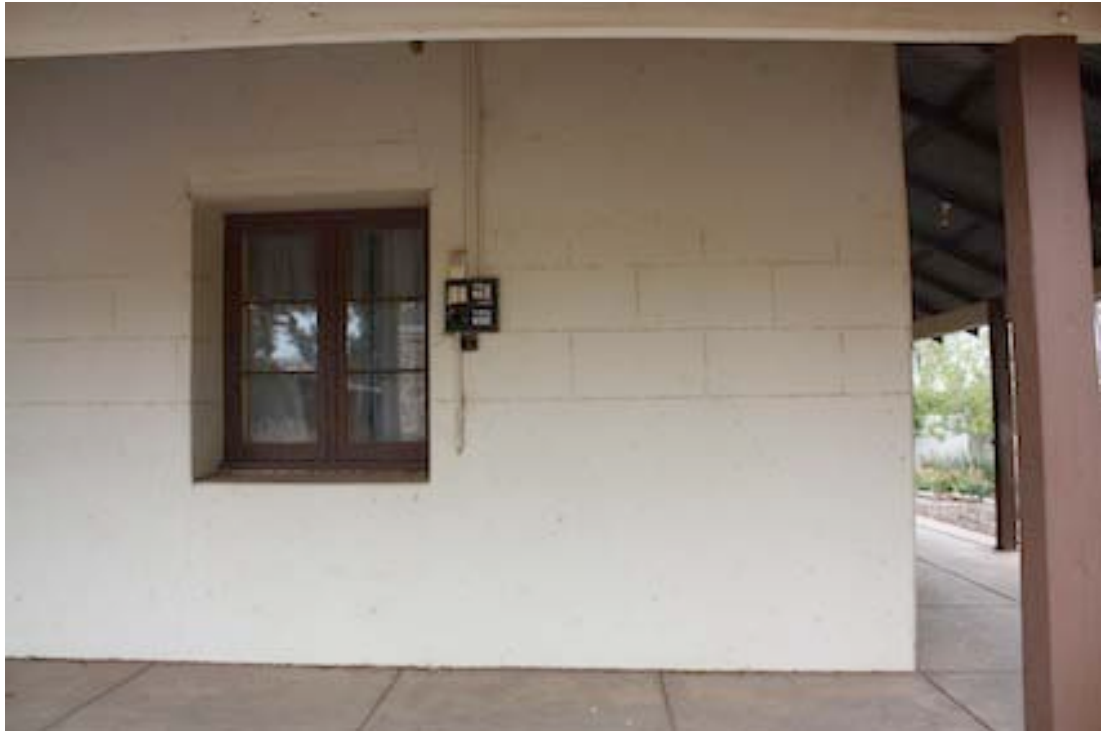
Figure 6 Detail of southern side showing lines of wall imitating dressed ashlar masonry. Note casement windows
