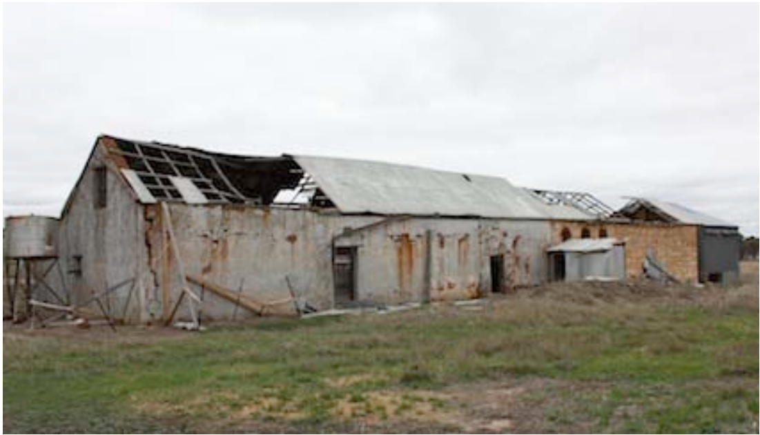
Figure 22 North-west corner of building with the Wool Barn on the left, the stone Shearing Shed in the Centre and the later steel shearing shed on the extreme right
