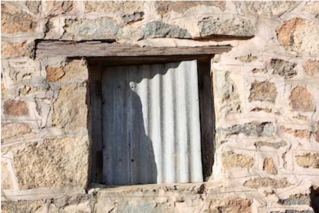
Figure 29 Detail of window on western side of building
