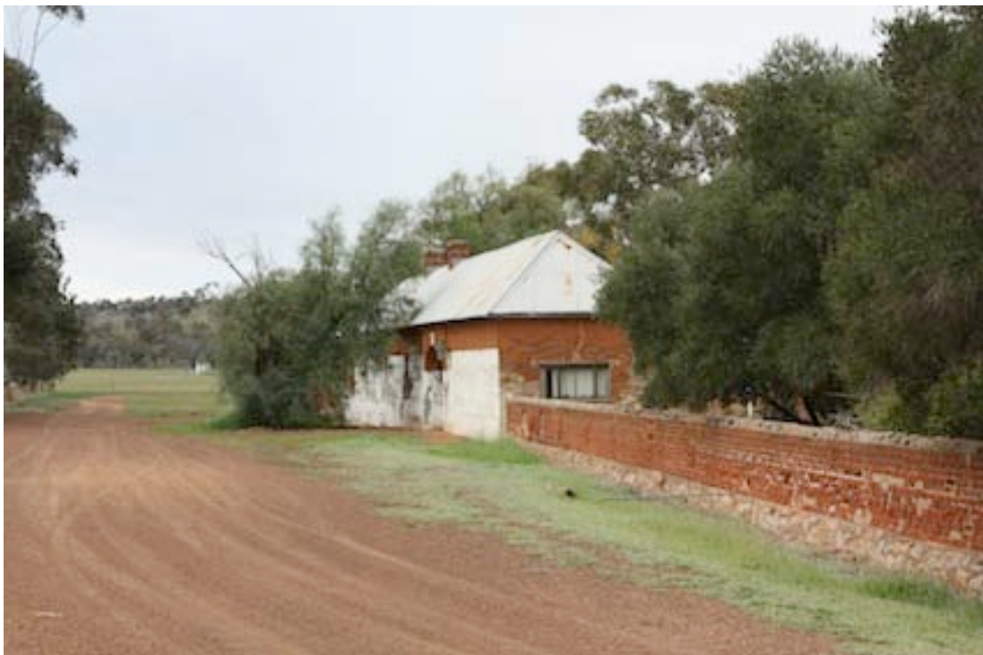
Figure 23 Gate House viewed from the west. Note the brick enclosure wall on the right.
