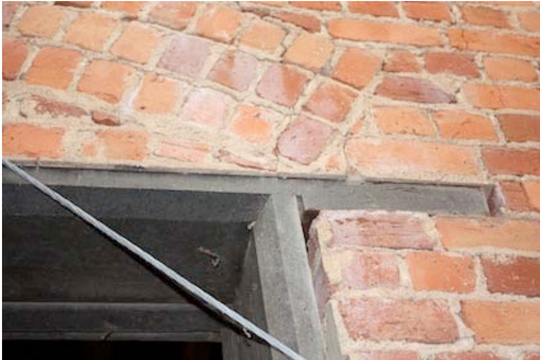
Figure 29 Detail of door frame in eastern wall of western section. Note chamfered edge.
