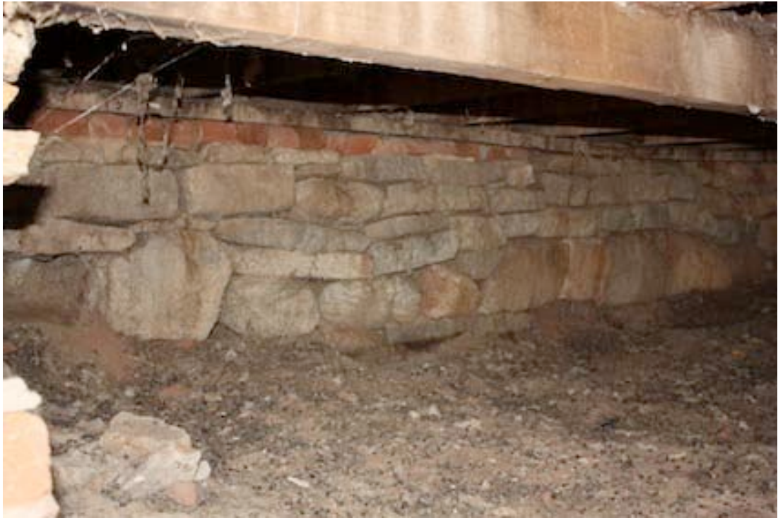
Figure 13 Detail of the Shearing Shed's brick foundation
