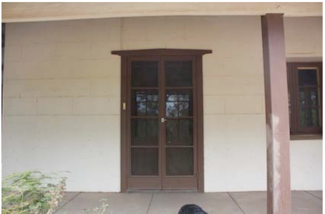
Figure 7 Detail of French doors and flyscreens on eastern side
