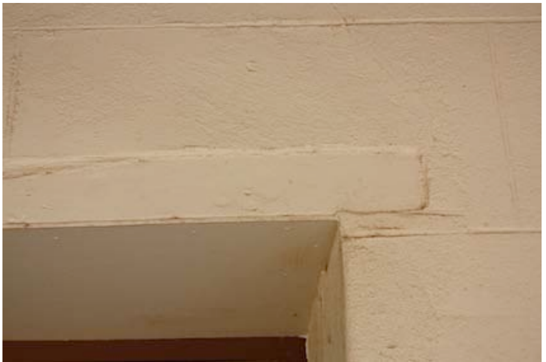
Figure 9 Detail of lintel above window opening
