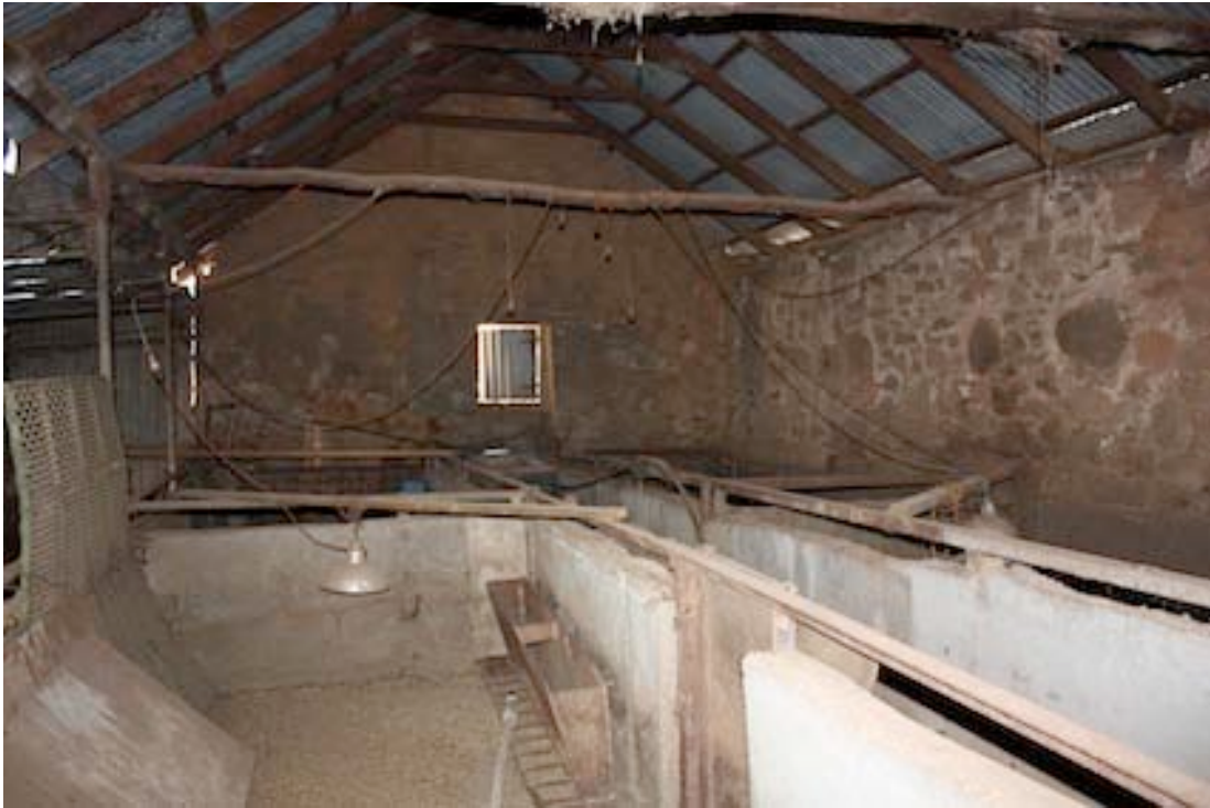
Figure 28 Interior view of southern section showing concrete walls and pig pens
