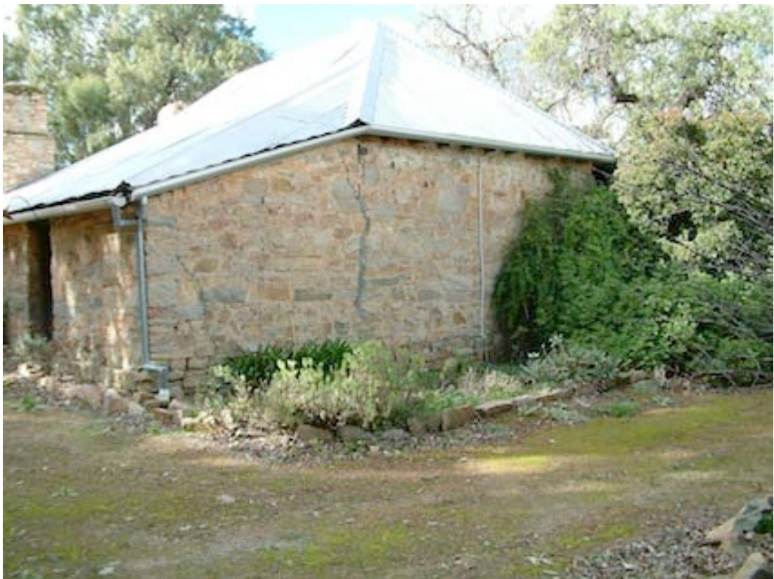
Figure 3 View of rear south-west corner
