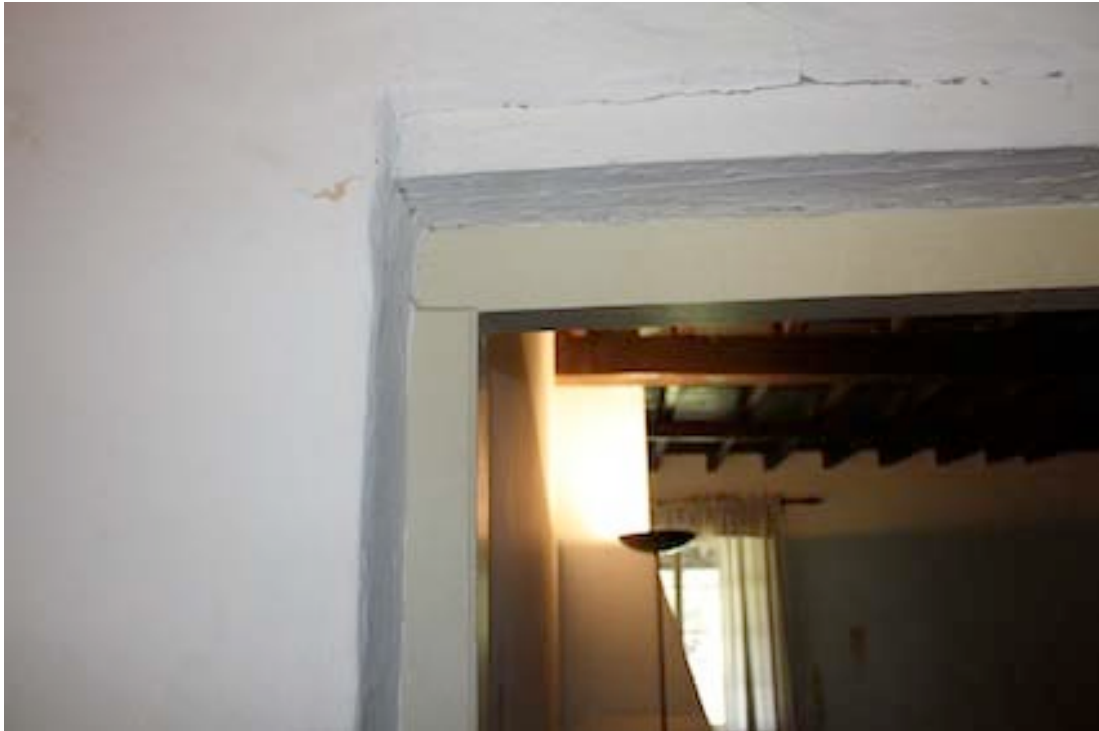
Figure 8 Detail of door frame which was joined with a mortise and tenon joint and a wooden dowel
