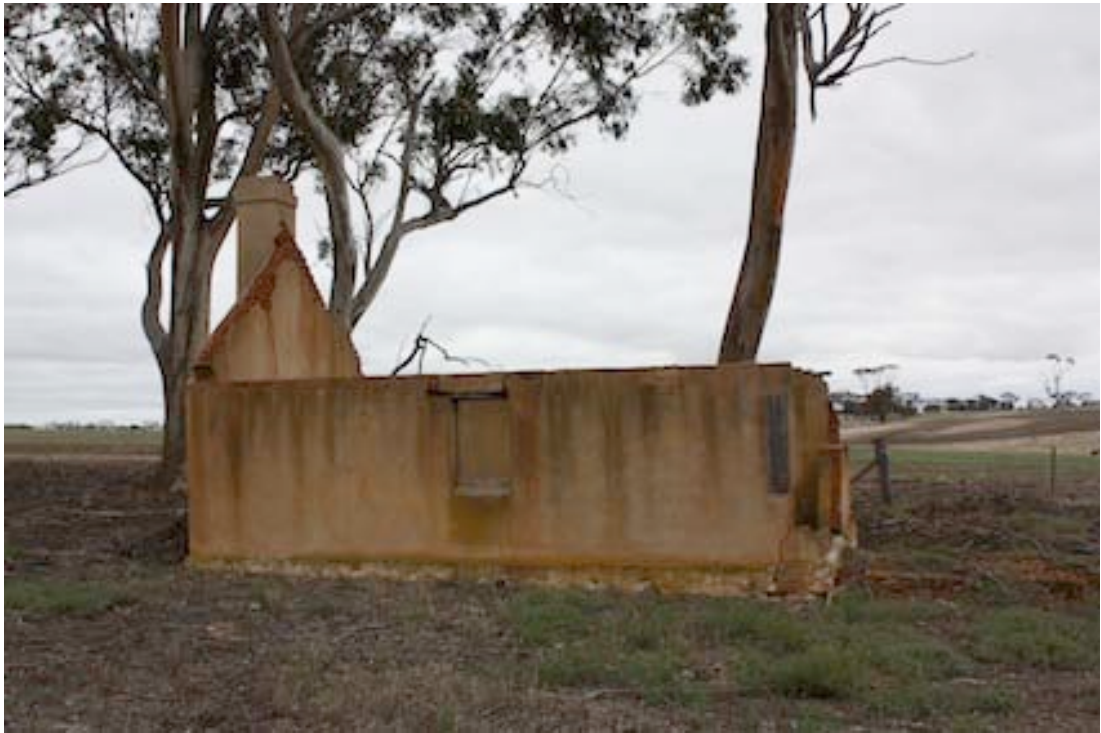
Figure 14 Eastern side with collapsed wall on the right (northern end)
