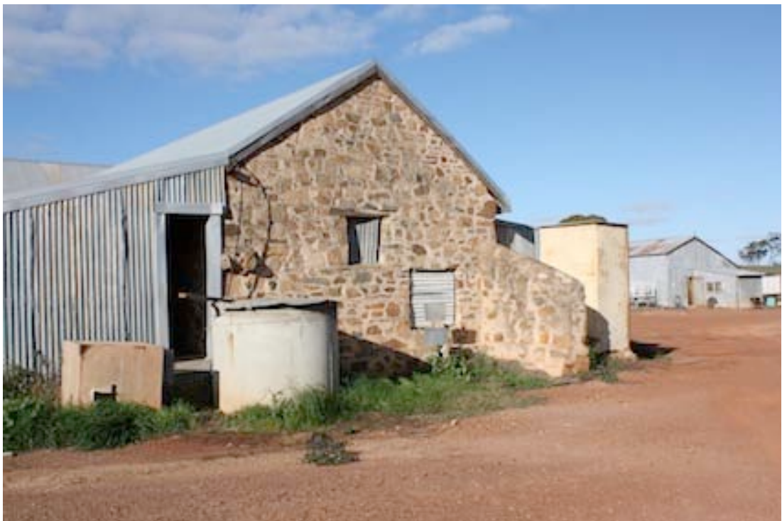
Figure 25 Western side of Stables. The iron clad wall on the left replaces a stone wall. This wall can be seen in a 1959 photograph in the conservation plan
