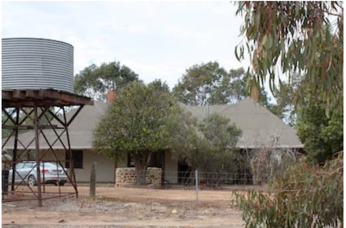
Figure 2 Front (western side) of Boyadine Homestead
