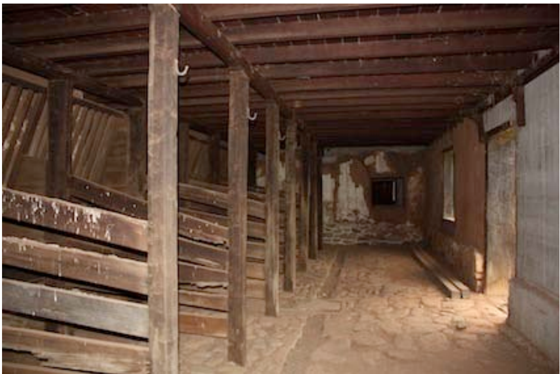
Figure 34 Horse stalls on the southern side of the Stables, looking east.
