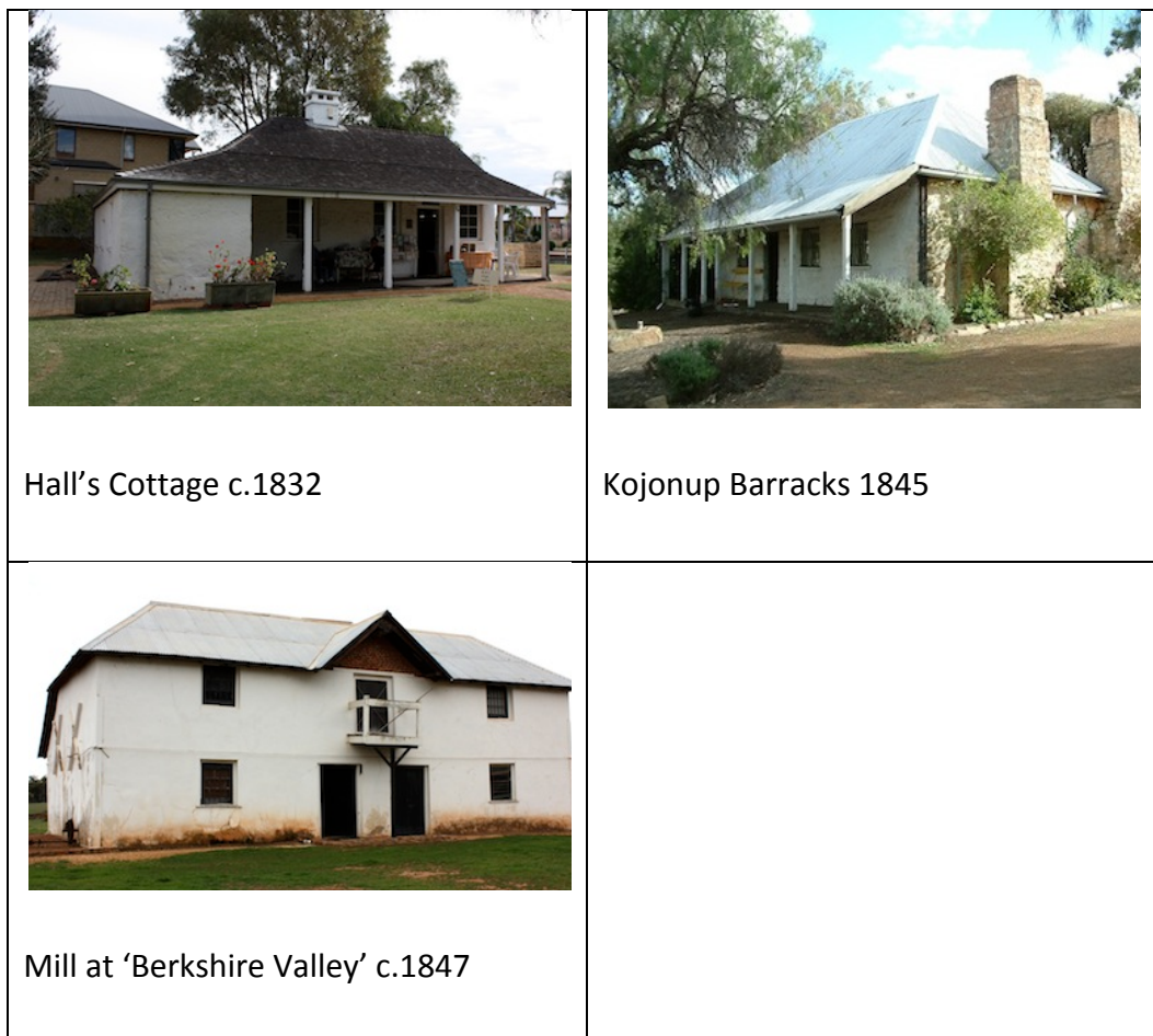
Figure 8.5 The three stone buildings in Group 1 (F Bush)
