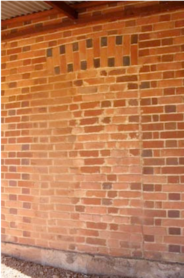
Figure 4 Bricked up opening on southern side; note brick arch
