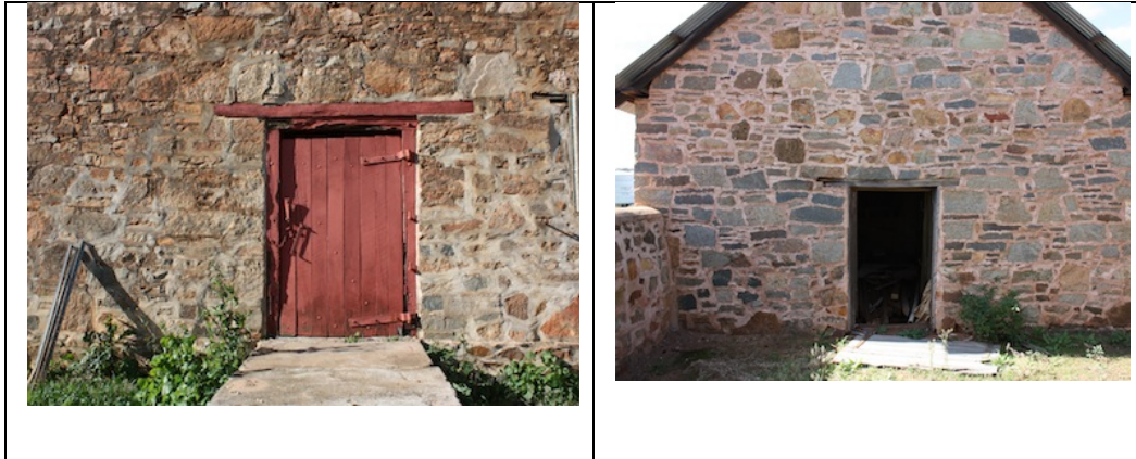
Figure 8.7 Two buildings at 'Walebing'. Wool Shed on the left and former Bulk Store on the right. Note the absence of an arch over the door openings. (F. Bush 29 June 2010)
