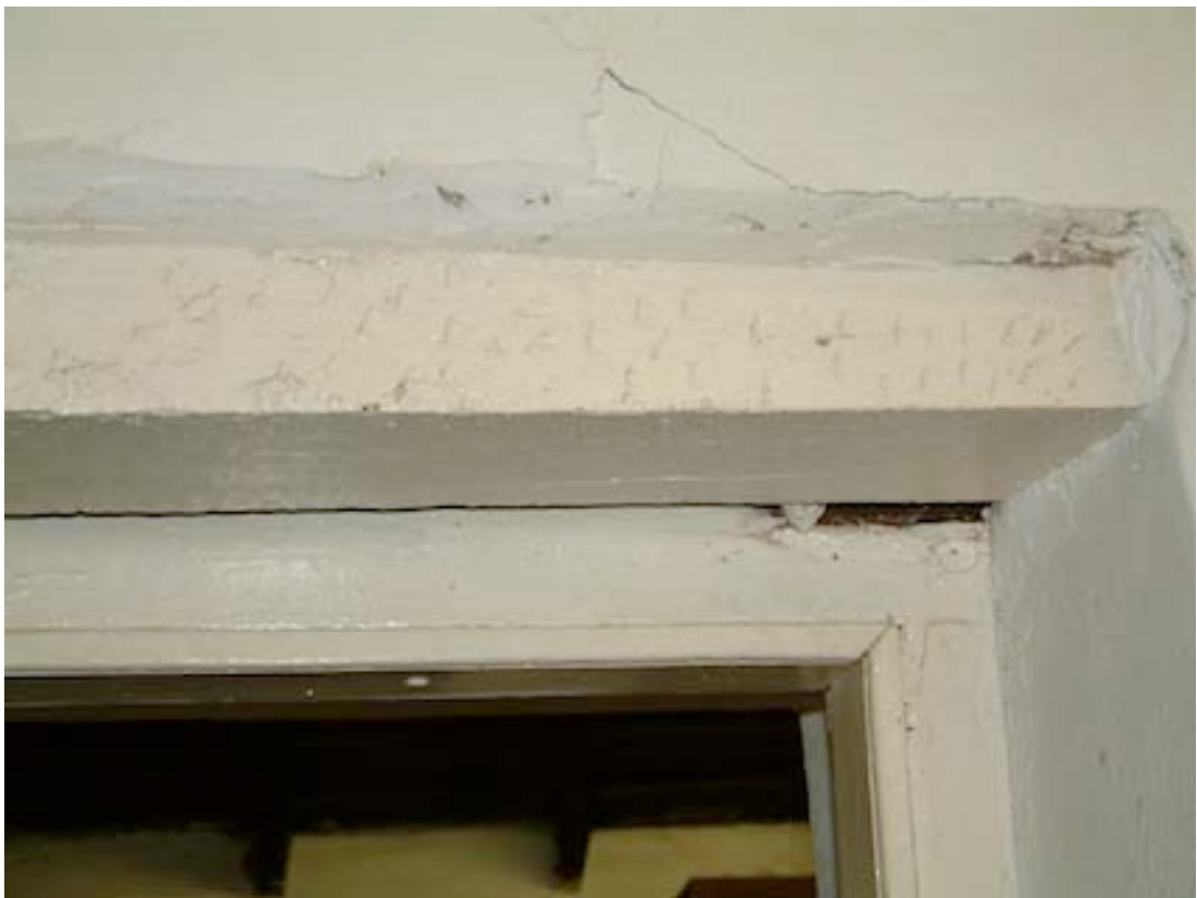
Figure 9 Detail of timber lintel above doorway and door frame. Note adze marks to lintel and the timber peg in the door frame denoting mortise and tenon joint.
