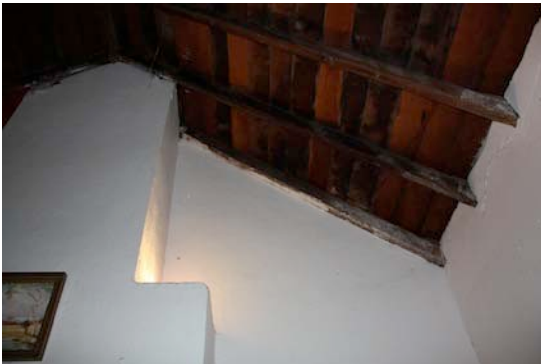
Figure 8 Room 1 looking east towards the chimney brest
