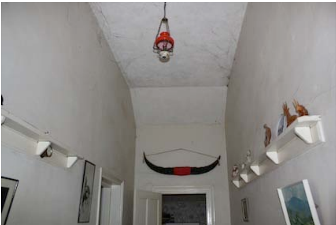
Figure 7 Interior view of Homestead. Central passage looking south. Note masard profile to ceiling at the end of the passage
