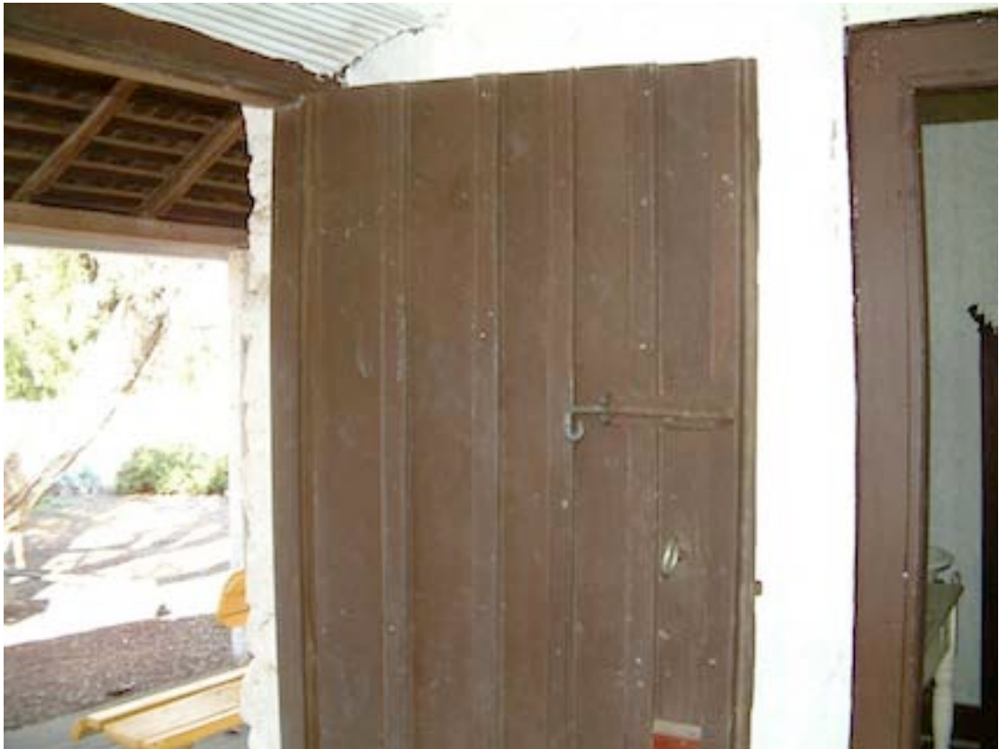
Figure 8 Detail of front door and doorframe of Room 2 on the right
