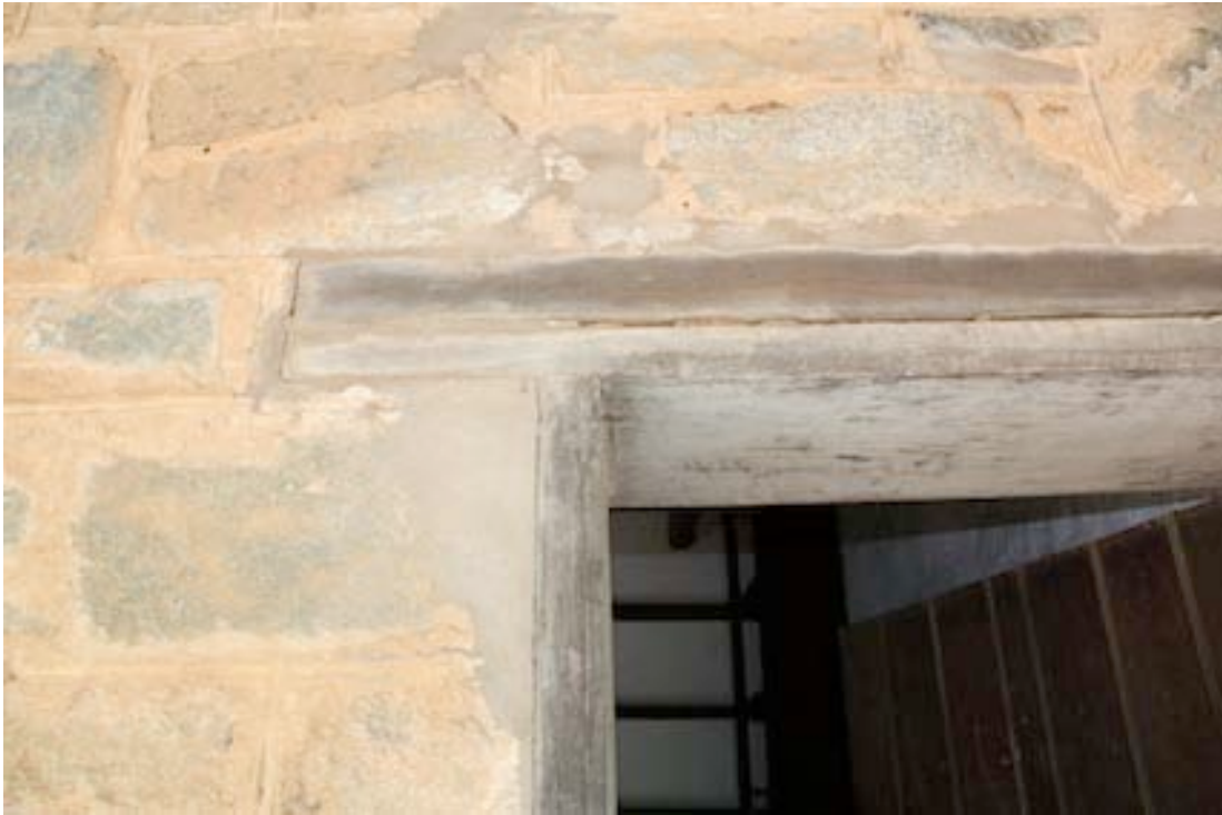
Figure 6 Detail of door frame to the Station Store Room.
