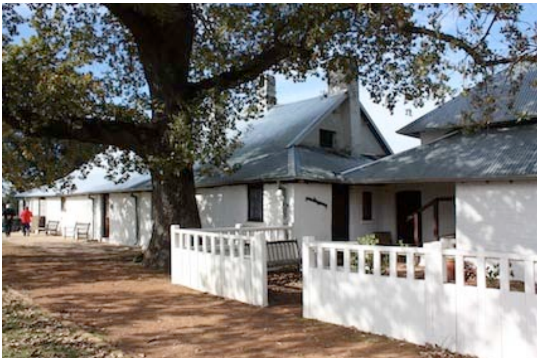
Figure 3 Northern side looking east. Detached store on right.
