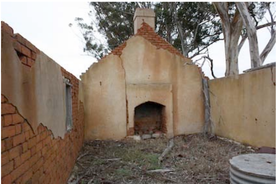
Figure 15 Looking south towards the fireplace
