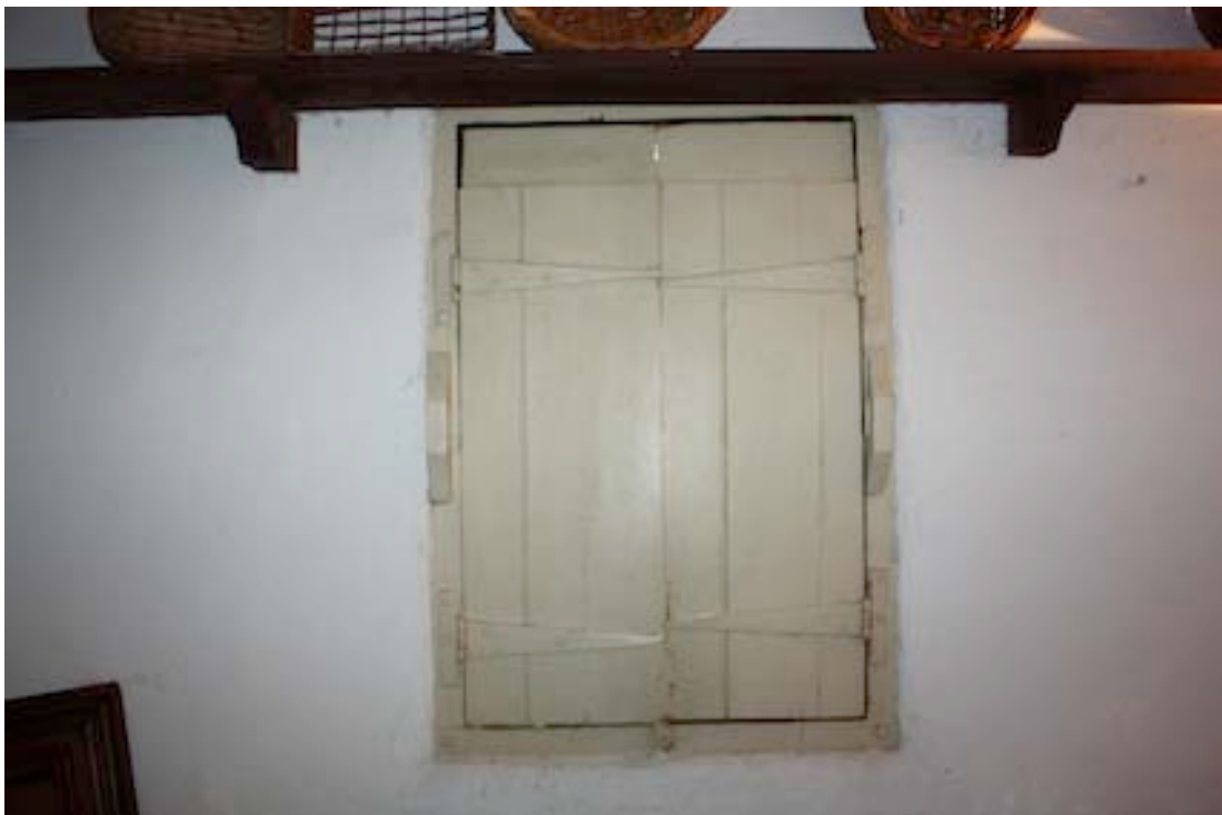
Figure 9 Interior view of east-west passage with timber shutters to one of the windows in the passage
