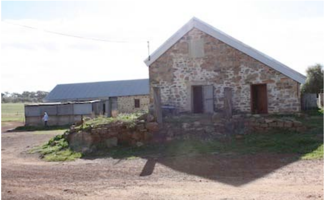
Figure 15 Southern side of building showing the former flour mill section. The Stables are visible in the distance on the left
