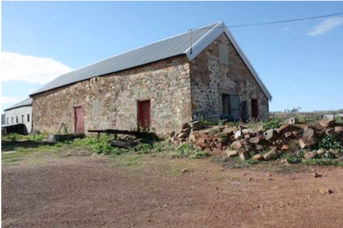
Figure 17 Western side of building. The stone wall is all that remains of the horse works area. The flour mill was powered by horses walking around a central shaft.
