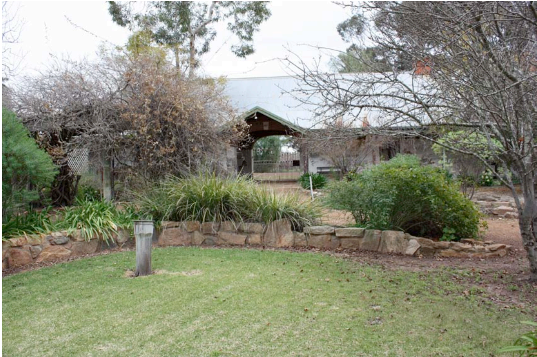
Figure 24 Gate House from the southern side which faces the central courtyard dividing the Gate House from the two houses.
