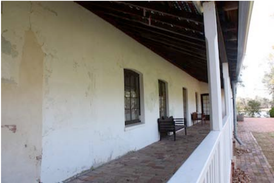
Figure 4 Verandah on the southern side of the house looking east
