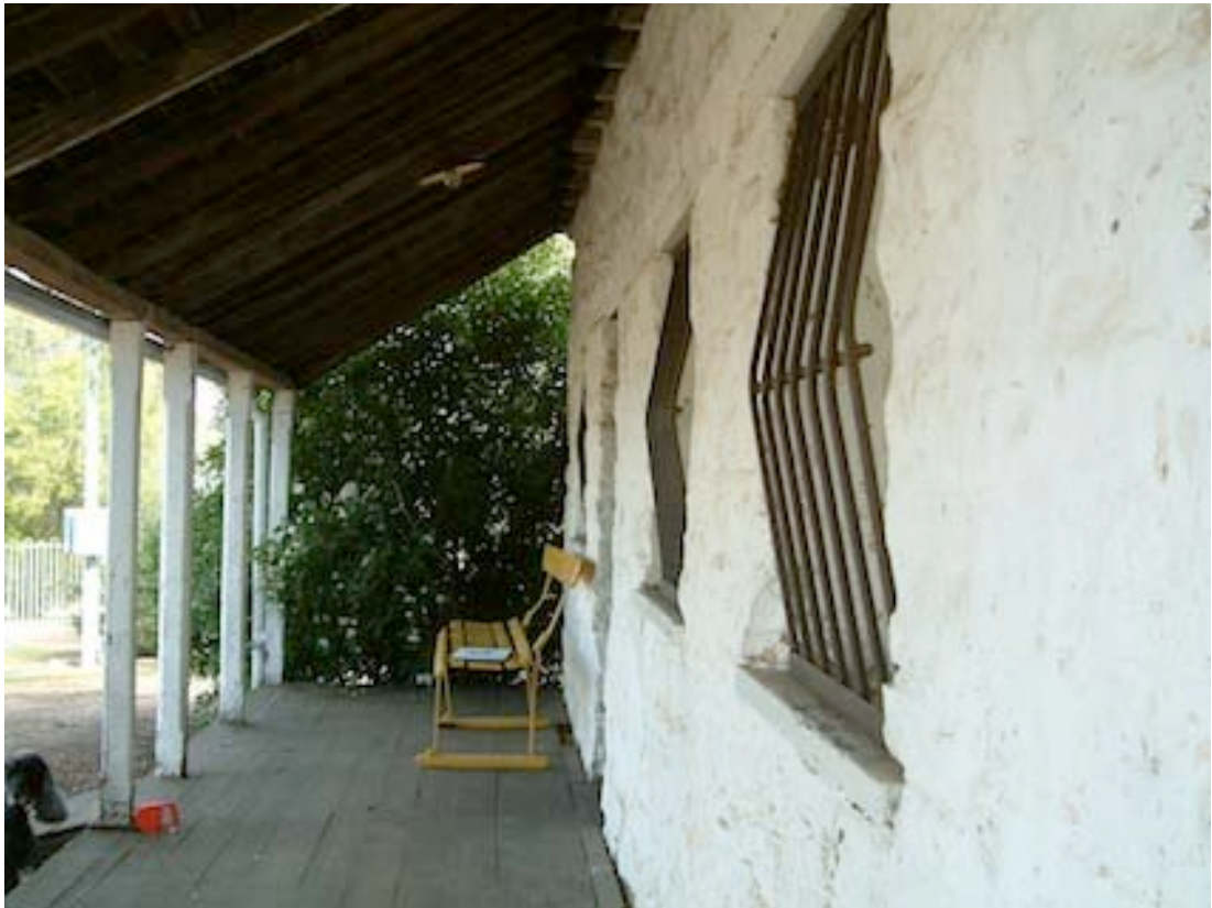
Figure 6 Front verandah. Note timber sills and lintels to windows
