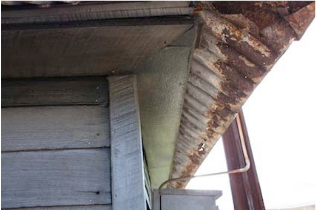
Figure 6 Detail of timber frame and weatherboard cladding
