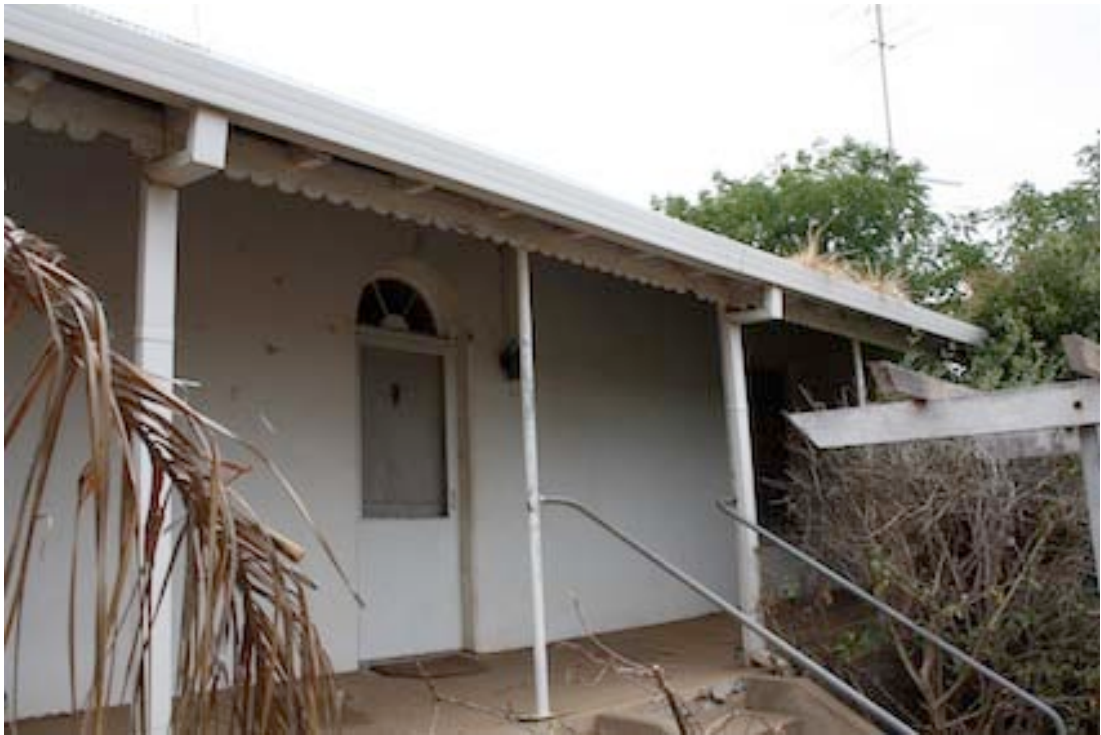
Figure 4 Southern side of Homestead. Note scalloped timber valance along verandah
