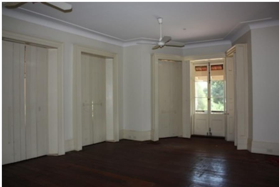
Figure 8.22 Timber shutters cover the interior side of the French doors in Bishop Hale's House (F. Bush 22 March 2010)
