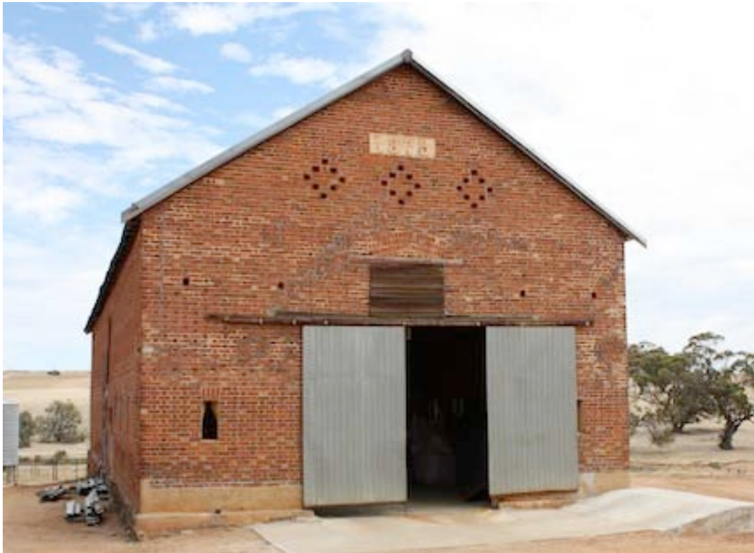
Figure 25 Eastern side of Stables bearing the plaque with the date of construction. Note round bricks which have been laid in a diamond pattern.
