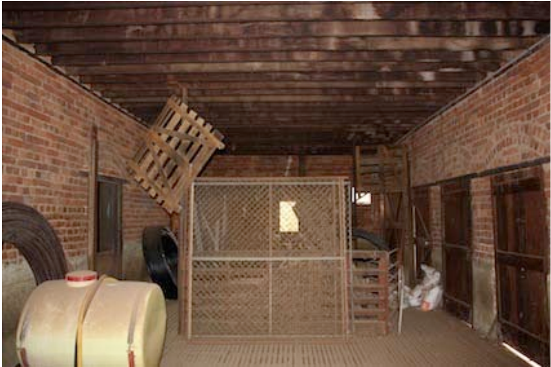
Figure 26 Eastern side of shearing shed with slatted timber floor and floor joists for loft area above.
