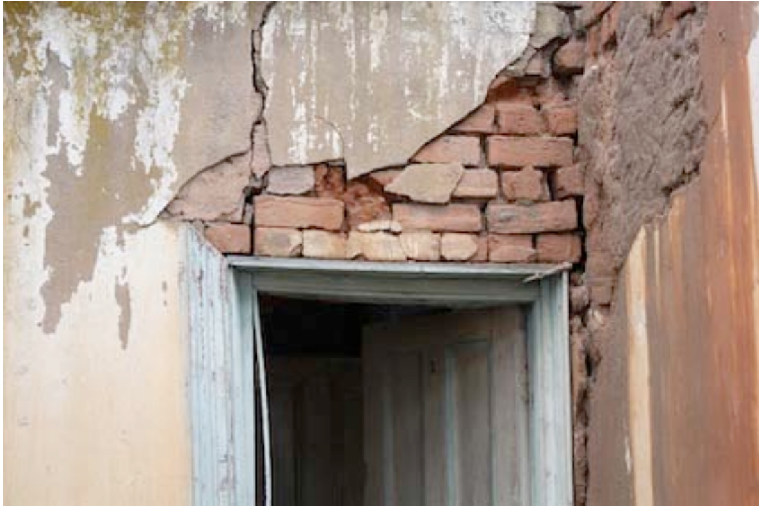
Figure 9 Southern door in Entertaining room that leads to Bedroom. Note the lack of a relieving arch and also the mud render that was applied to the wall before layers of lime wash and then paint.
