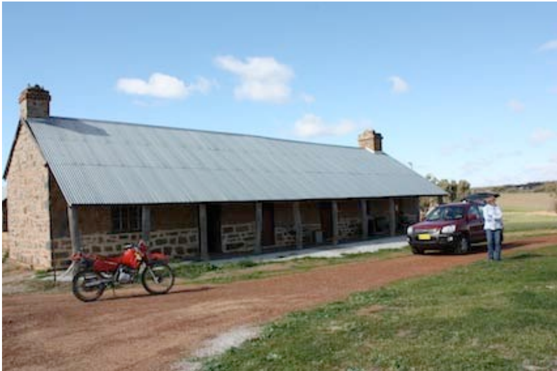
Figure 3 Western side of Kitchen Stores looking towards the south.
