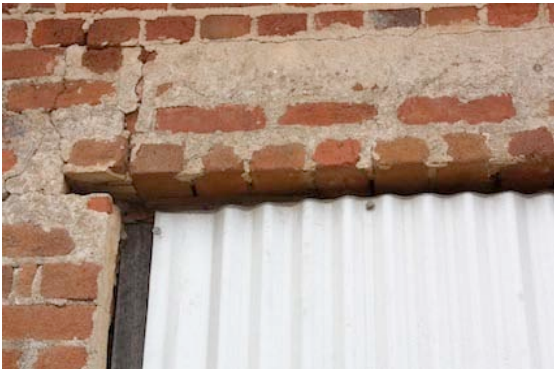
Figure 23 Detail of brick arch above doorway on the northern side
