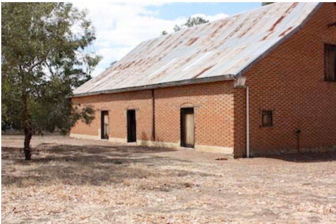
Figure 23 Western side of shearing shed.
