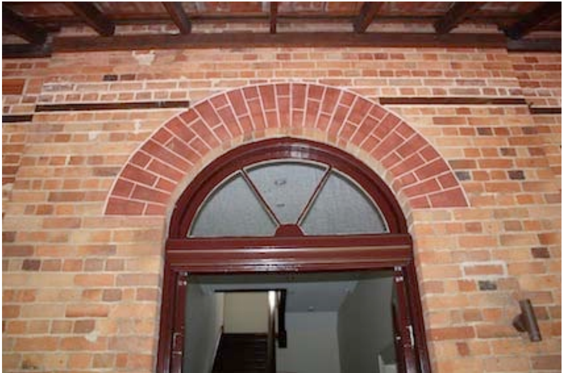
Figure 6 Detail of brick arch above main door on the north side.
