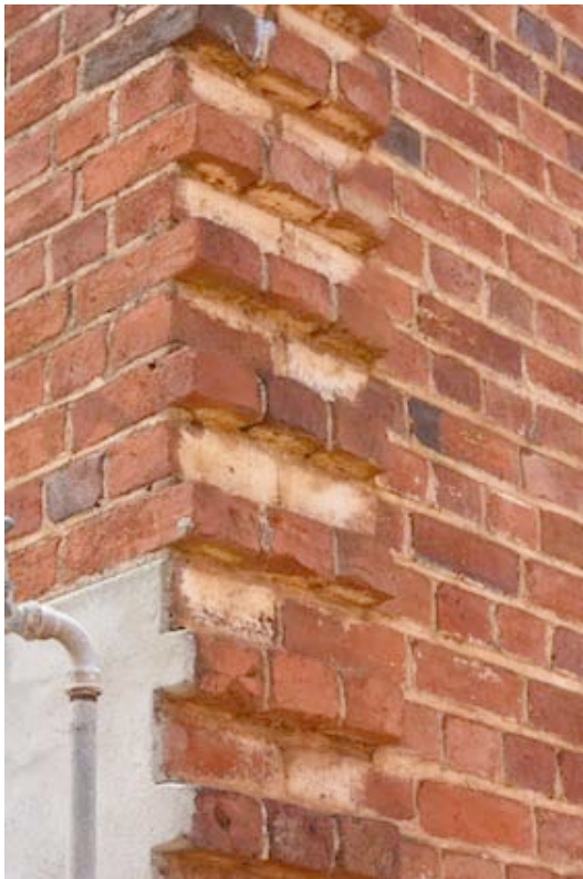
Figure 30 Detail of south-west corner of Stables showing toothed edge that may have been provided for a future extension
