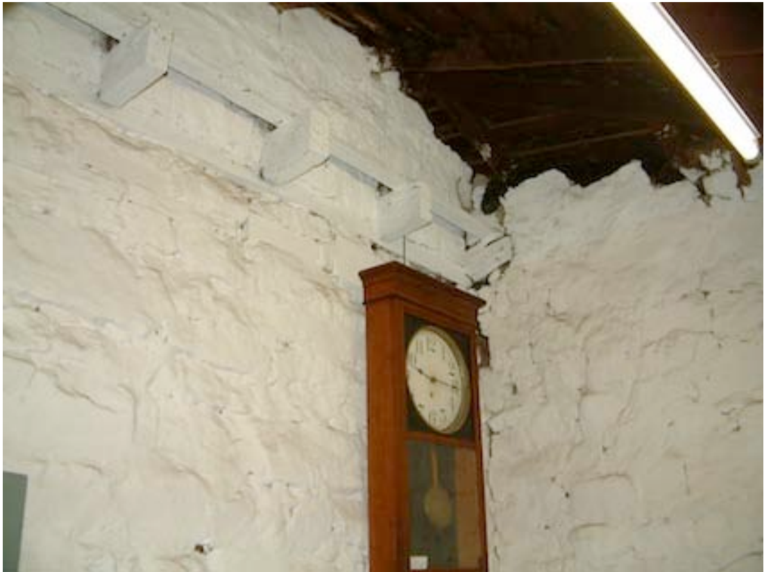
Figure 10 South-east corner of Room 3 showing edge of floor joists in attic
