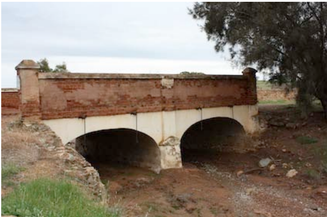
Figure 48 Bridge, viewed from the north.
