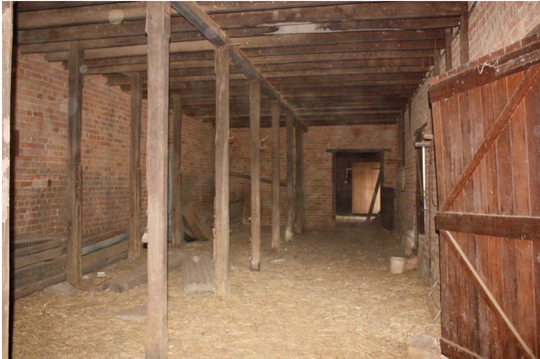
Figure 17 The remains of the timber stalls in the southern half of the stables. Note stop chamfering to vertical posts.
