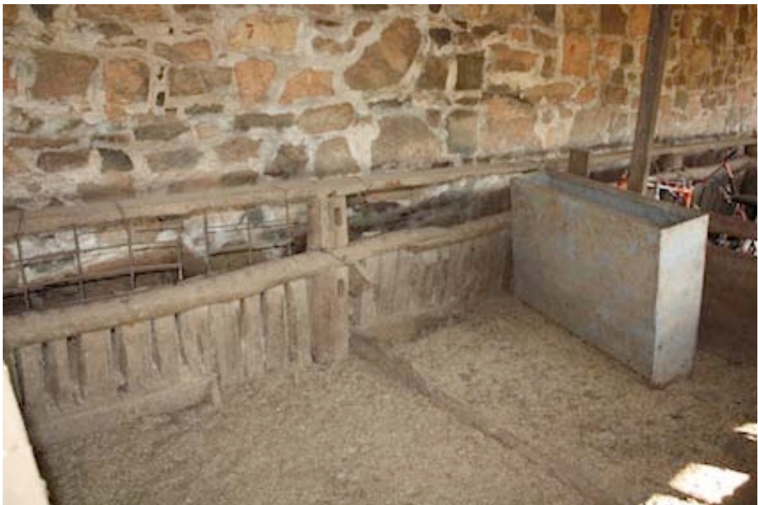
Figure 27 View of horse stall in northern section together with feeding trough
