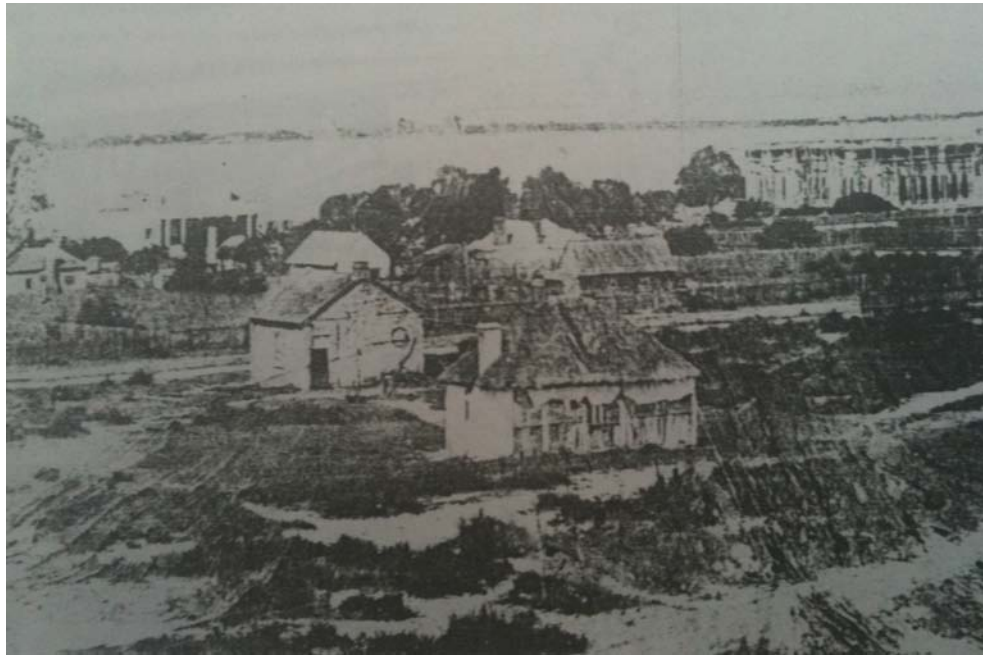
Figure 4.7 Perth in early 1860s. The cottage in the foreground appears to have been abandoned as the plaster covering is falling off. (J.S. Batty Library 26345P, reproduced with permission of Mrs Croft)
