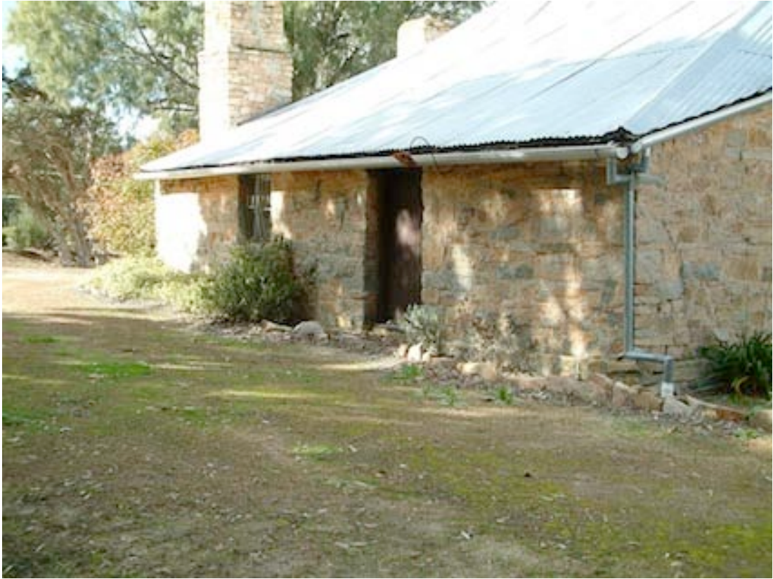
Figure 4 Rear of Barracks building
