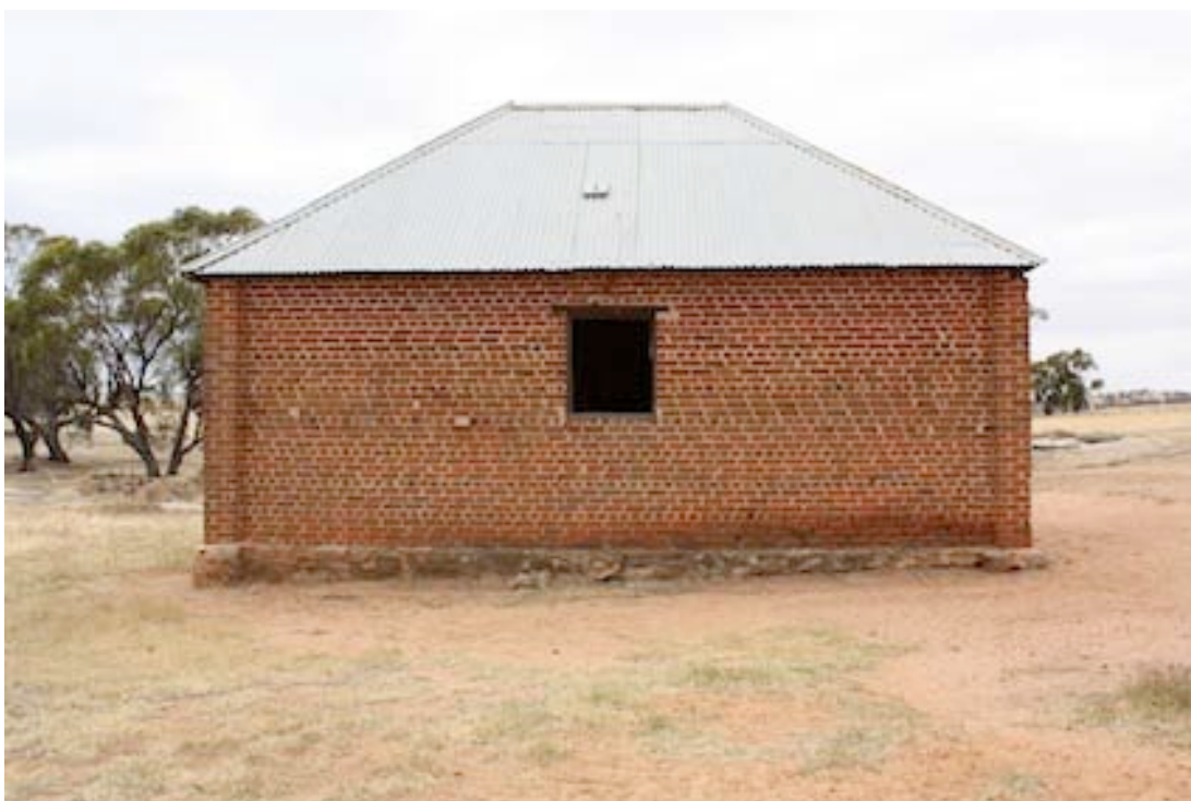
Figure 21 Southern side of Workers' Quarters
