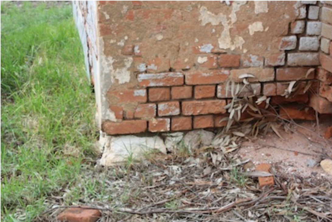
Figure 8.4 Homestead at 'Martinup', note the stone foundation which is little thicker than the brick walls (F. Bush 10 February 2011)
