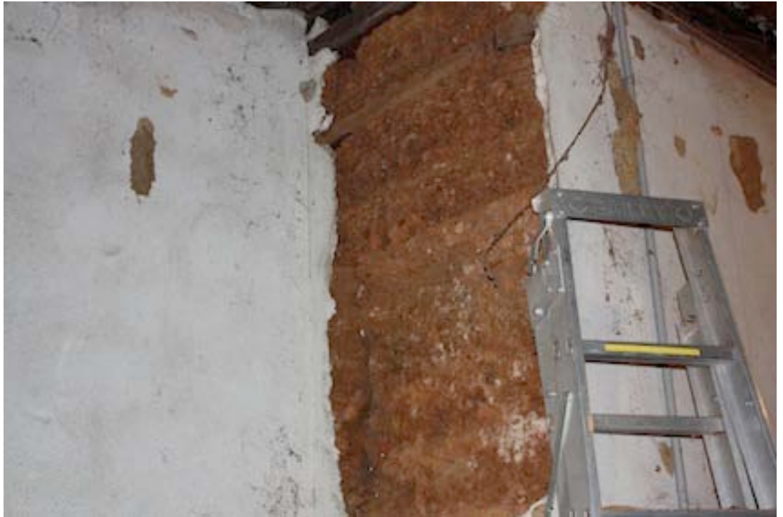
Figure 8 Detail of south-east corner of building showing rammed earth construction
