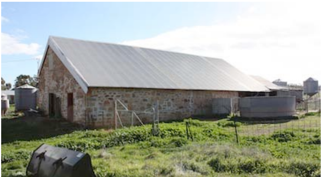
Figure 16 Eastern side of building showing single storey section with the new shearing shed at the rear
