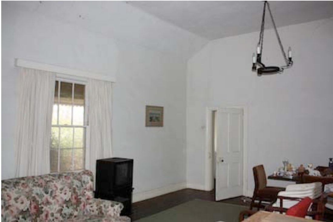
Figure 8 Interior view of lounge room looking north-east. Note mansard shaped ceiling
