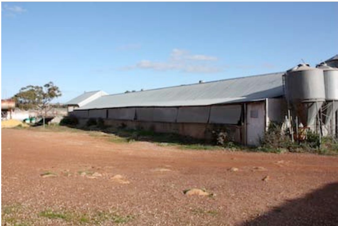
Figure 32 Eastern side of Cart Shed showing new concrete walls to c.1 metre high.
