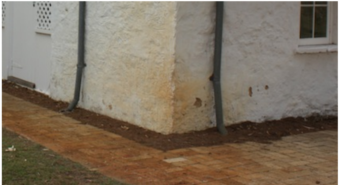
Figure 8.3 Hall's Cottage, there was no evidence of a foundation beneath the gravel (F. Bush 15 May 2011)
