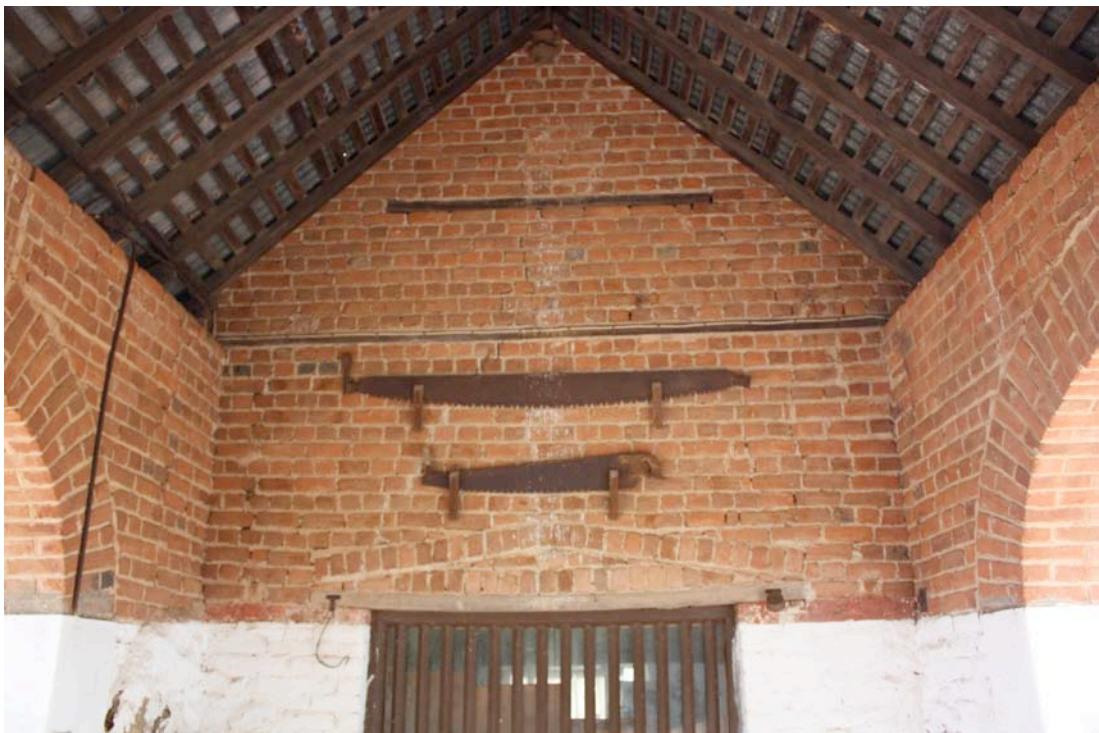
Figure 27 Entry area looking west towards door that leads to dairy. Note the brickwork that has been laid using English bond
