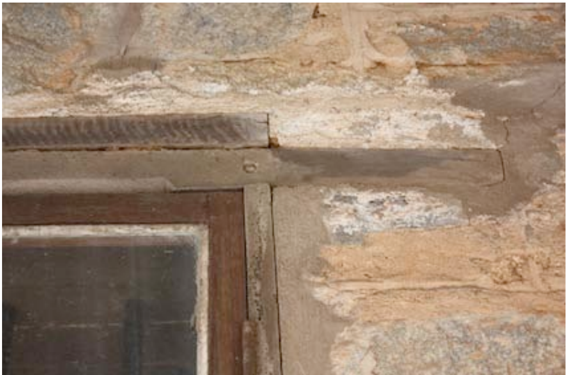
Figure 5 Detail of window frame in the Station Store room.
