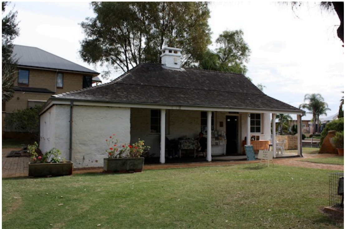
Figure 4.6 Hall's Cottage, front elevation (F. Bush 15 May 2011)
