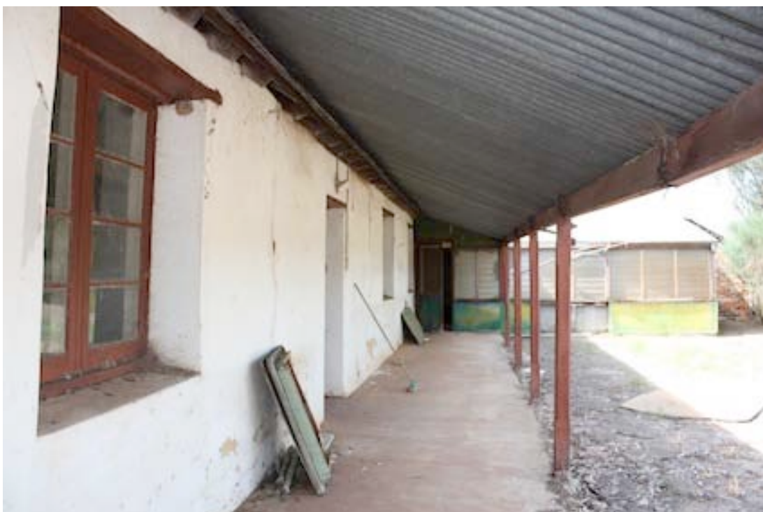
Figure 5 View of western verandah (rear) looking north
