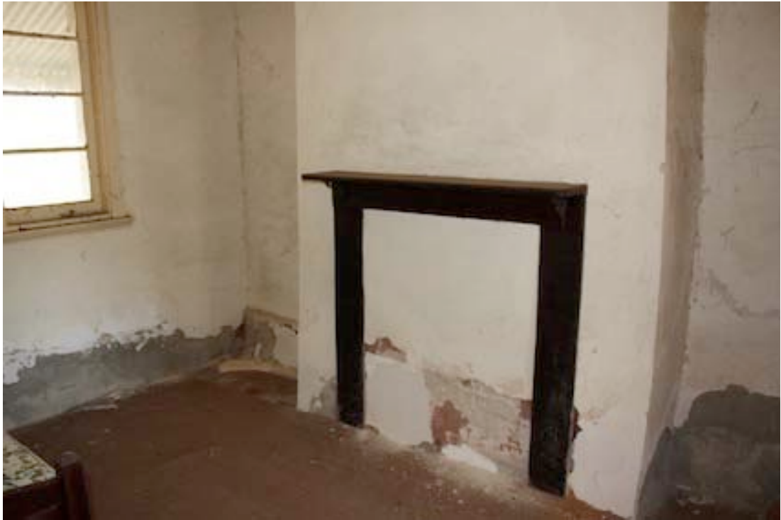
Figure 8 Room 11 showing blocked up fireplace and timber mantelpiece
