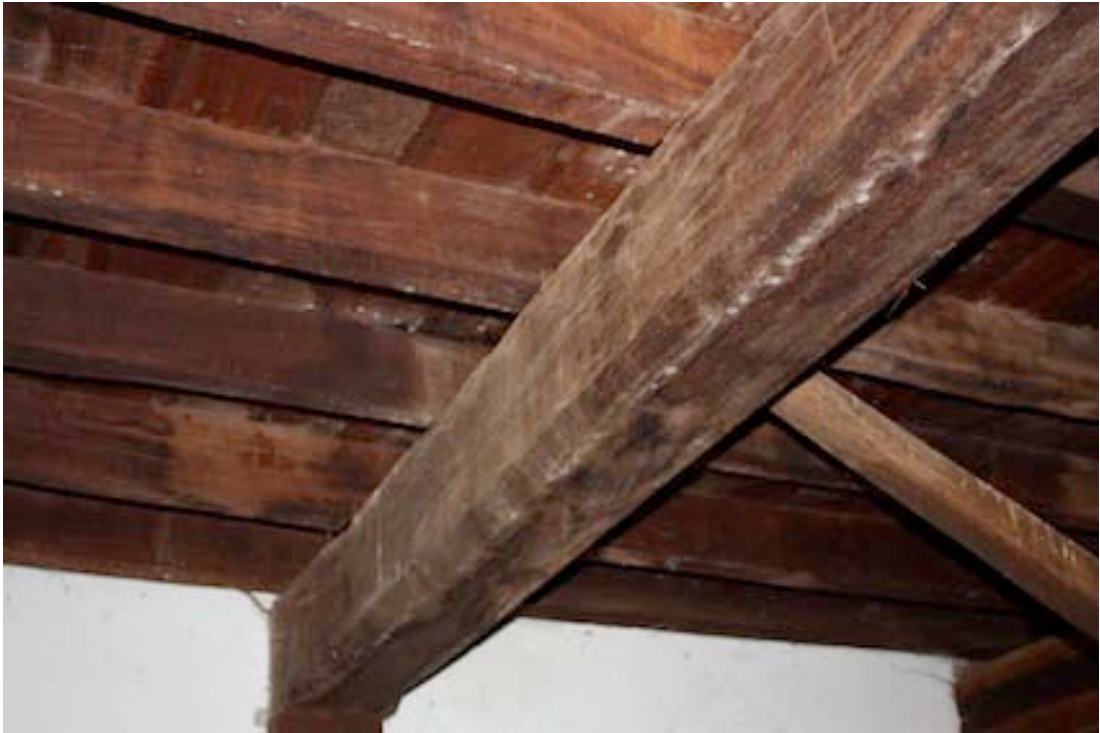
Figure 9 Detail of adzed timber bearer on ground floor.
