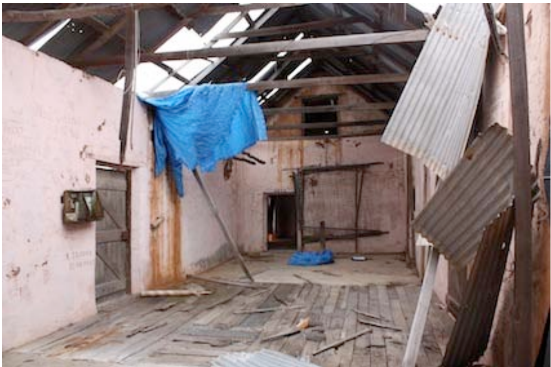
Figure 25 Interior view of Wool Barn looking south towards Shearing Shed
