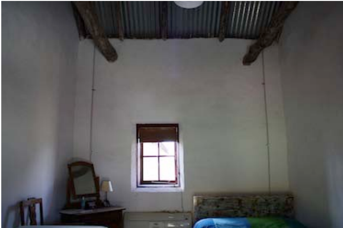
Figure 8 Interior view of the Cook's Room, looking east
