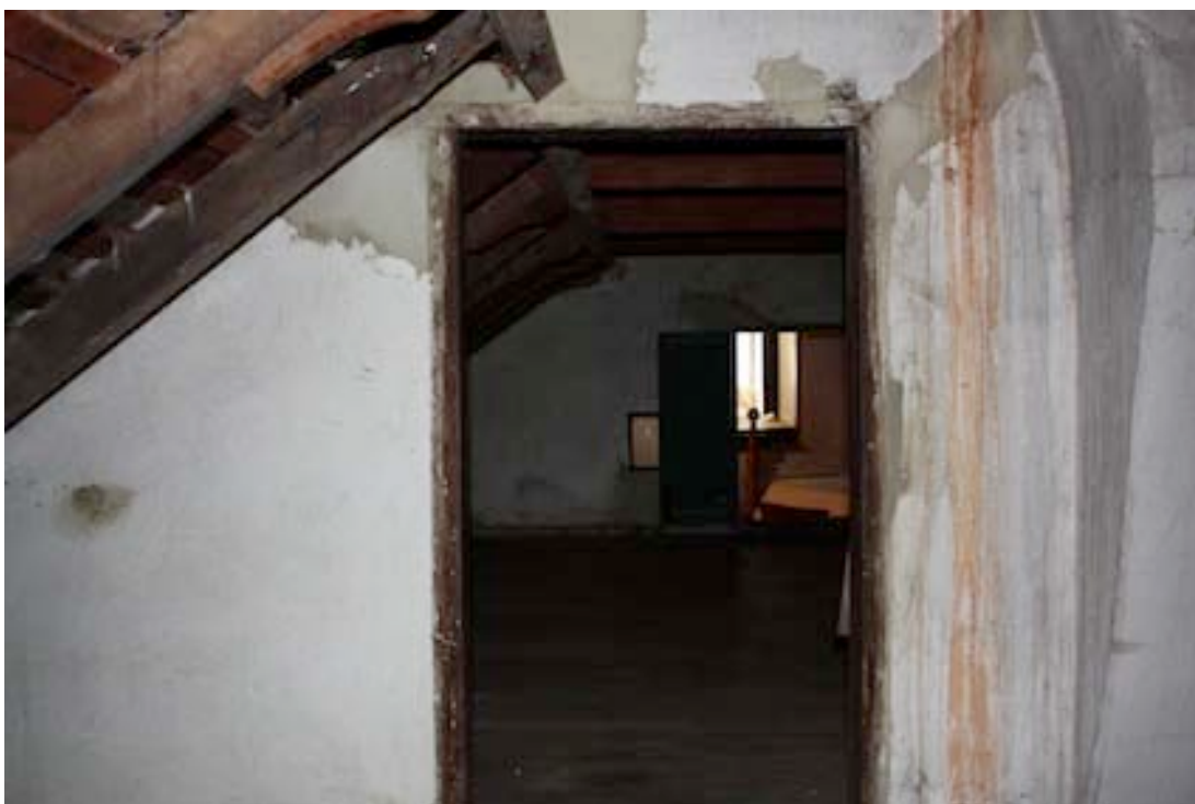
Figure 7 Interior view of attic area. Room 23 looking east towards Rooms 24, 25 and 26
