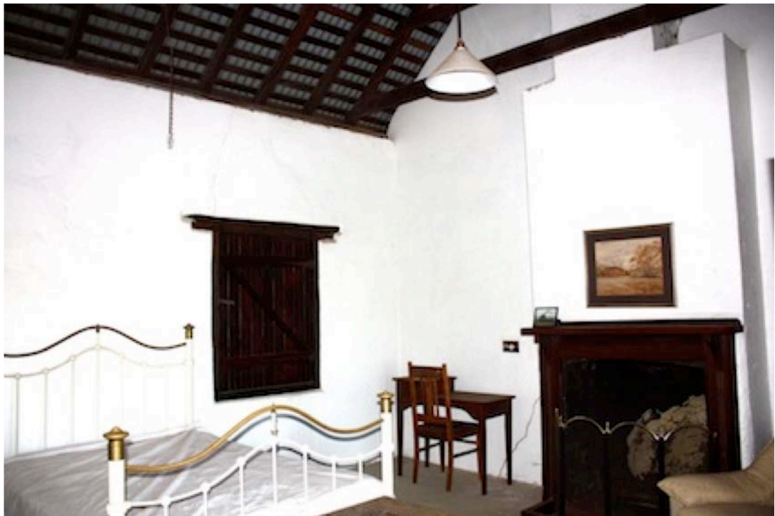
Figure 8 Interior view of Room 2 looking west.
