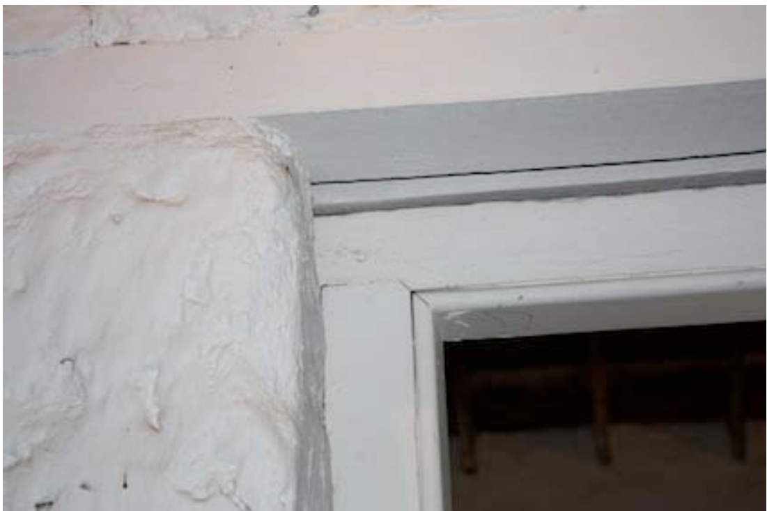
Figure 11 Detail of door frame
