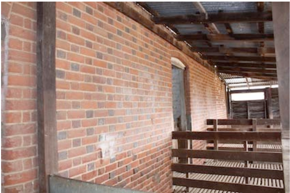
Figure 14 Northern side of the Shearing Shed
