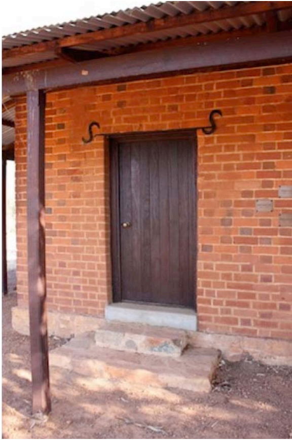
Figure 5 New opening in north wall.
