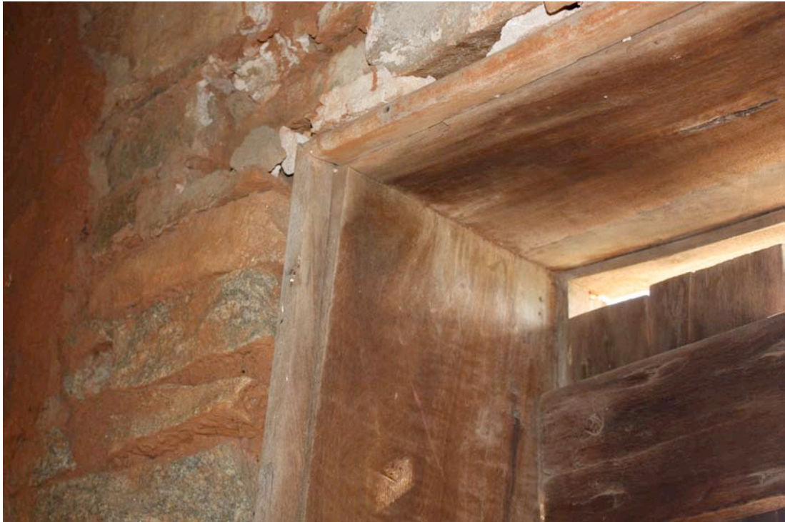
Figure 12 Interior side of window frame. Note the mud mortar and evidence on the stones of a lime wash coating
