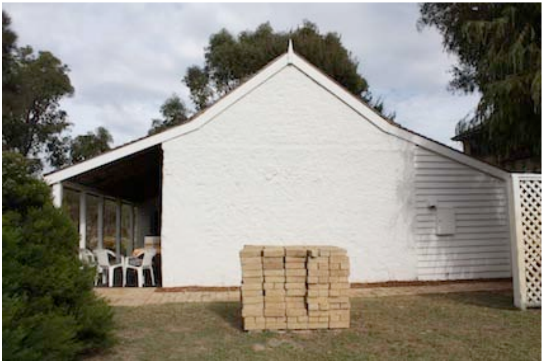
Figure 3 View of Cottage from south-west side
