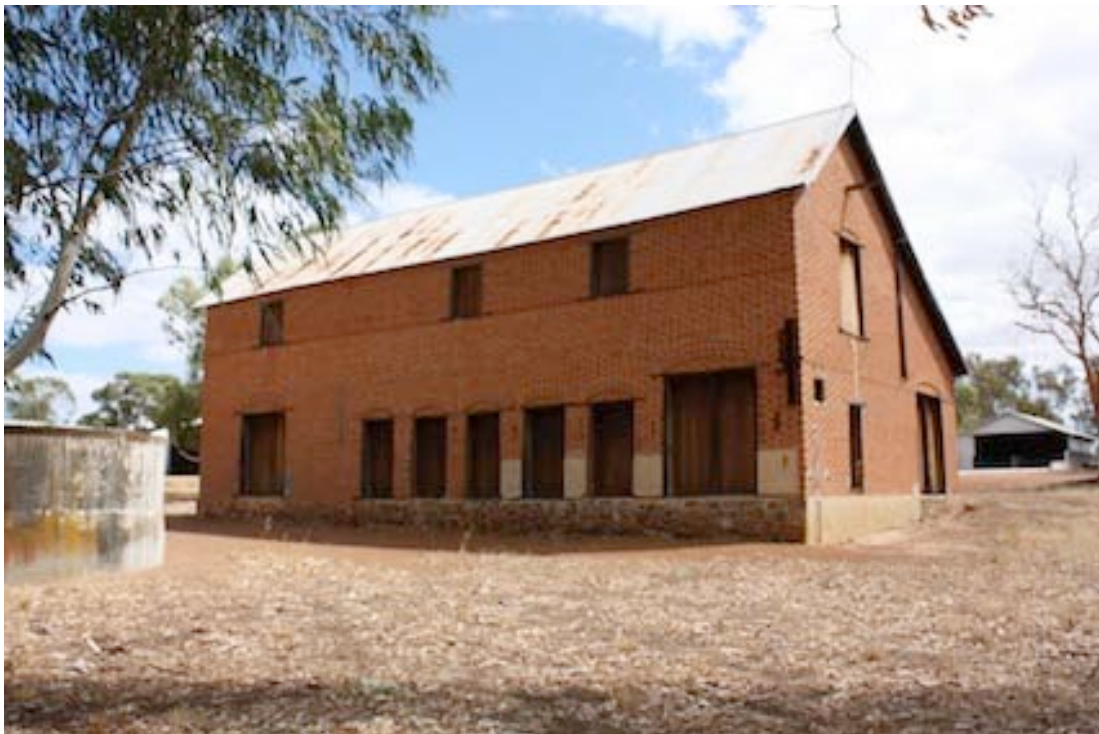
Figure 22 Eastern side of shearing shed.
