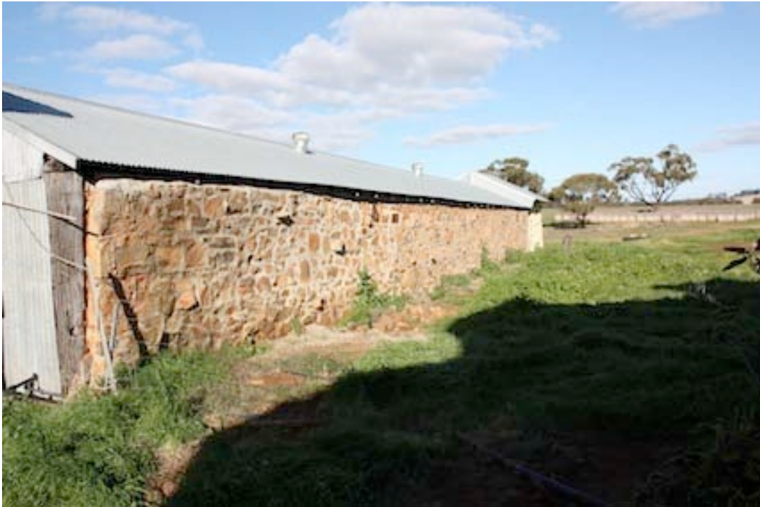
Figure 33 Western side of Cart Shed
