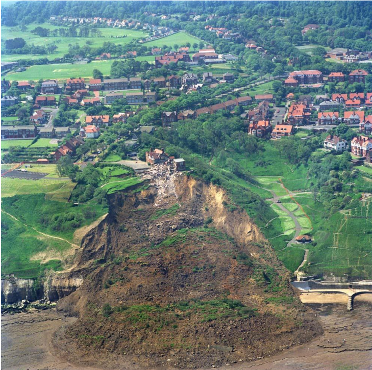
Fig. 3 The Holbeck Hall Hotel landslide, Scarborough, North Yorkshire
