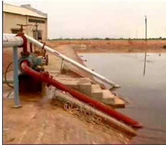
Figure 2.6 The external heat exchanger at Bhuj solar pond
