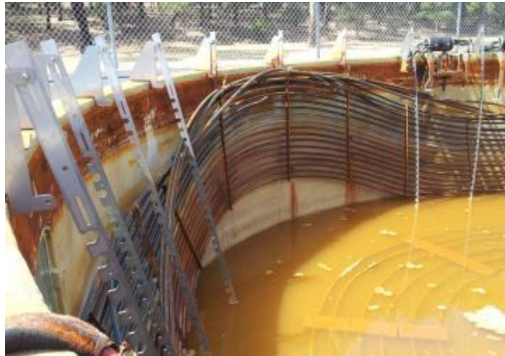
Figure 3.15 Installation of new supports
