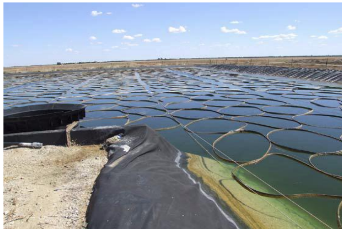
Figure 2.4 Wave suppression by floating ring at Pyramid Hill solar pond
