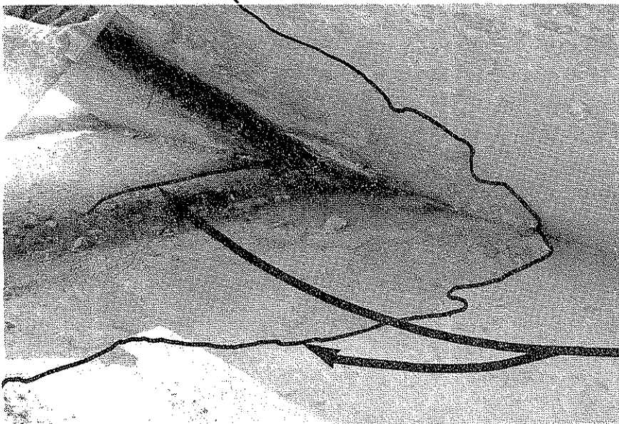
Joint #8 Leave Panel: Note Joint Deterioration. Grout and subbase material adhering to underside of panel.
