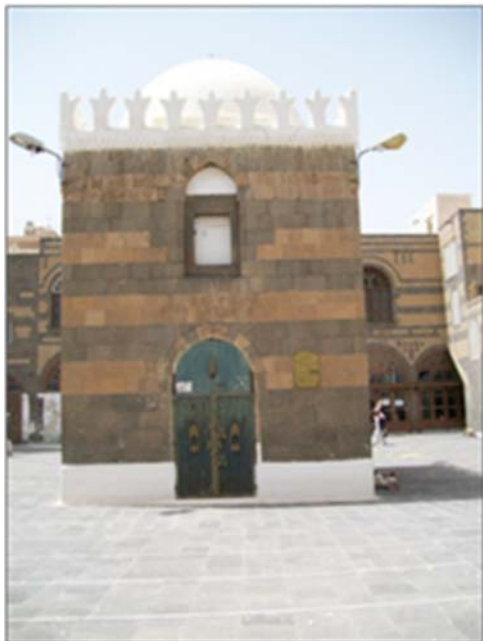
Figure 5. Sana'a, general view of Dome of Oil, Photo: Enab, 2011
