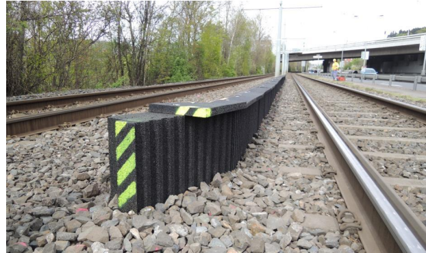
FIGURE 10. Municipal Noise-absorbing Screen after modification.
