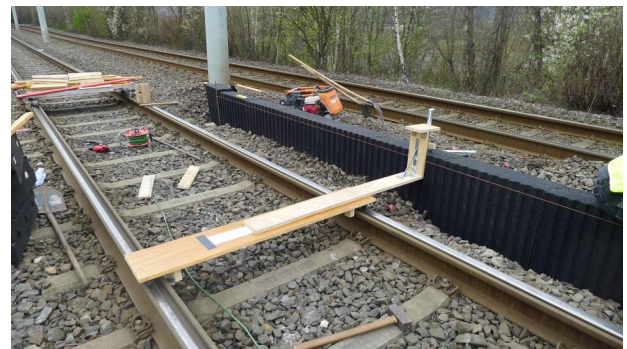
FIGURE 7. Checking the screen distance and height from the rail axis and TR.
