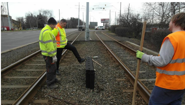
FIGURE 3. Mounting of MNAS prototypes – Vandal resistance test.
