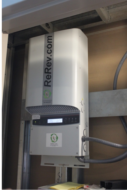
Figure 8: Wind Inverter for AC grid intertie
