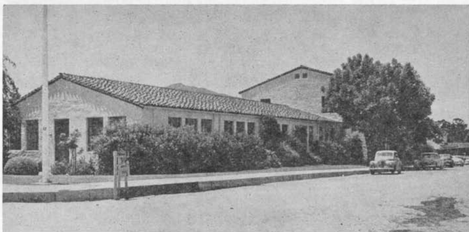
Air Conditioning Building
