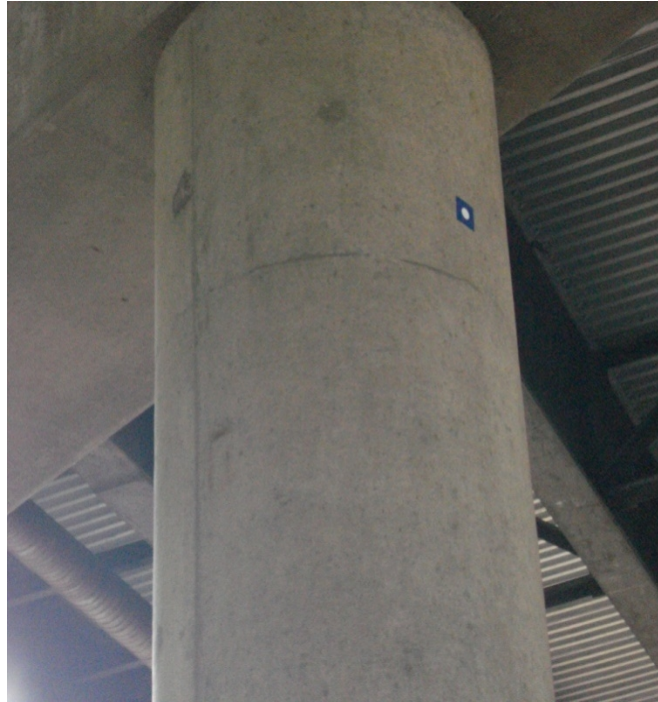
Figure 4.3: An installed target on a column
