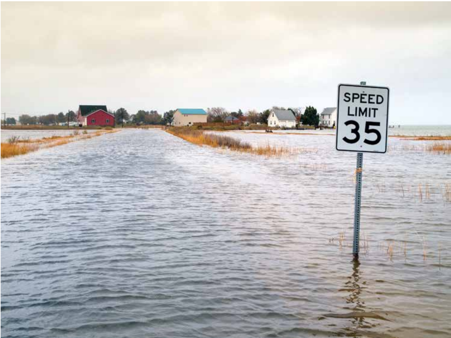
A road on Hoopers Island that floods regularly during extreme tidal events, Dorchester County MD, 2009. David Harp/ChesapeakePhotos.Com.
