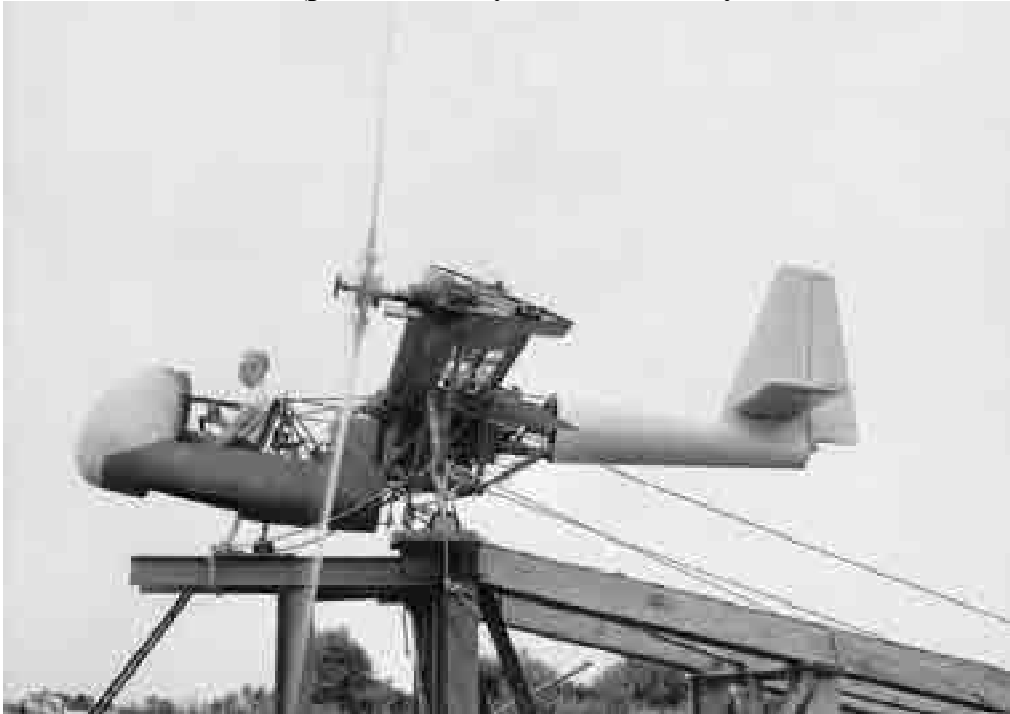
Fig. 2-118. Mario Guerrieri's Model 1, shown here on its ground test rig, was virtually destroyed in November 1950 because of ground resonance (photo courtesy of Howard Levy and Mike Hirschberg).
