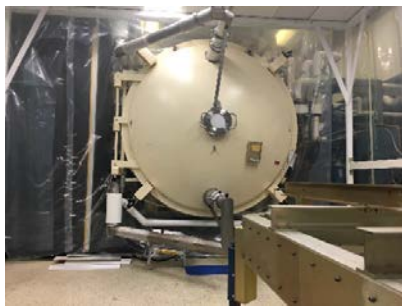
Figure 5. OCL Chamber in building 5
