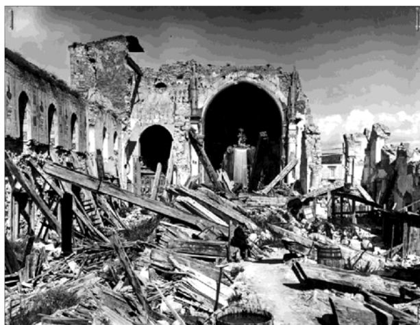
Fig. 2. Messina Cathedral destroyed in the earthquake of 1908
