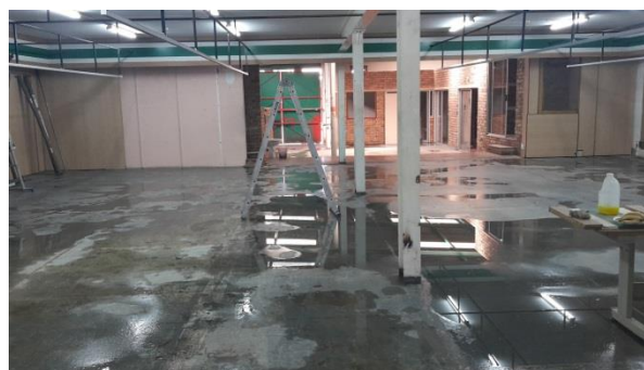
Photo 3: Renovations for EDC / Textile Hub in progress
