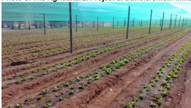
Photo 7: Shade-net structure for the production of vegetables (1x hectare)
