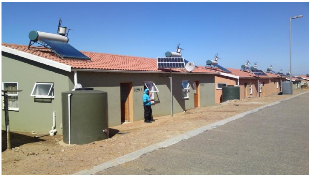
Fig. 1.3. Houses in the Kleinmond Housing Scheme site fitted with 2000 L DRWH tanks, solar geysers and photo-voltaic panels (Adopted from WRC Project K5/2124/3 Report, 2014).
