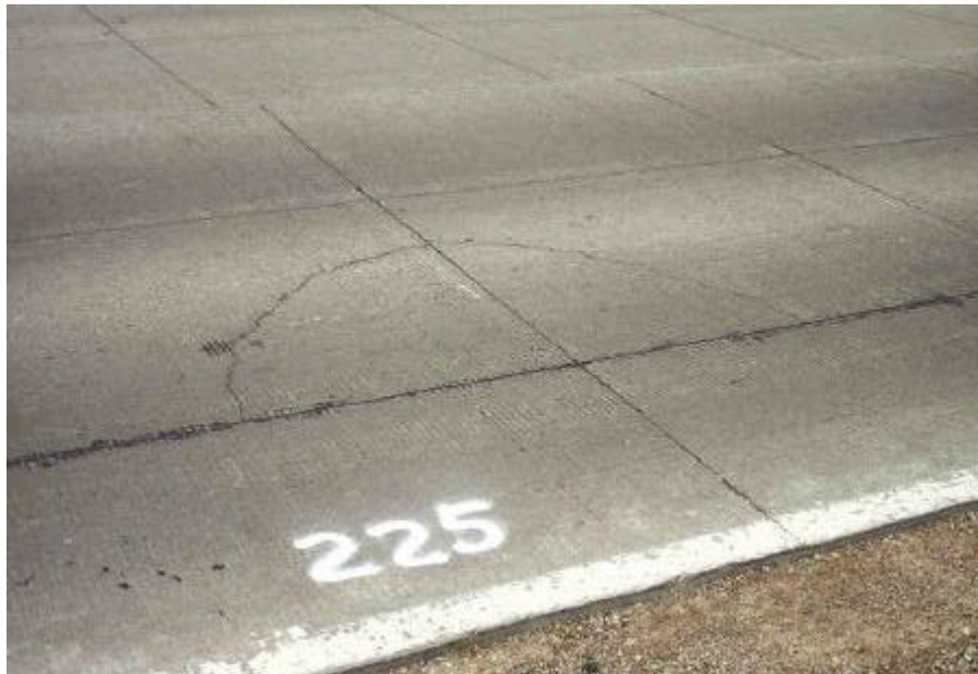
Figure 2.16 Panel Corner Breaks in Tuscola Project (Winkelman 2002)
