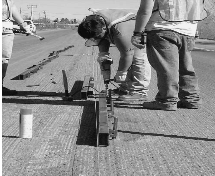
Figure 2.8 Use of Fixed Forms (Rasmussen and Rozycki 2004)
