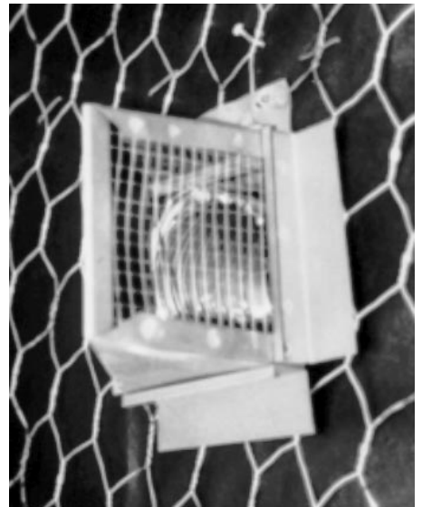
Fig. 26. A side wall exhaust vent with 1/4-inch hardware cloth.
