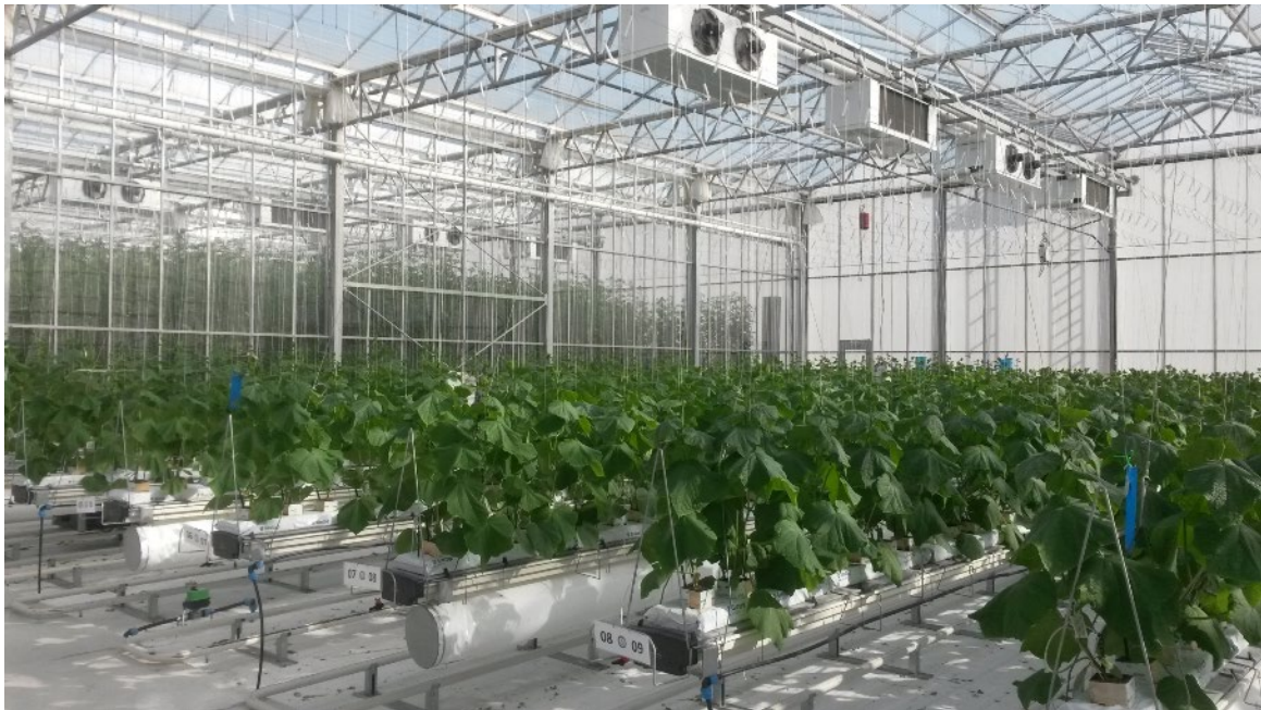
Figure 1. Picture of the greenhouse compartment showing the coolers placed above the canopy below the cover and thermal screen, the growing gutters, the air ducts for dehumidification and the heating transport system
