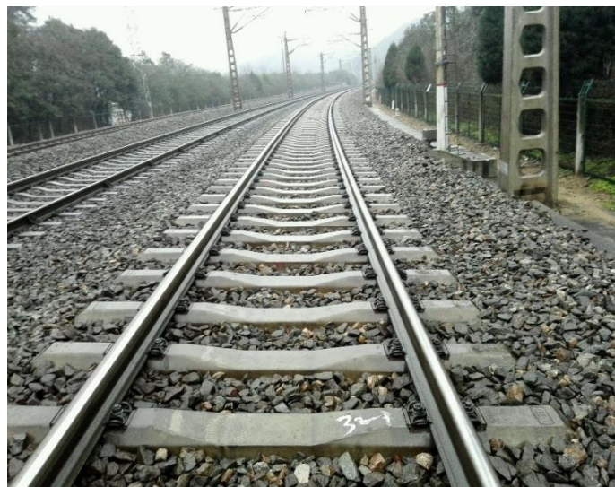
Fig. 1. Prestressed concrete sleepers in ballasted railway track
