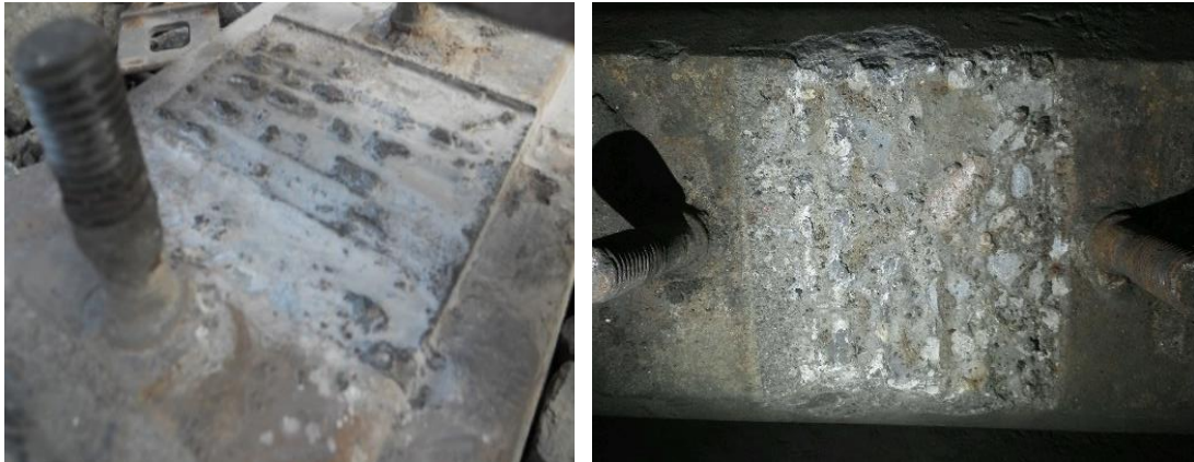
Fig. 2. Typical RSA of prestressed concrete sleeper
