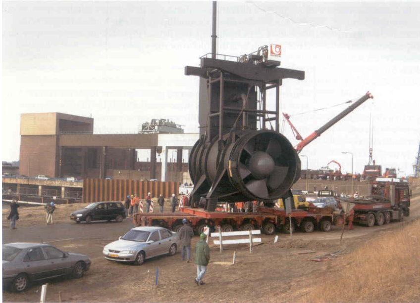
Figure 4.1 Picture from RWS Netwerk June 2004. One of the two additional pumps for the discharge station IJmuiden. This is at the moment the discharge station with the largest discharge capacity in Europe.
