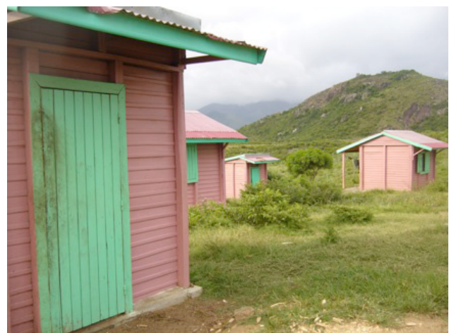
FIGURE 3. Resettlement houses built by Rio Tinto/QMM (photo taken by Seagle, March 2009).
