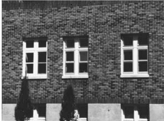
Figure 1: Near View of Old Building Low in Visual Richness and With No Visible Entrance
