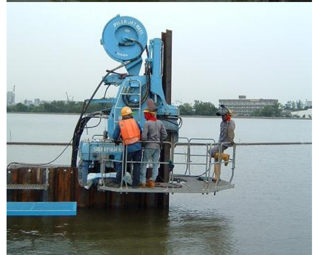
Fig. 21: Non-Staging Piling Work using GRB System
