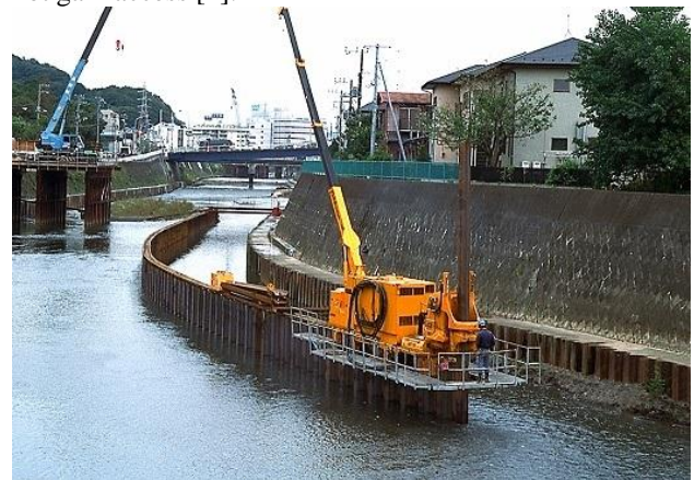
Fig. 8: Non-staging Press-in Piling in Marine Condition
