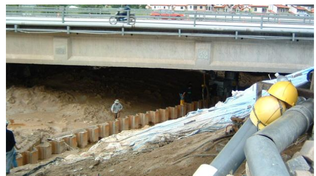
Fig. 14: Sheet Pile Installation Work using Clear Piler
