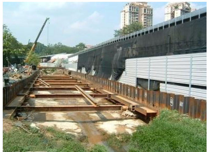
Fig. 18: Strutting Work for Construction of New Drain
