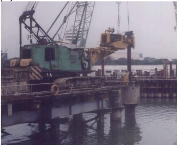
Fig. 2: Challenges by using Conventional Piling Method
