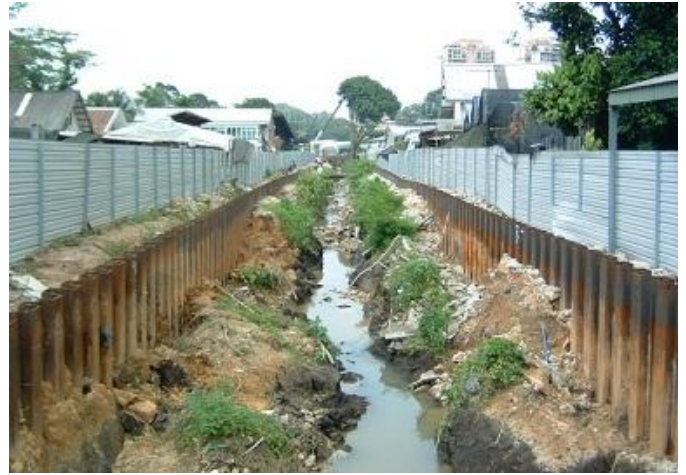
Fig. 17: After Installation of Sheet Piles at Both Sides
