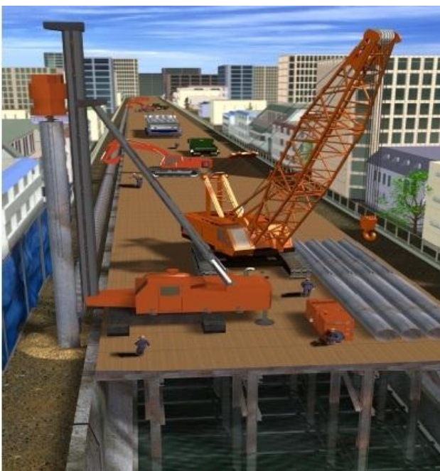
Fig. 3: Requirement of Temporary Deck for Piling Operation in Soft Soil & Marine Conditions
