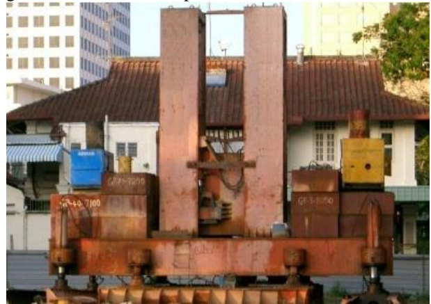
Fig. 4: Jack-in Piling based on Counter Weight System
