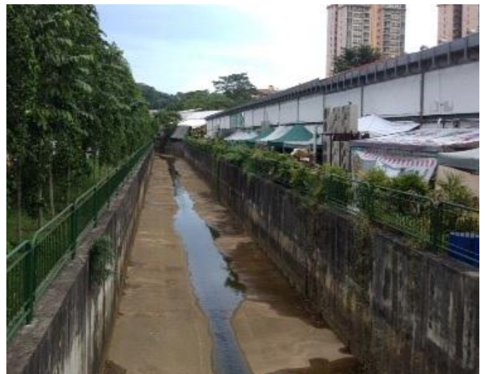
Fig. 19: Completion of New Drain (after 3 years)
