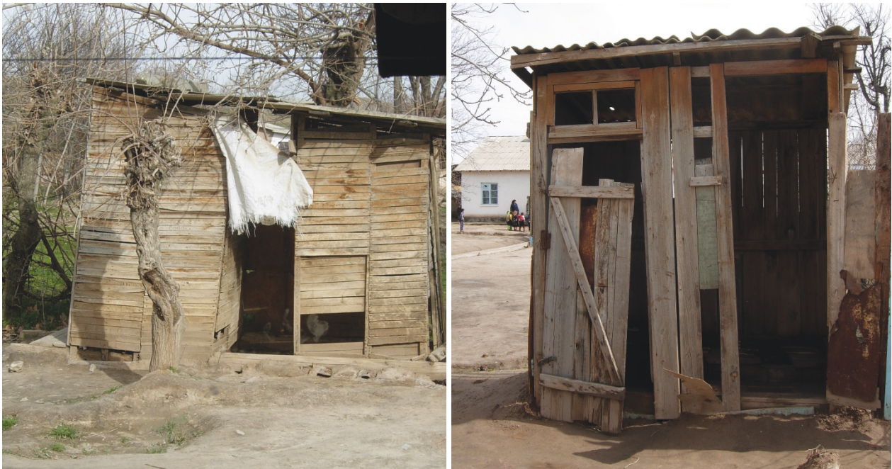
Figure 2 School latrines in two primary schools in western Tajikistan, early 2009.
