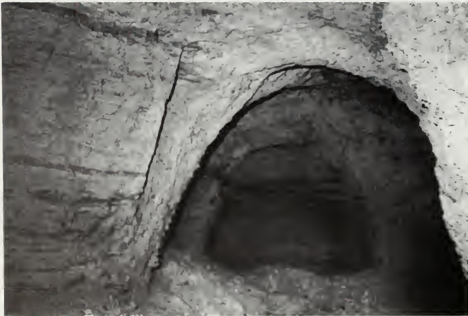
Figure 21 Inactive underground silica mine northeast of Olive Branch (site 119, fig. 10). The haulage way is about 5 meters (16 ft) wide. Figure 20 shows the location of the photo (taken by J. M. Dexter).
