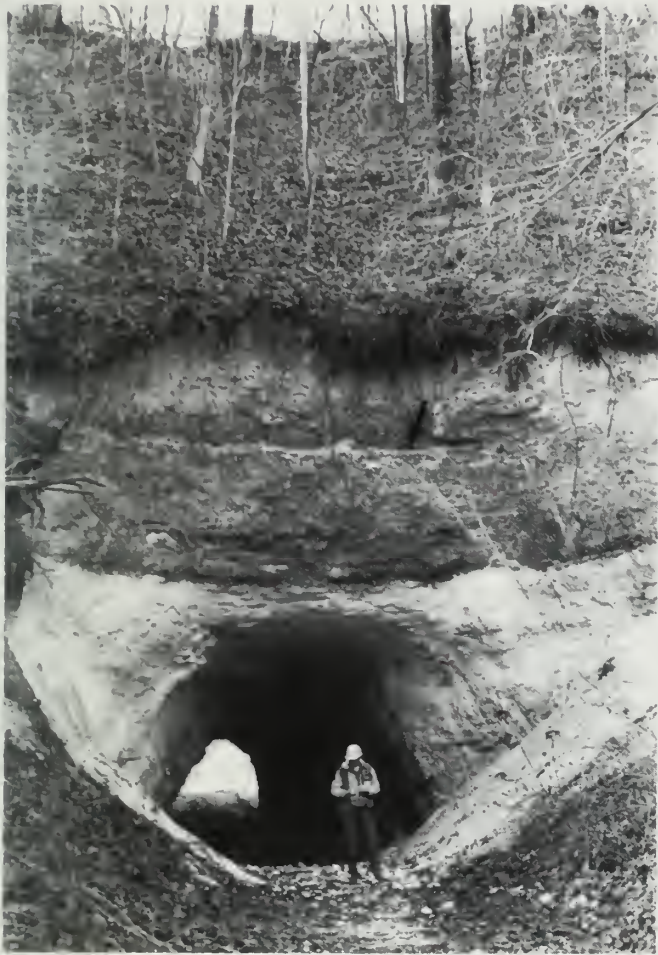
Figure 39 Portal of an inactive silica mine at site 100 (appendix A and figure 5). The photo shows the abrupt change in the amount of discoloration caused by iron oxide. Note the thin unstained bed, as indicated by the arrow, in the upper part of exposure. Photo By J. M. Masters, ISGS.
