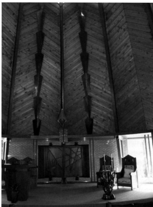
FIG. 5. Interior of Temple Emanu-El. Photo by the author.
